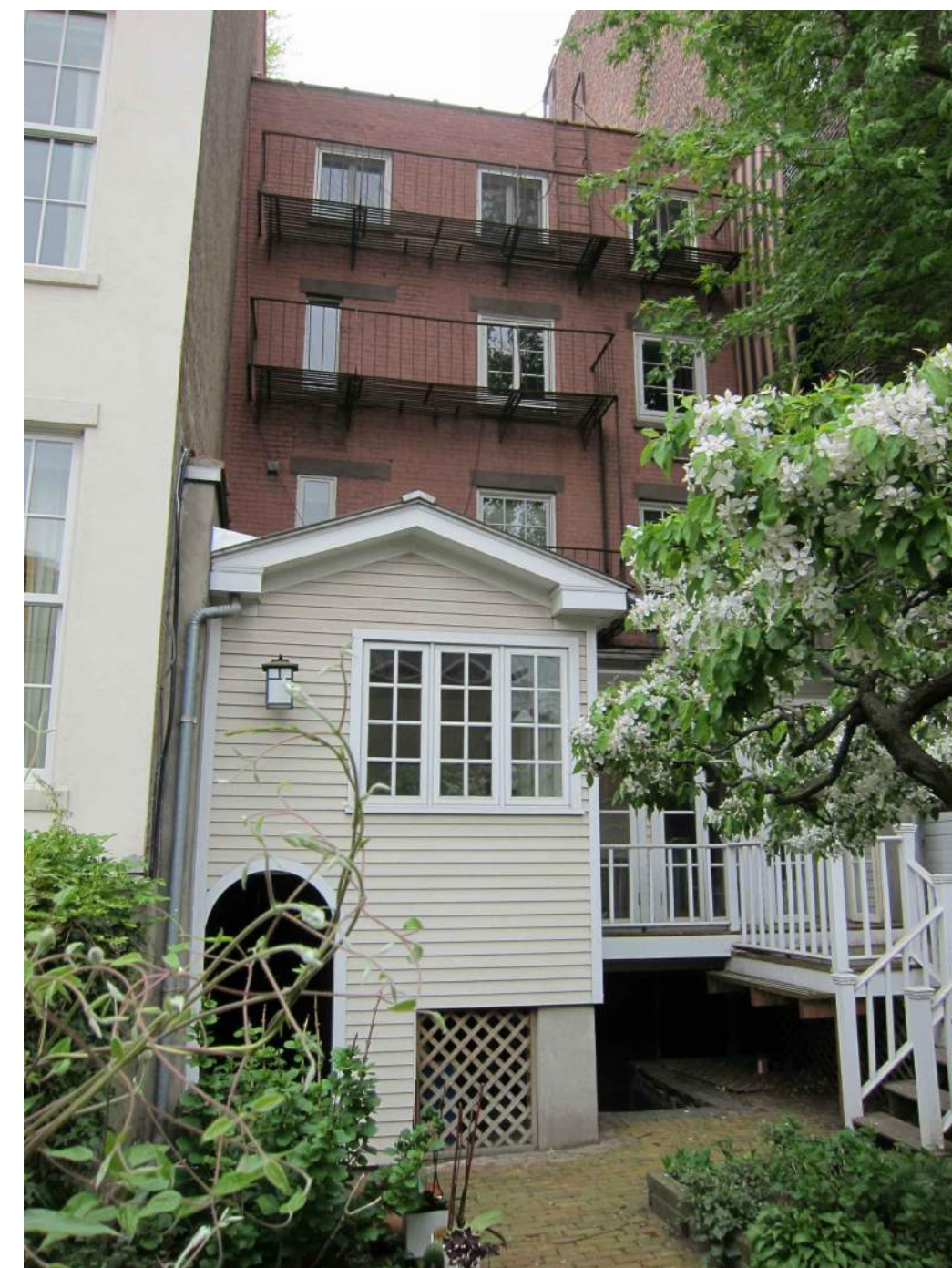
VIEW OF REAR FROM NORTH EAST
