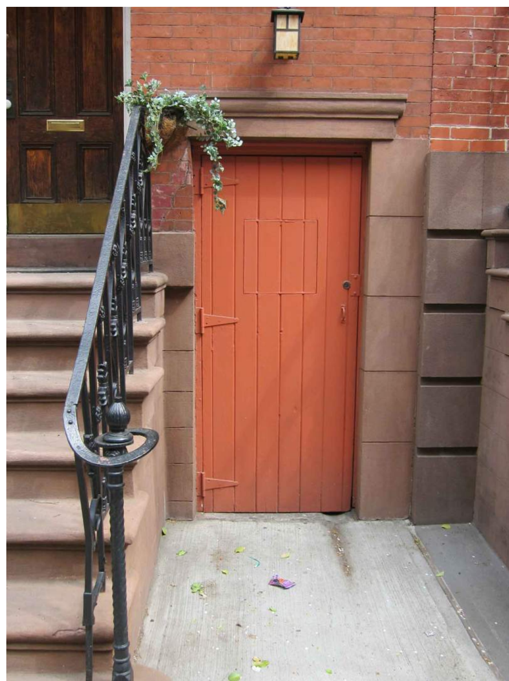
'HORSE-WALK' ENTRANCE ON SOUTH FACADE
