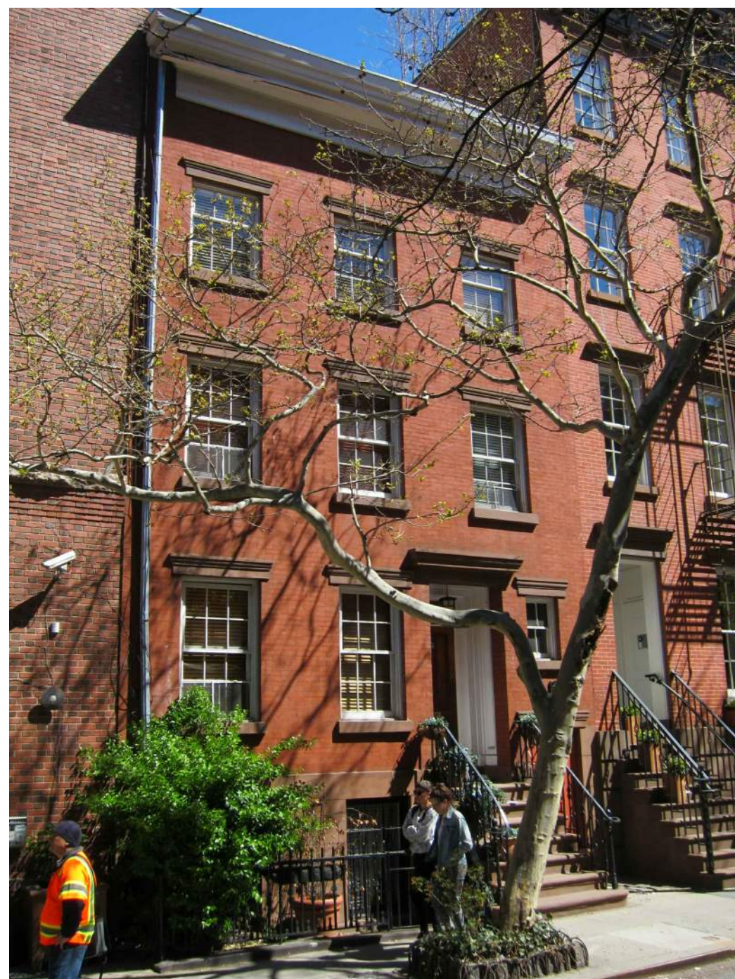
VIEW OF FRONT FACADE FROM SOUTHWEST
