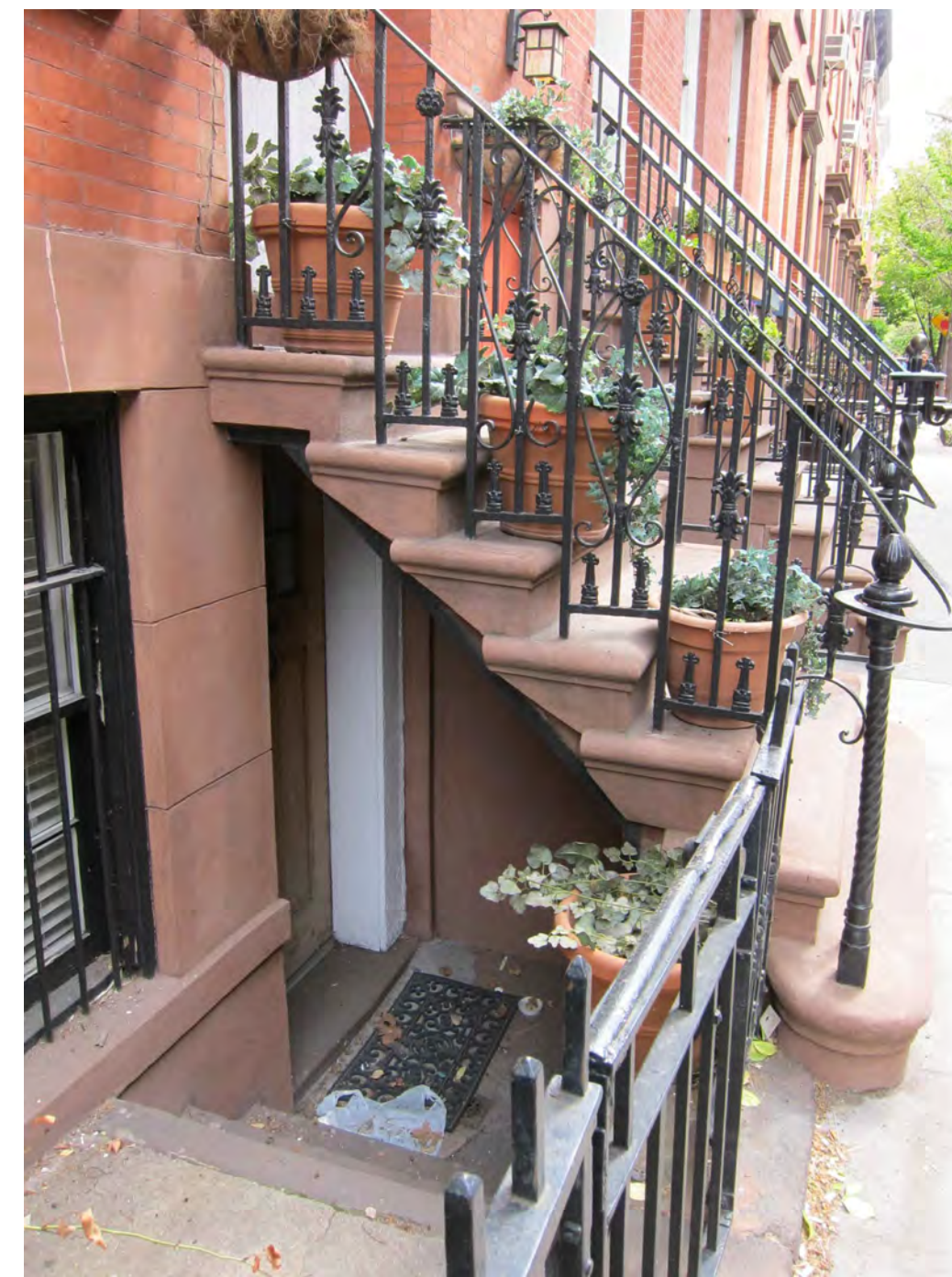
ENTRANCE STOOP AND RAILING
