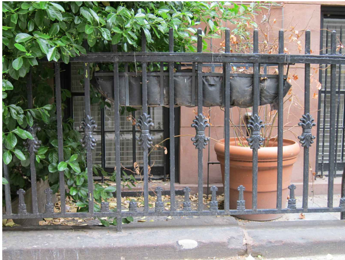
EXISTING RAILING FRONT YARD
