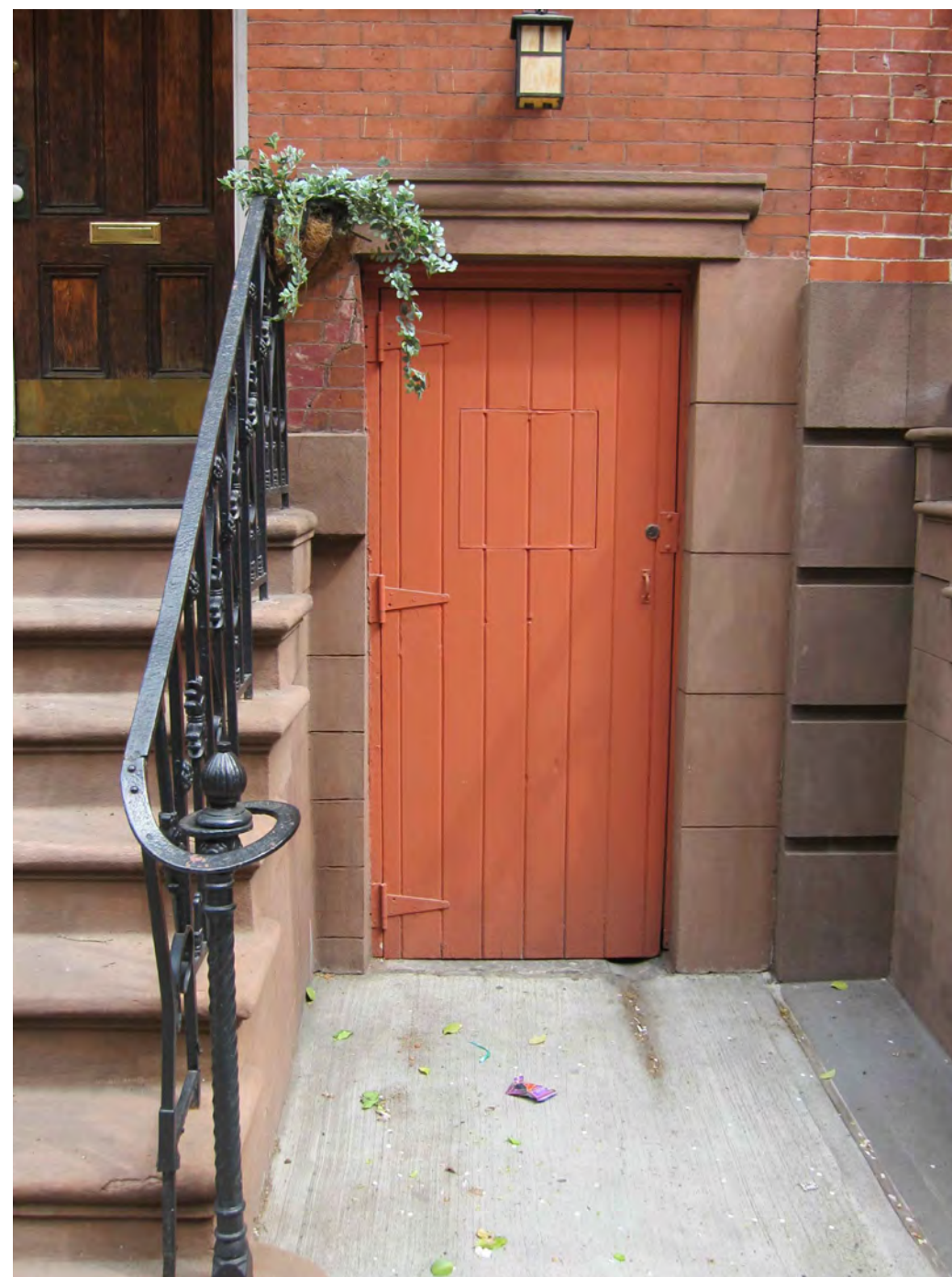
'HORSE-WALK' ENTRANCE ON SOUTH FACADE
