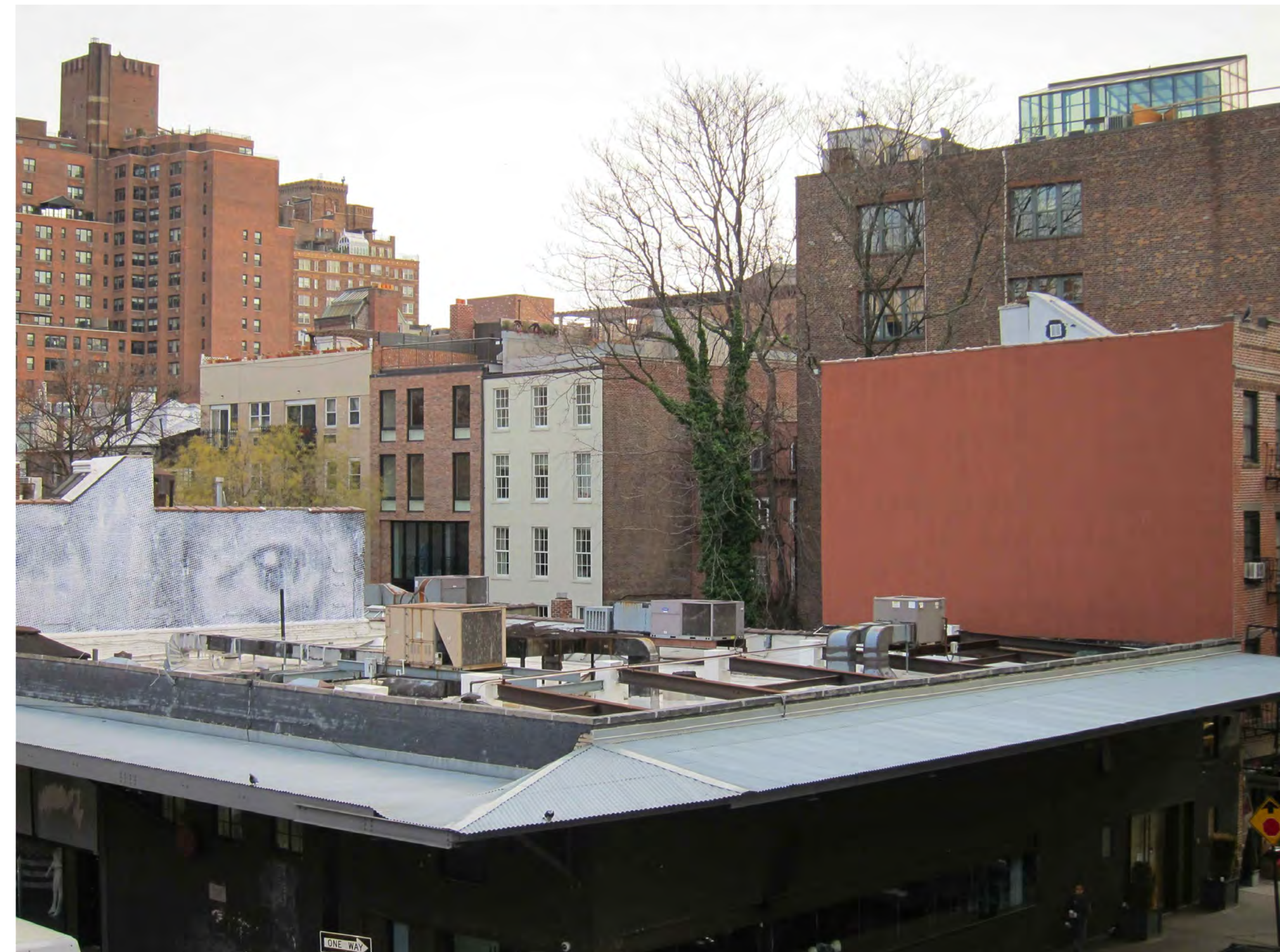
NORTH FACADE FROM HIGH LINE
