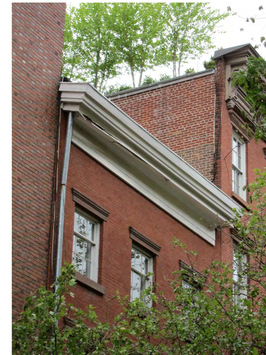
CORNICE ON SOUTH FACADE
