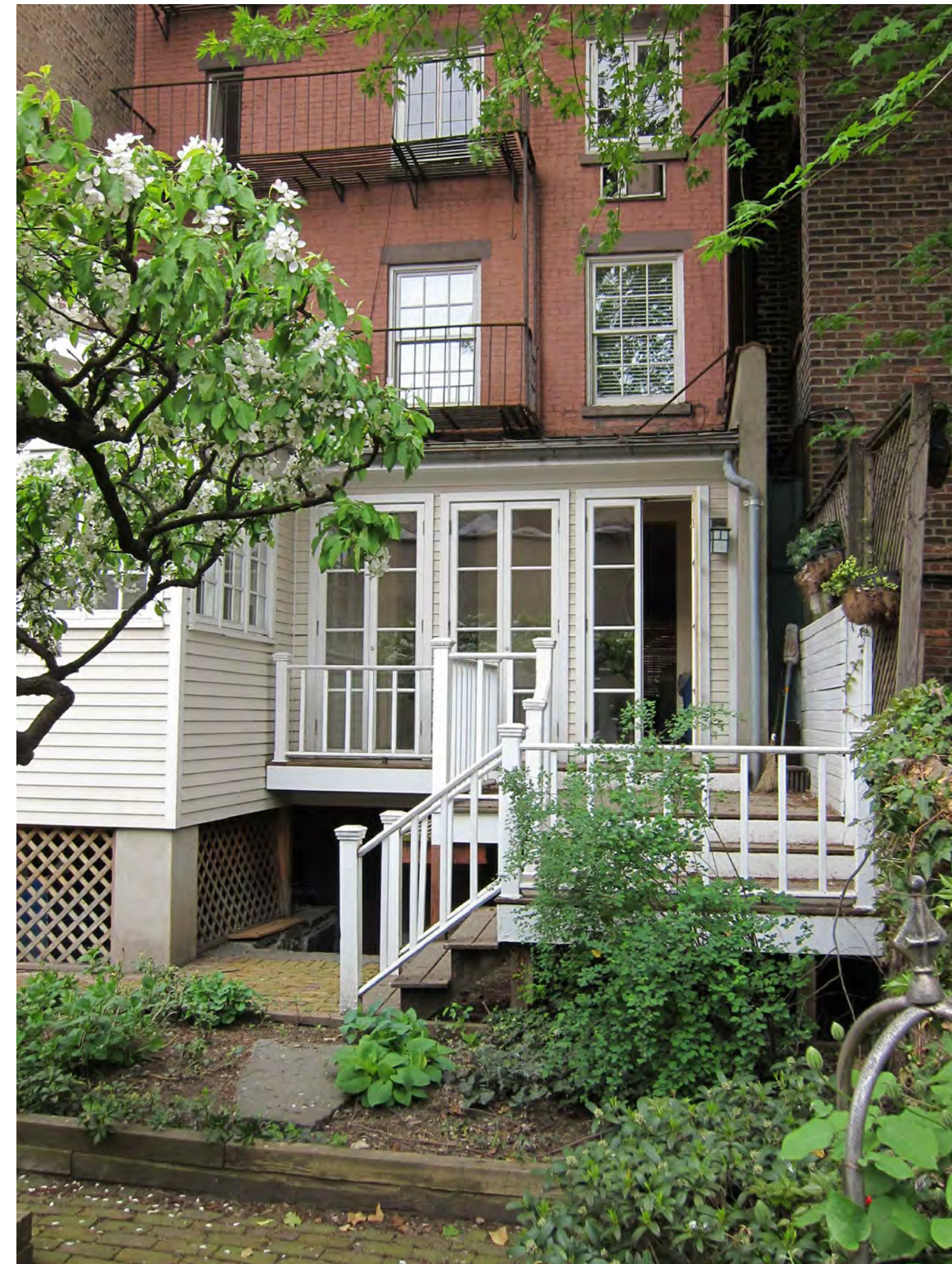
EXISTING NORTH FACADE
