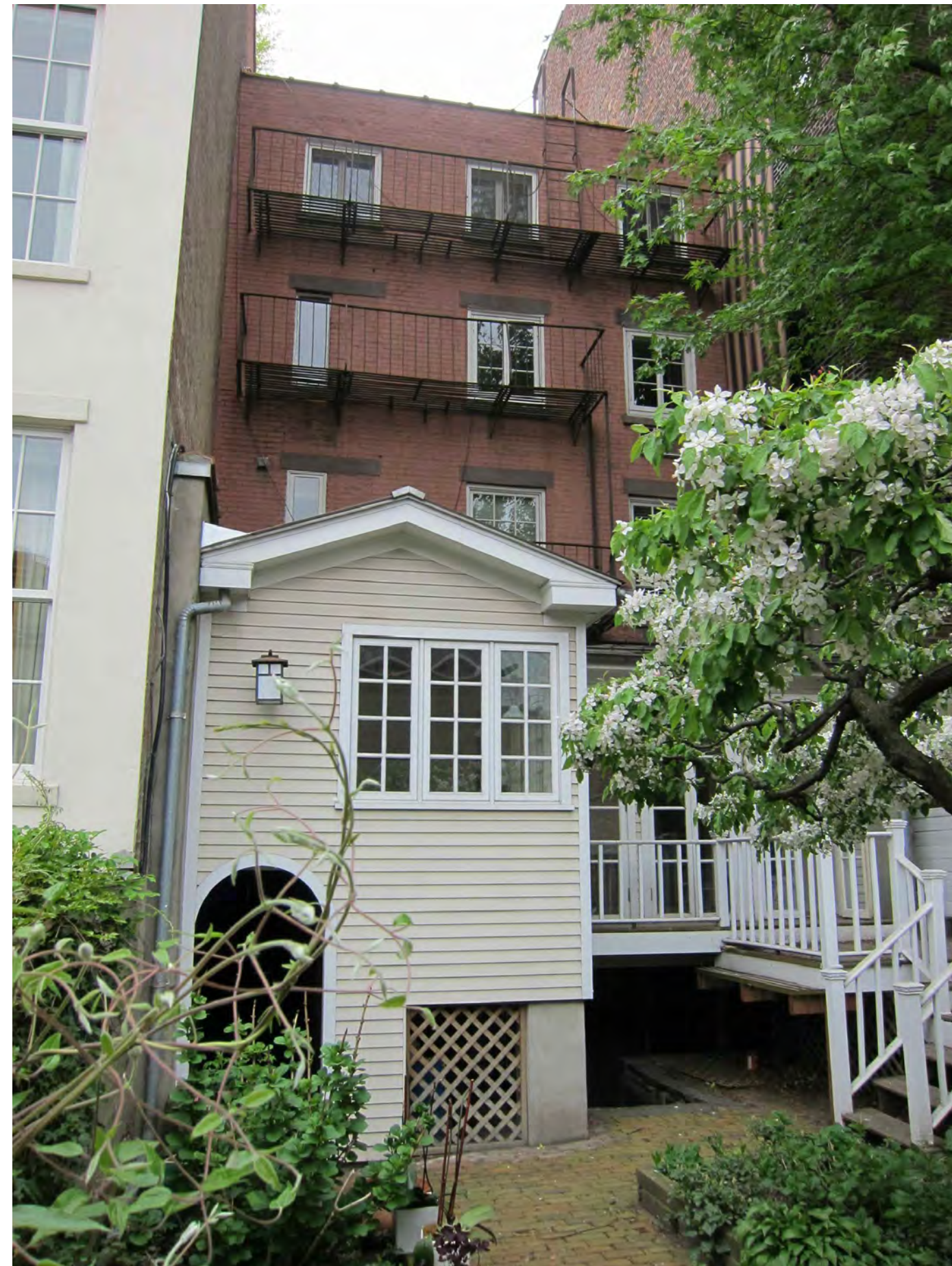
EXISTING NORTH FACADE
