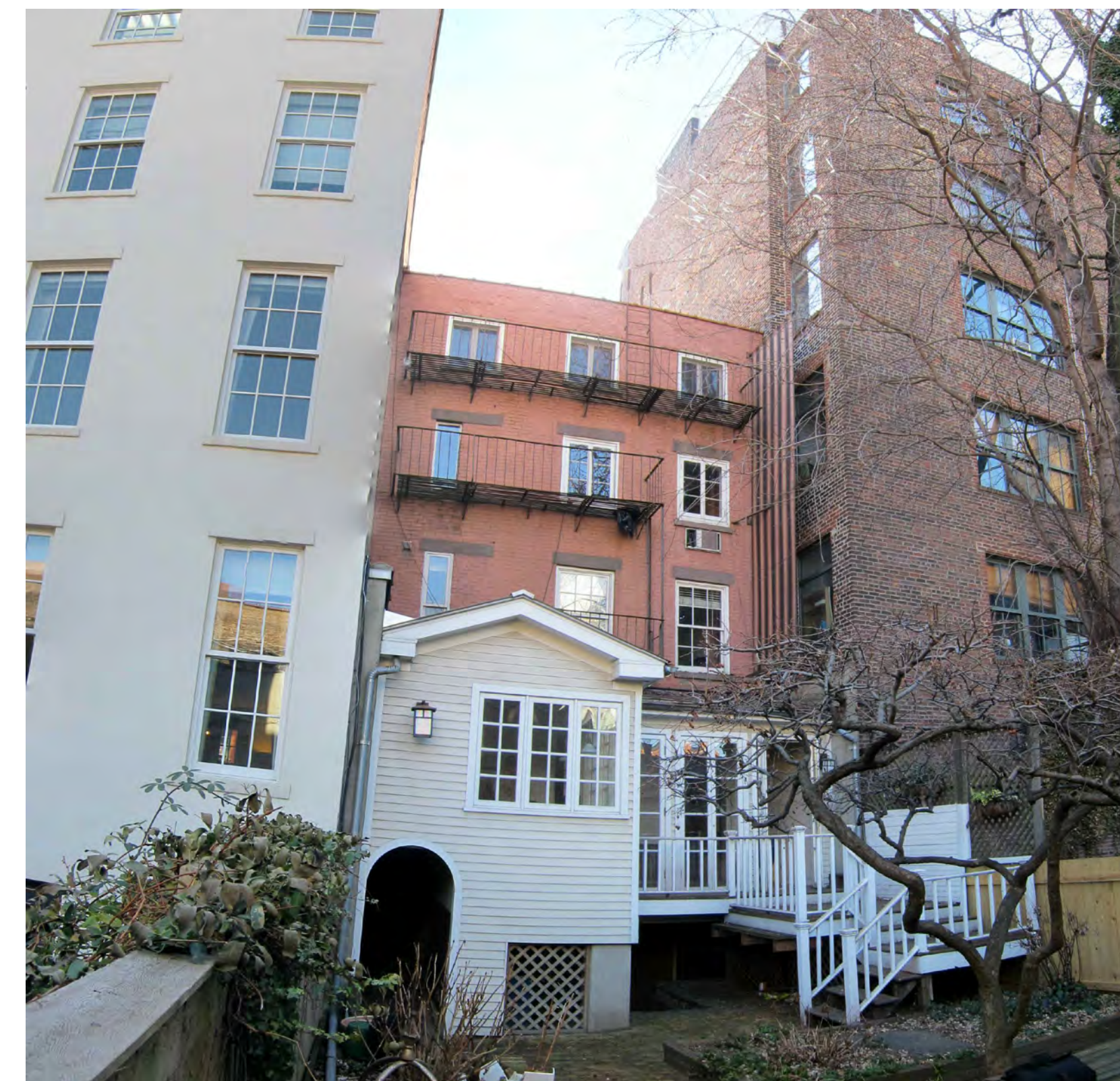
NORTH FACADE AND ADJACENT BUILDINGS
