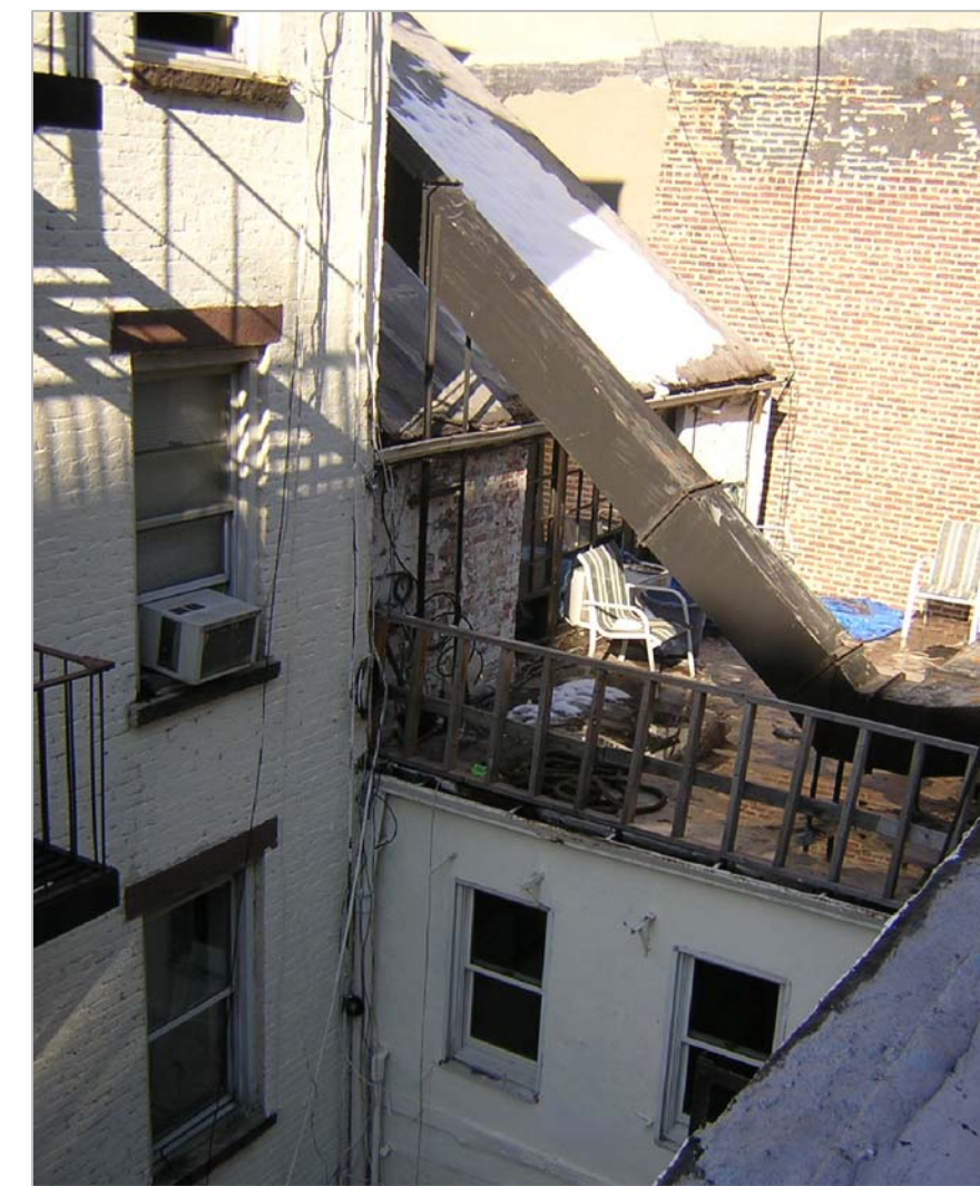
2 VIEW FROM ADJ. ROOF PRIOR TO CONSTRUCTION
