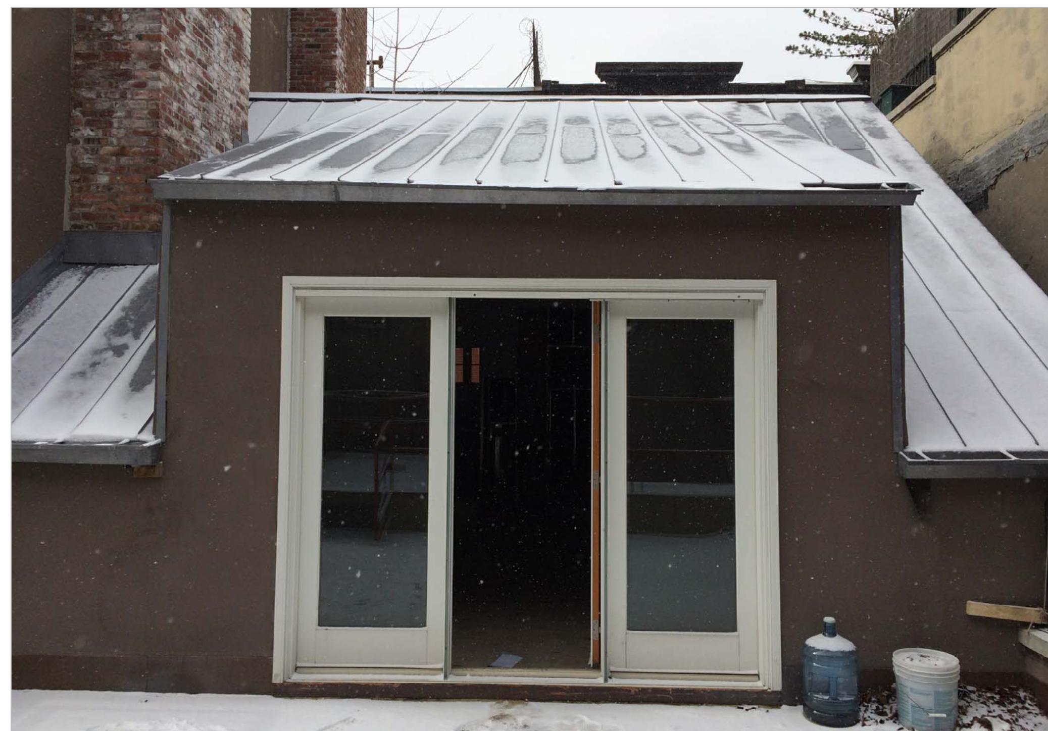
6 NEW AS-BUILT SHED DORMER AT REAR OF ROOF
