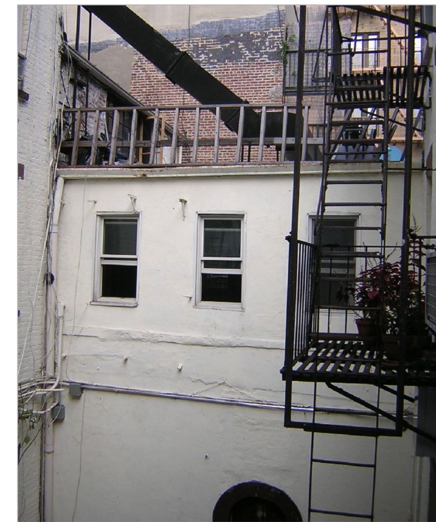
5 VIEW FROM ADJ. PROPERTY 2ND FL - PRIOR TO CONSTRUCTION
