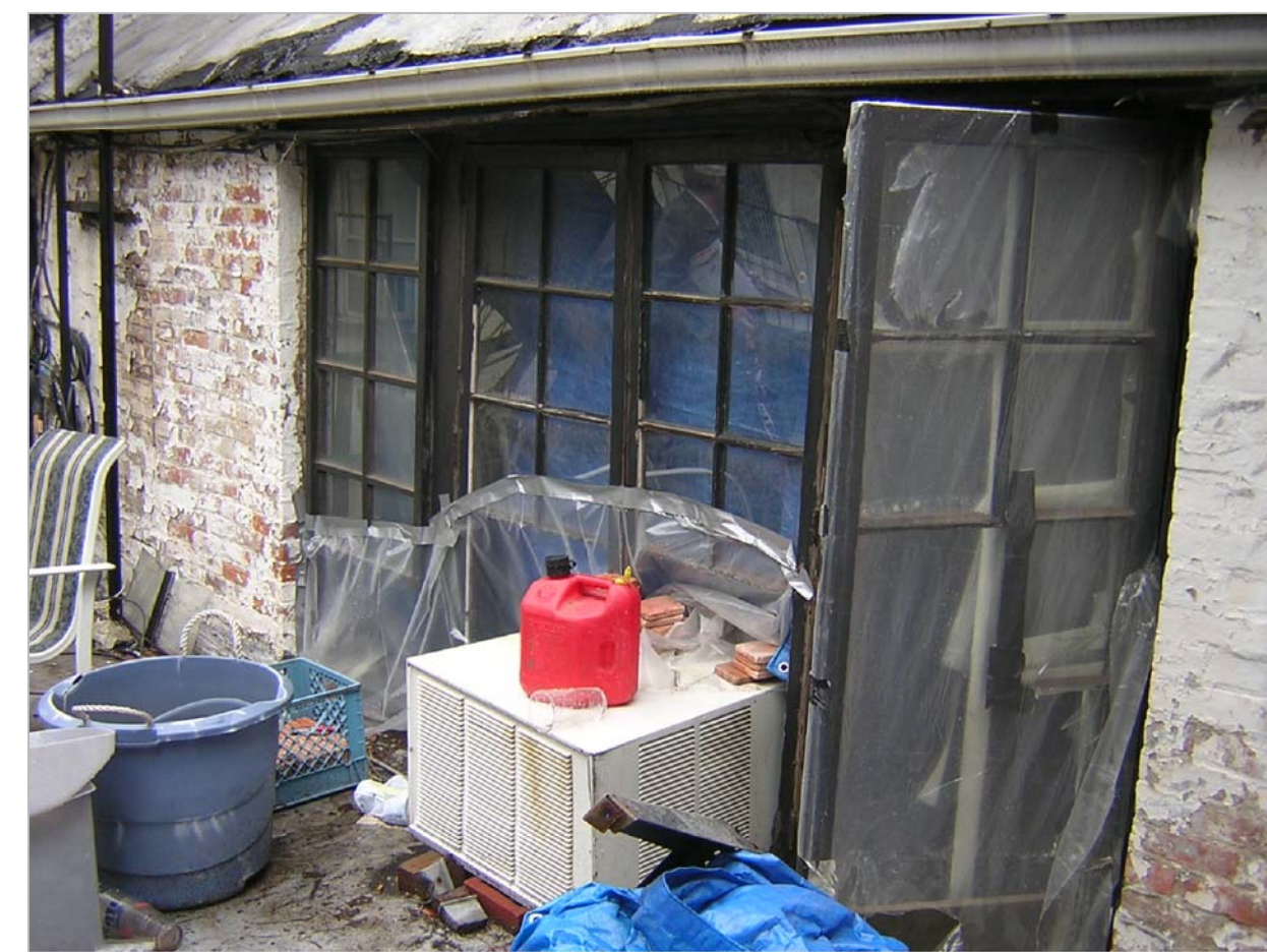
3 REAR FACADE OF ROOF PRIOR TO CONSTRUCTION
