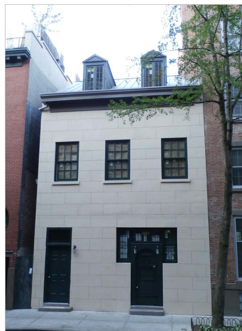
8 FRONT FACADE AS-BUILT CONDITIONS
