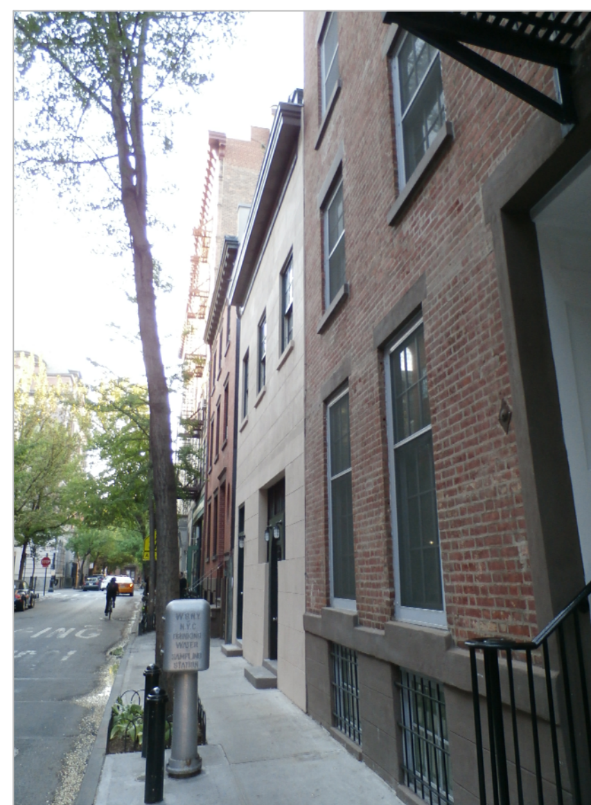
9 VIEW ALONG BEDFORD ST AS-BUILT CONDITIONS
