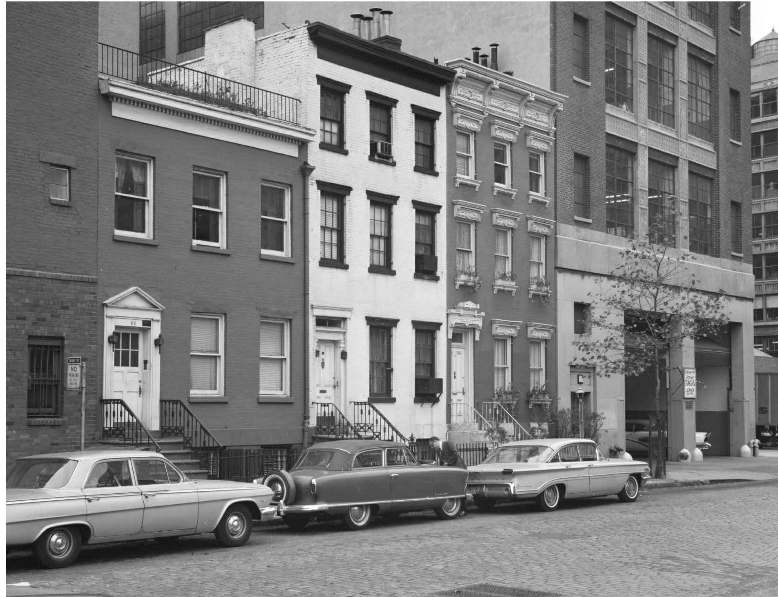
1 EXISTING FRONT FACADE (LPC DESIGNATION PHOTO) N.T.S.
