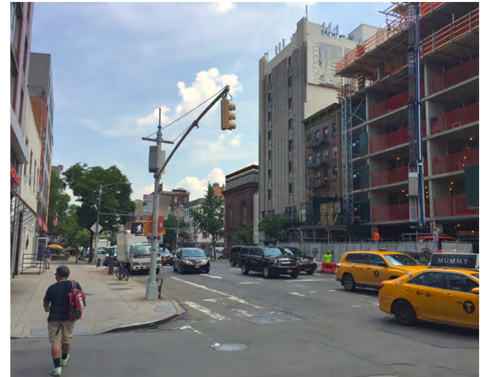
VIEW FROM 2nd AVE LOOKING NORTH
