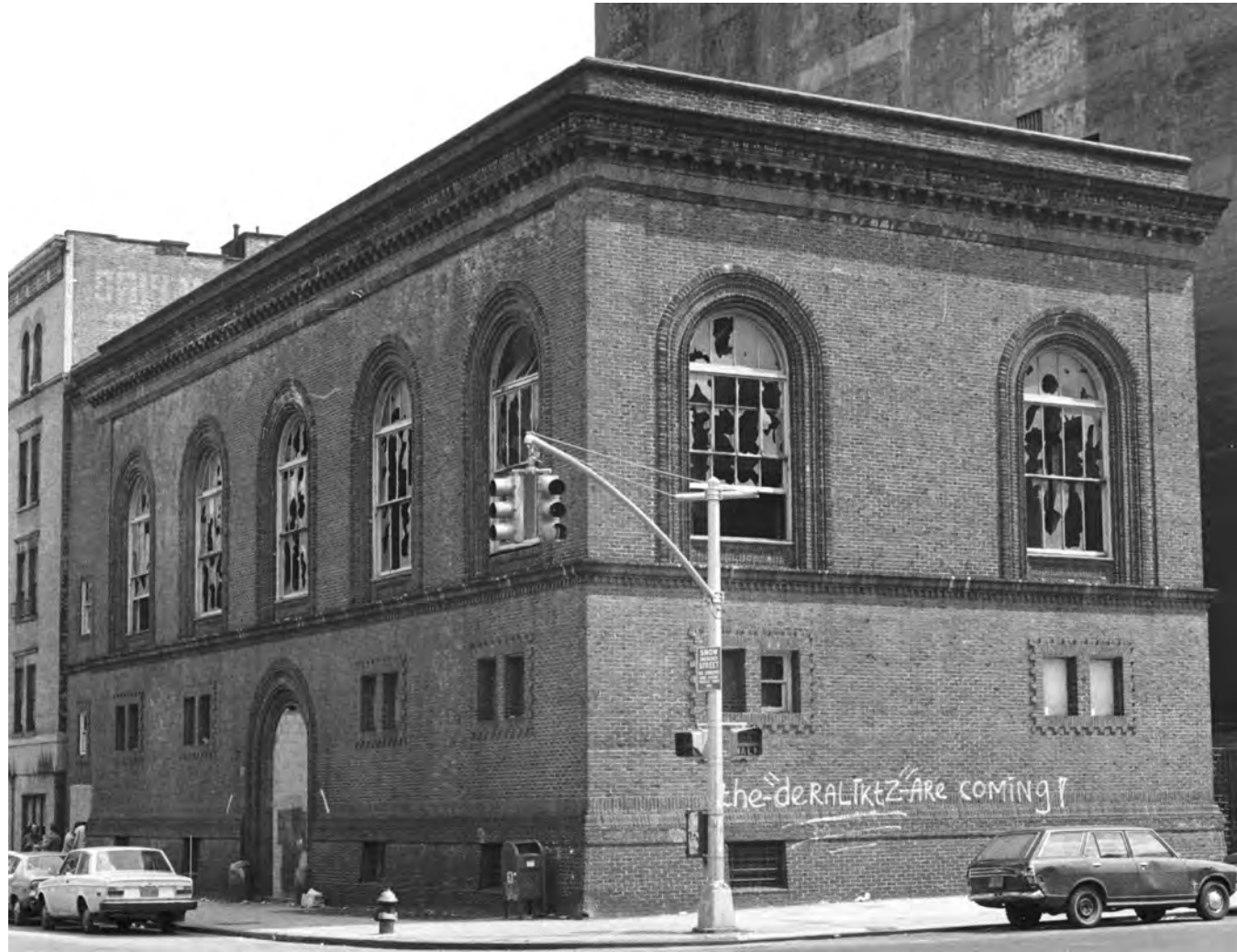
Conditions of building ca. 1980's
