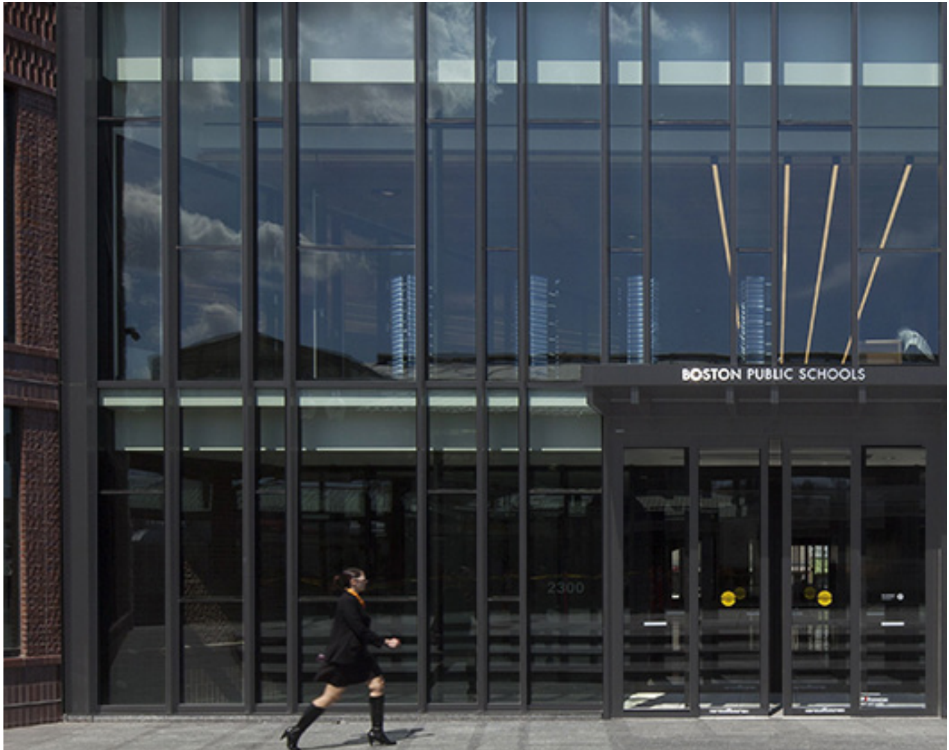
NEW STOREFRONT: STEEL MULLIONS WITH RECESSED GLAZING
