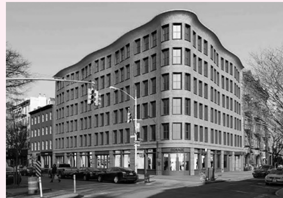
Some of the many controversial approvals by the LPC under the recent chair: (top to bottom) 11 Jane Street, 145 Perry Street, and 540 Hudson Street
