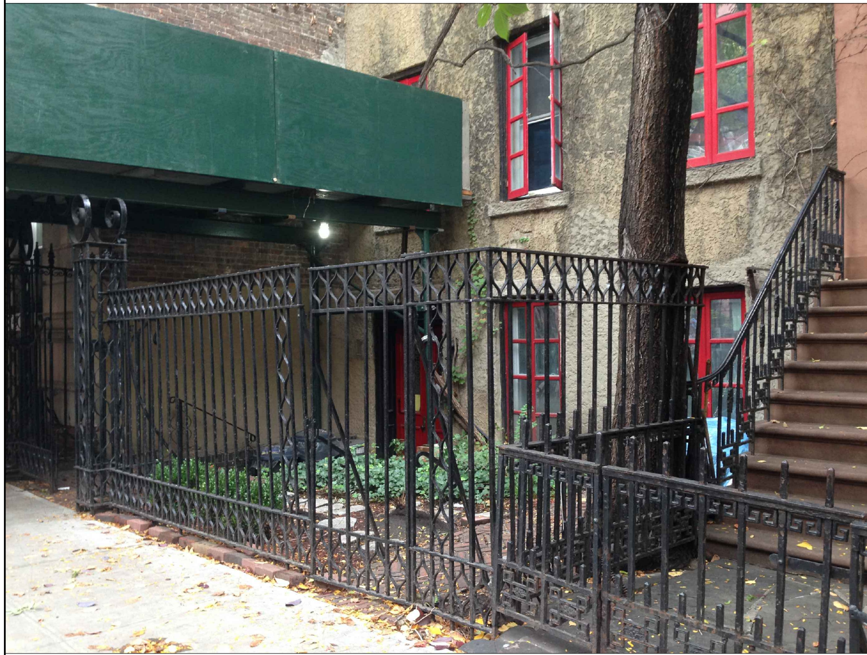
A VIEW 235 WEST 11TH STREET - RESIDENCE
