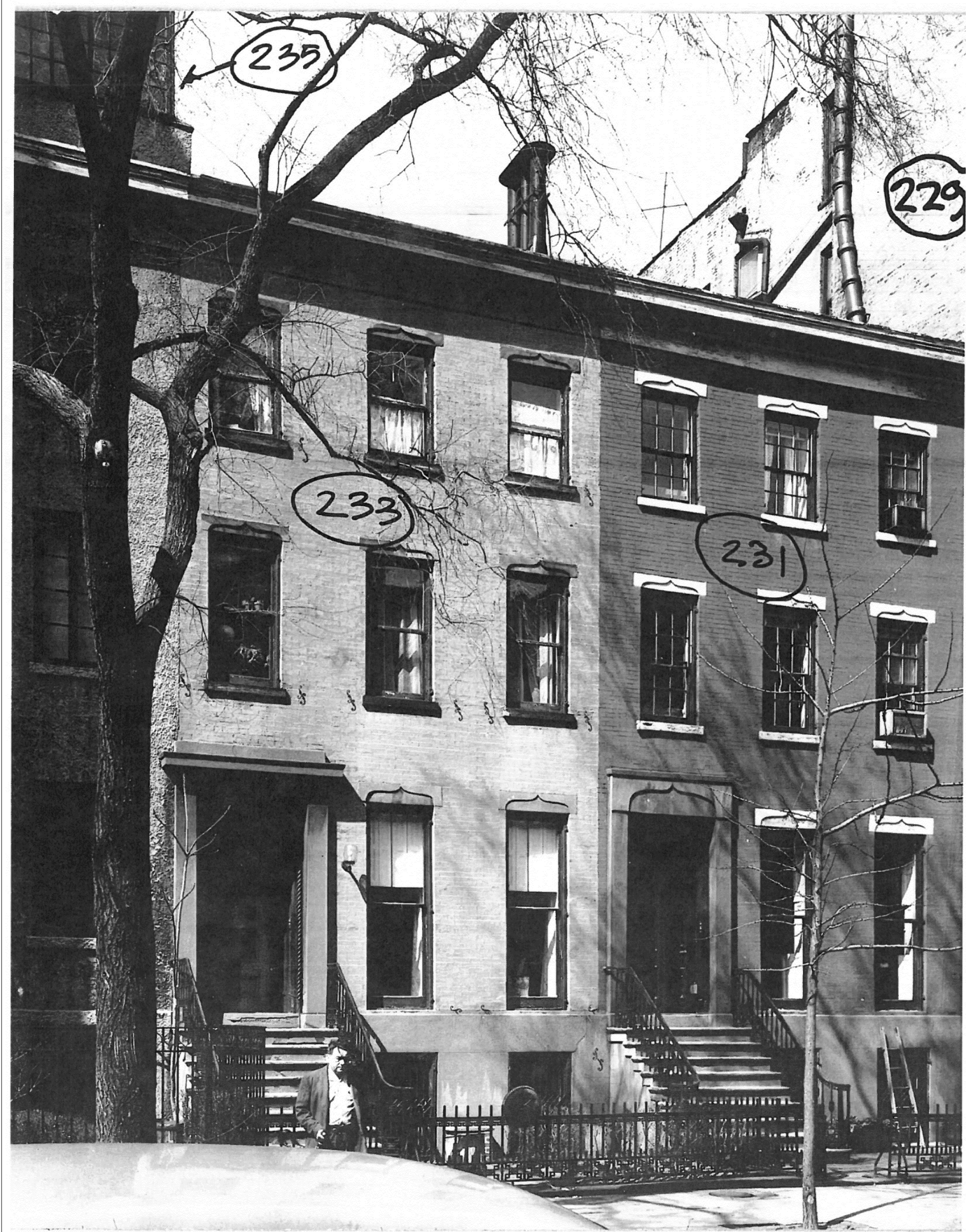
(3) LPC - DESIGNATION PHOTO
