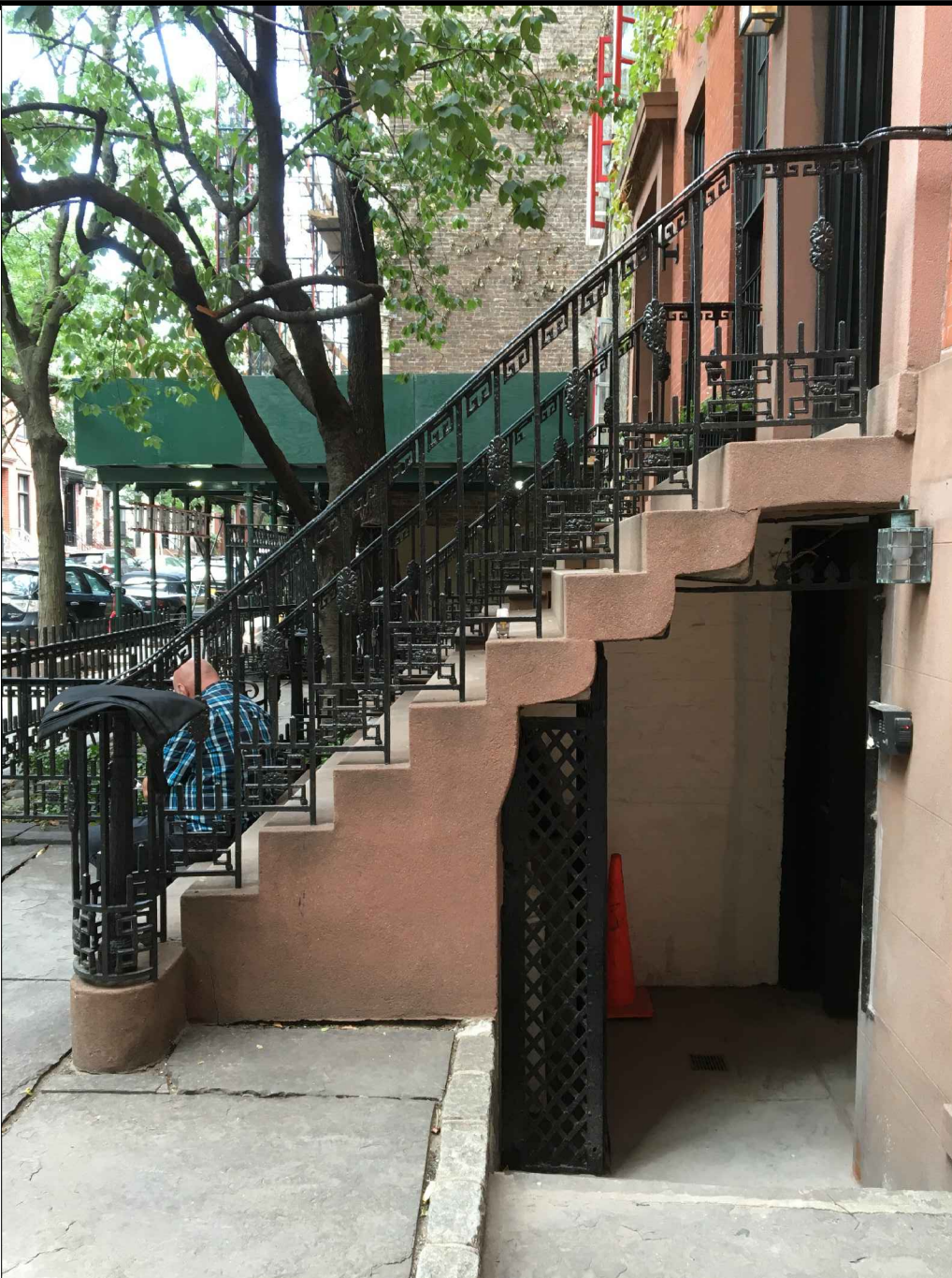
8 VIEW OF THE STAIRS
