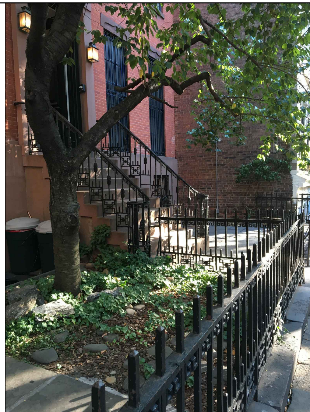
7 VIEW OF THE STAIRS
