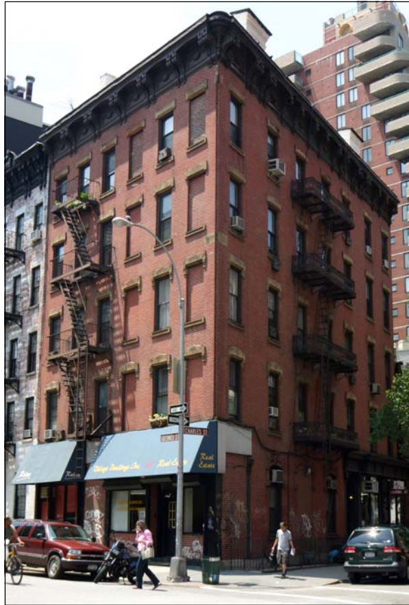
716-718 Greenwich Street aka 128 Charles Street
