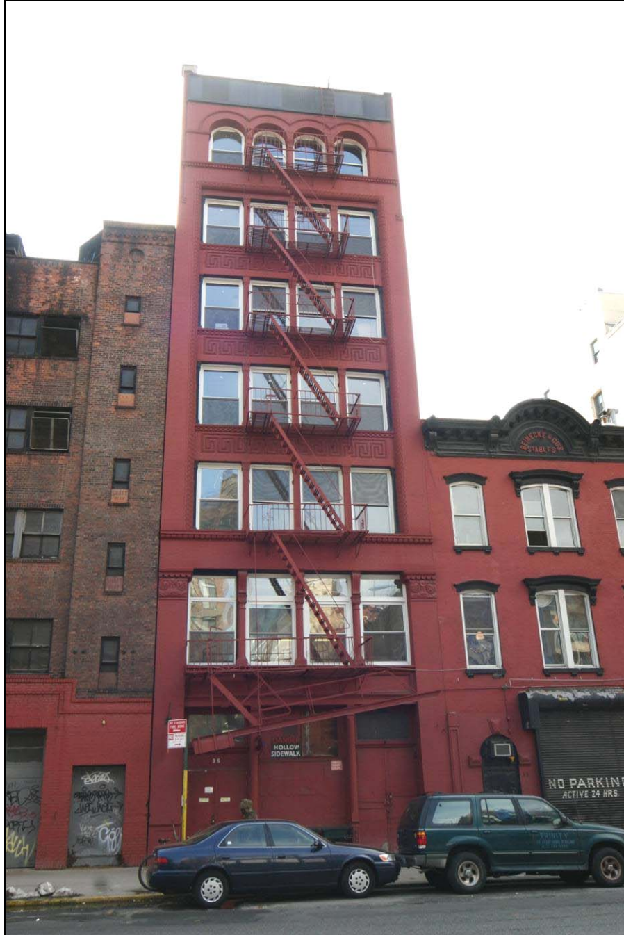
Figure 38 35 Great Jones Street Cleverdon & Putzel, 1893-94 Photo: Carl Forster
