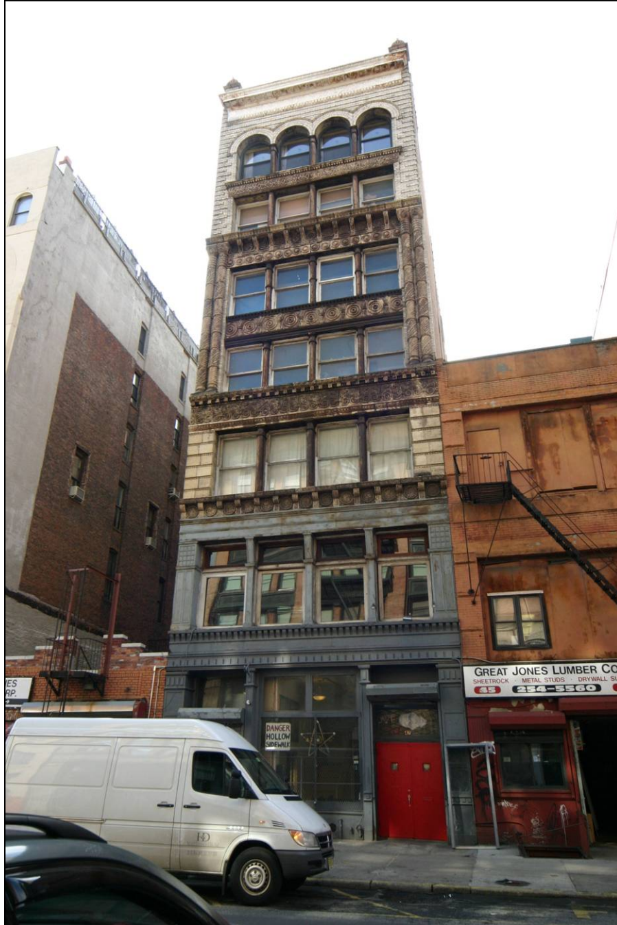
Figure 44 47 Great Jones Street Cleverdon & Putzel, 1895-96 Photo: Carl Forster
