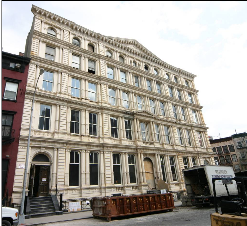
Figure 23 (Former) Bond Street Savings Bank aka Bouwerie Lane Theatre 330 Bowery (Bond Street elevation) Henry Engelbert, 1873-74 Photo: Carl Forster
