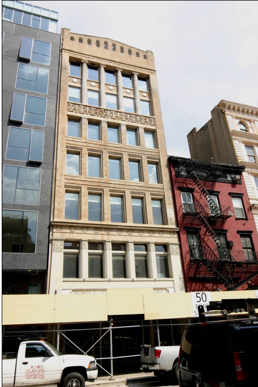
Figure 20 50 Bond Street Cleverdon & Putzel, 1896-97 Photo: Carl Forster
