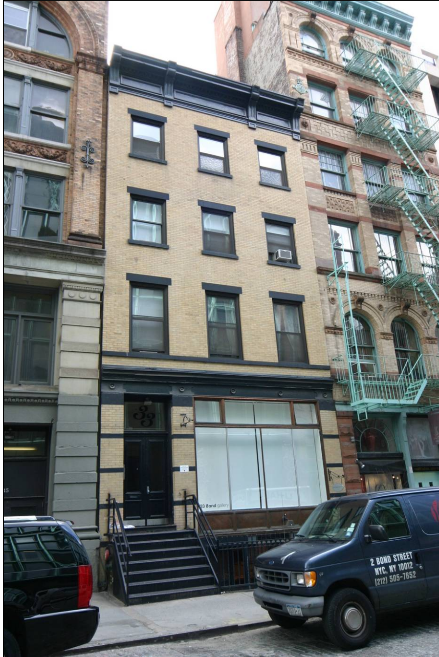
Figure 5 33 Bond Street c. 1830-31; altered by Cleverdon & Putzel, 1911 Photo: Carl Forster
