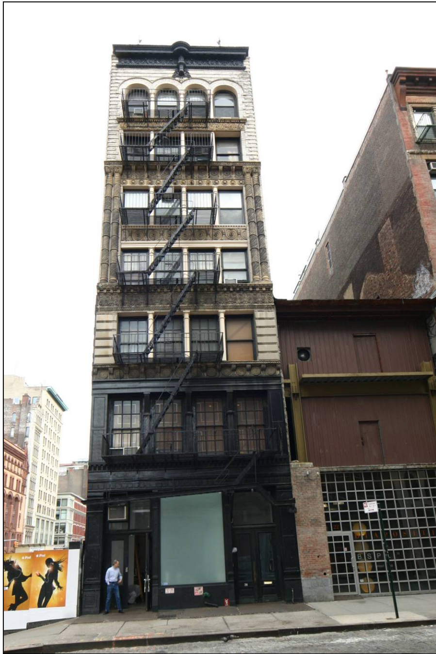
Figure 11 20 Bond Street Cleverdon & Putzel, 1894-95 Photo: Carl Forster
