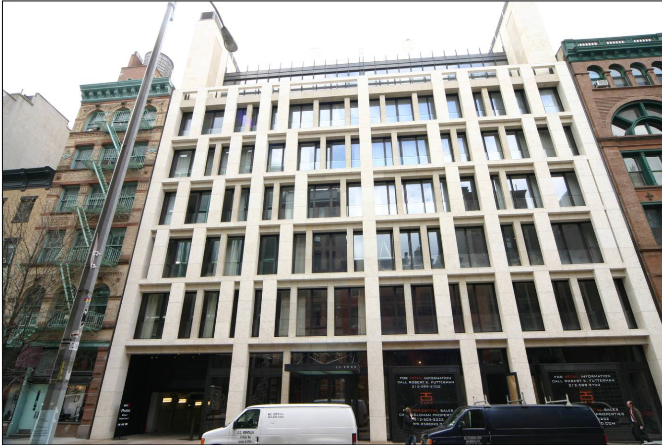
Figure 3 25 Bond Street George Schieferdecker, BSK Architects, 2003-2008 Photo: Carl Forster
