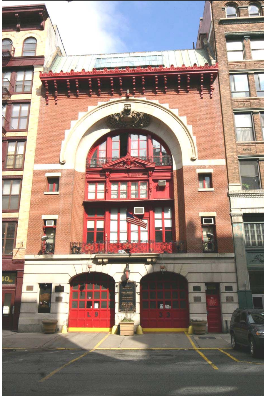
Figure 49 Firehouse Engine Co. Thirty-Three 42-44 Great Jones Street Ernest Flagg and W. B. Chambers, 1898-99 Photo: Carl Forster
