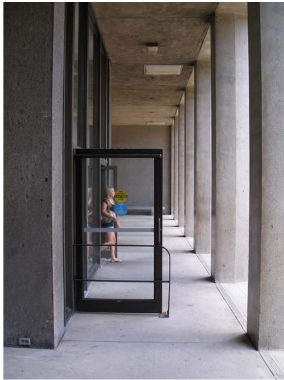
Arcade, 100 Bleecker Street, view south
