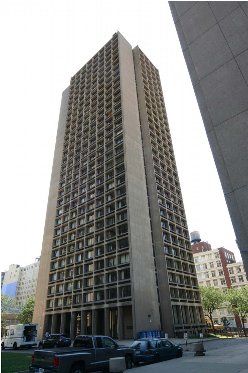
110 Bleecker Street, north and west facades
