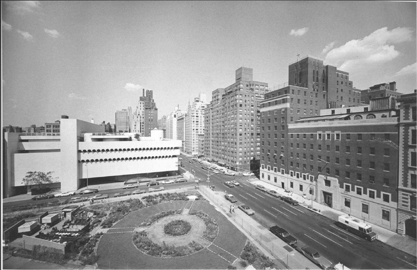
Edward and Theresa O'Toole Medical Services Building of St. Vincent's Hospital, 1973-2010
