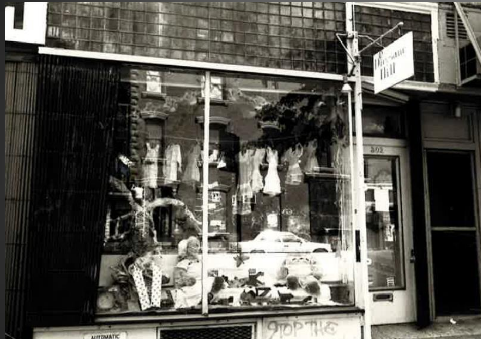
Original Storefront Ca. early 1980s
