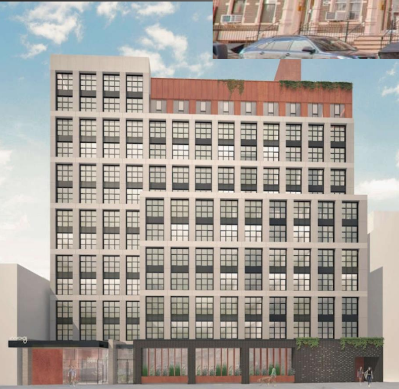
12-story 'Moxy' Hotel to be built on site
