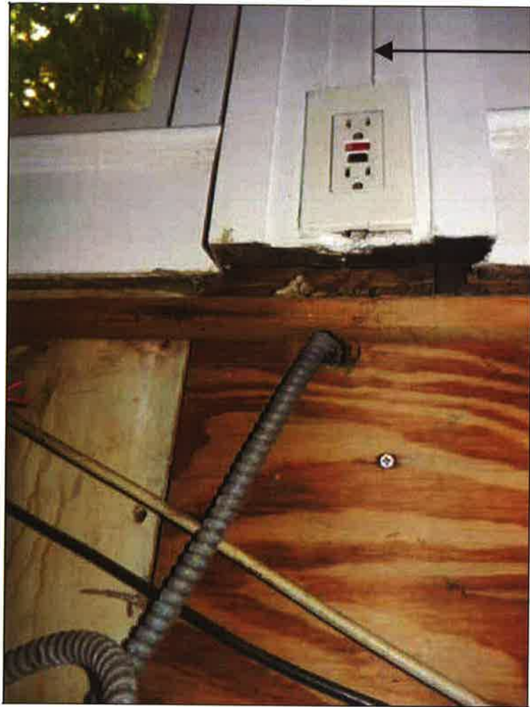
Figure 6: Historic wood column trim is applied over wall board
