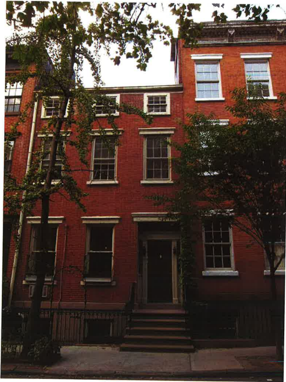
1 - 313 W 4TH STREET EXISTING FACADE
