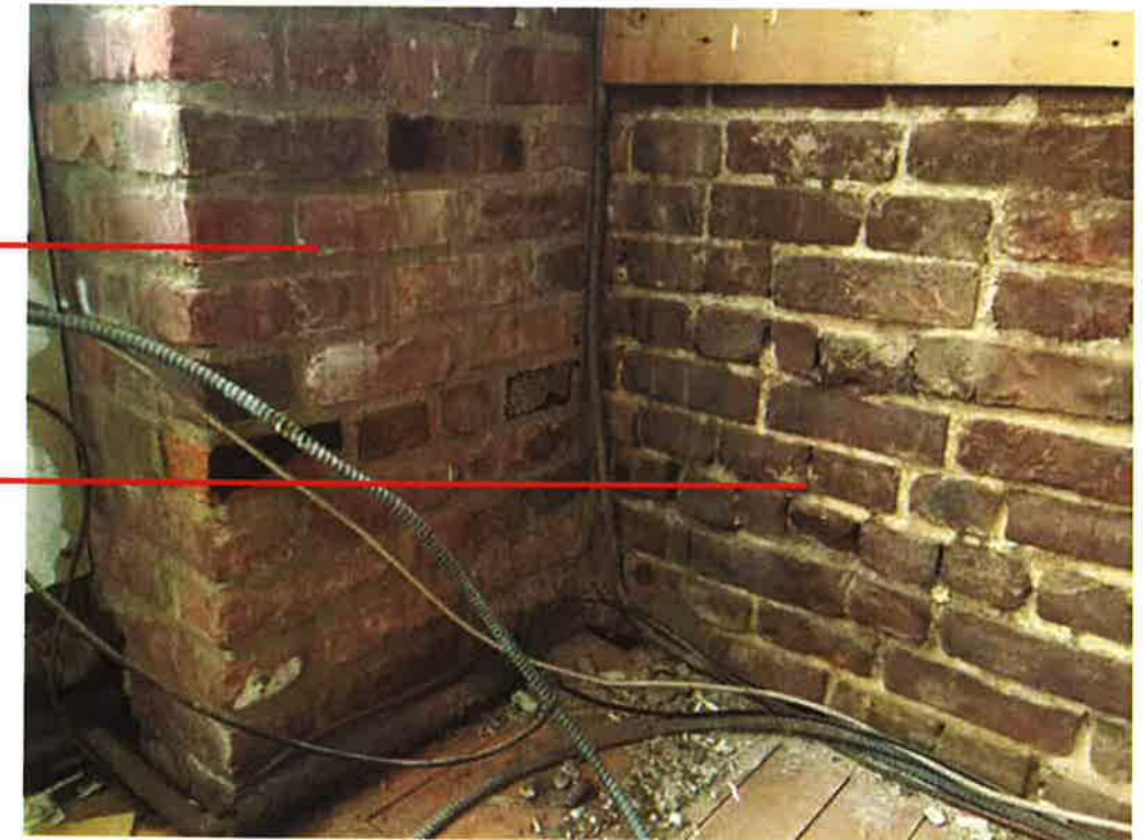
2 - BRICK CONDITION AT REAR YARD EXTENSION AT 1ST FLOOR
