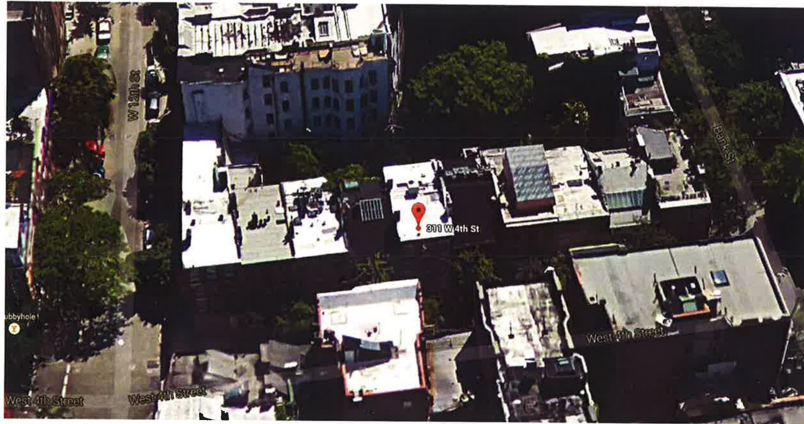
1 - AERIAL SITE IMAGE
