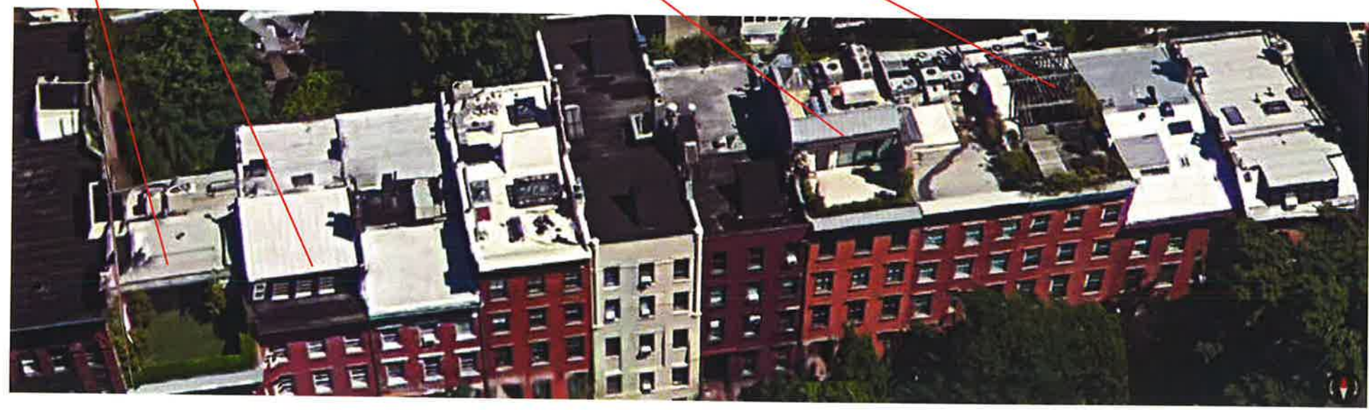
3 - BANK STREET BTW W4TH AND GREENWICH AVE
