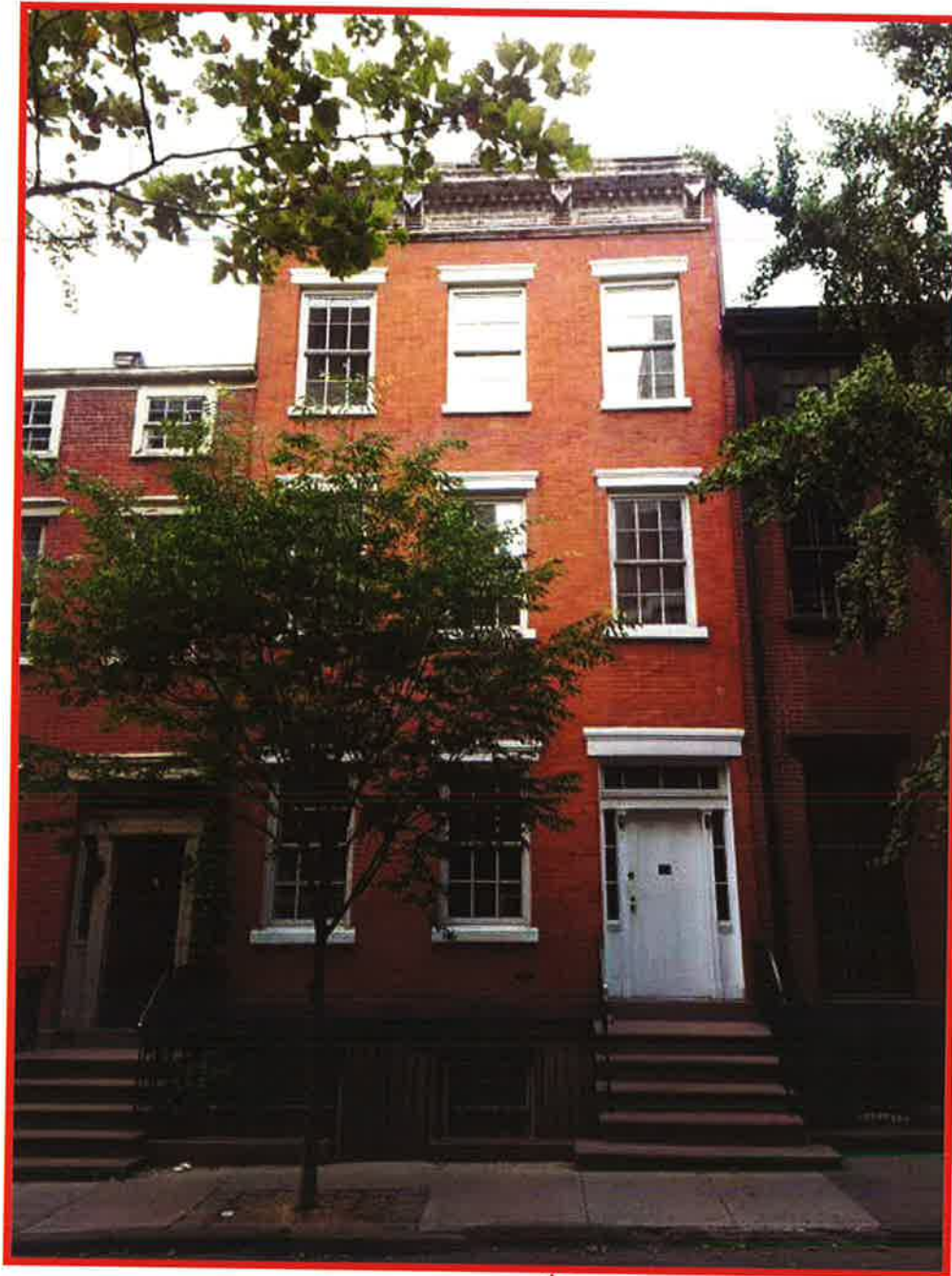
2 - 311 W 4TH STREET EXISTING FACADE
