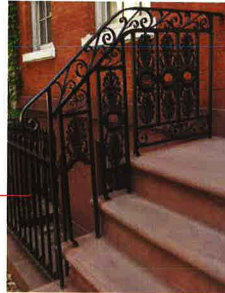
3 - EXISTING RAILING PATCH, PAINT AND RESTORE IRONWORK TO ORIGINAL CONDITION
