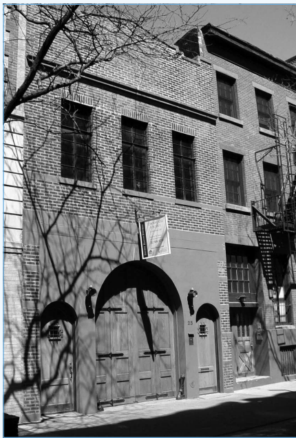
The former stable at 23 Cornelia Street, before work commenced and the iconic horse hooves around the entrance were removed.
