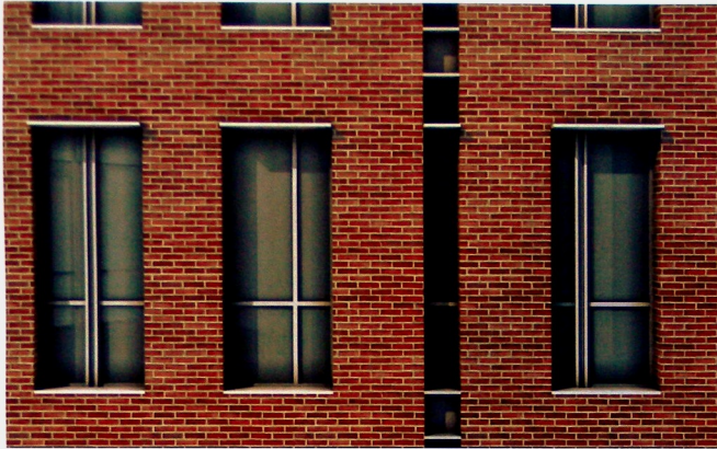
1 View Of Typical Brick Facade Detail
