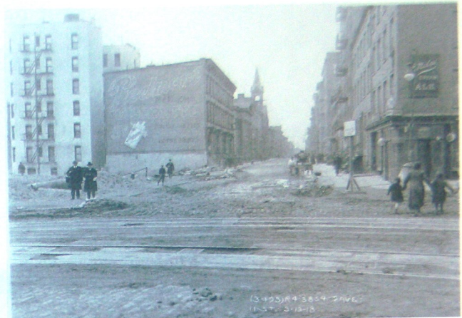
3 1918 Site After Subway Construction Was Completed (NYHS)
