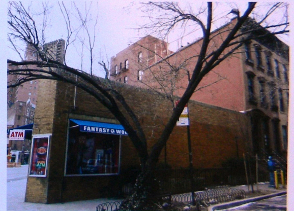
4 West 11th Street Facade
