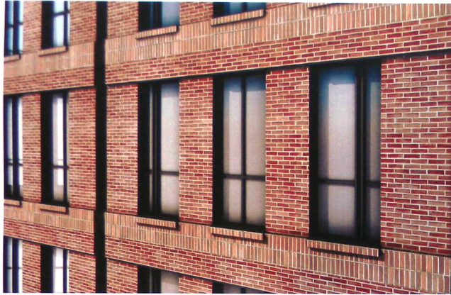
1 View Of Typical Brick Facade Detail
