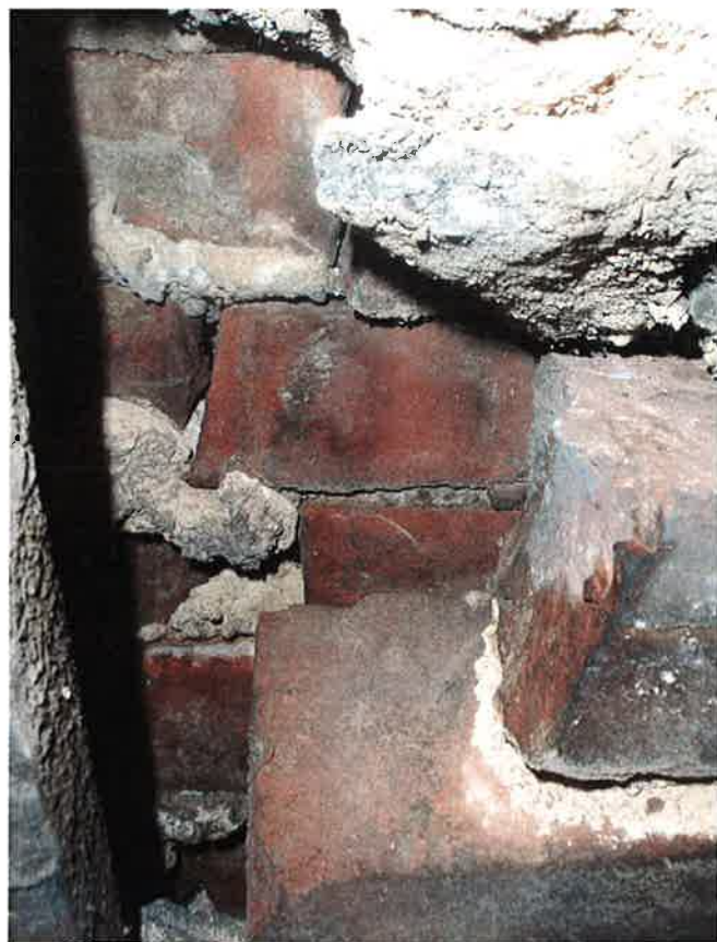
5 PROVE @ SOUTH FACADE (INTERIOR) A-5
