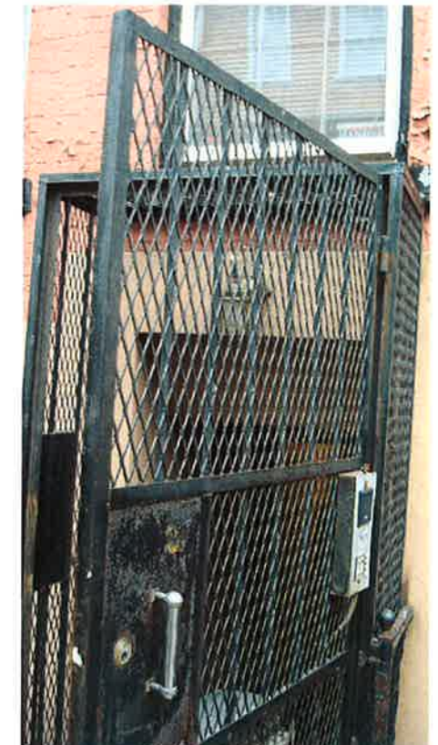
7 GATE @ BASEMENT TO BE REMOVED A-4
