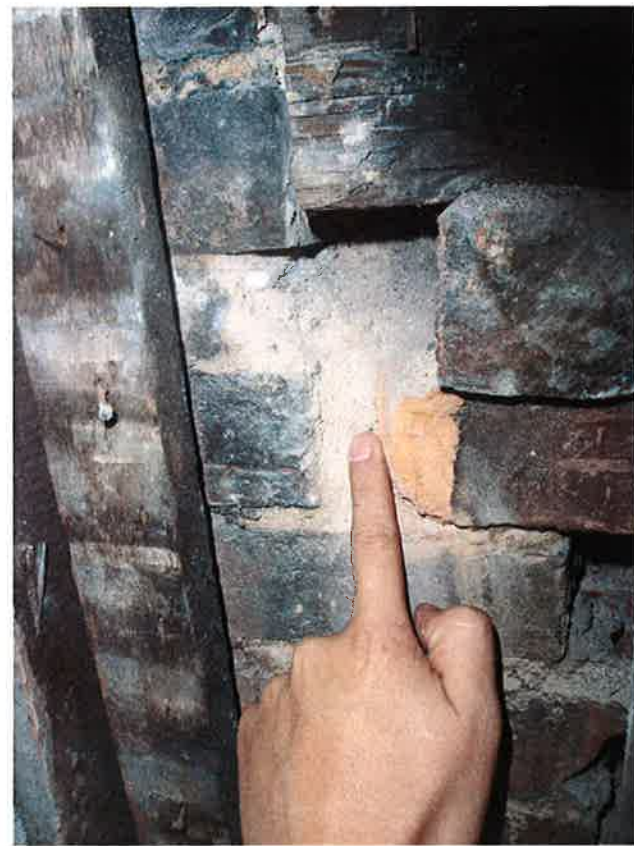
2 PROVE @ SOUTH FACADE (INTERIOR) A-5
