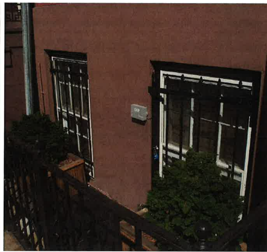
5 TYPICAL WINDOWS AT BASEMENT A-4
