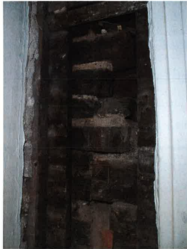
1 PROVE @ SOUTH FACADE (INTERIOR) A-5
