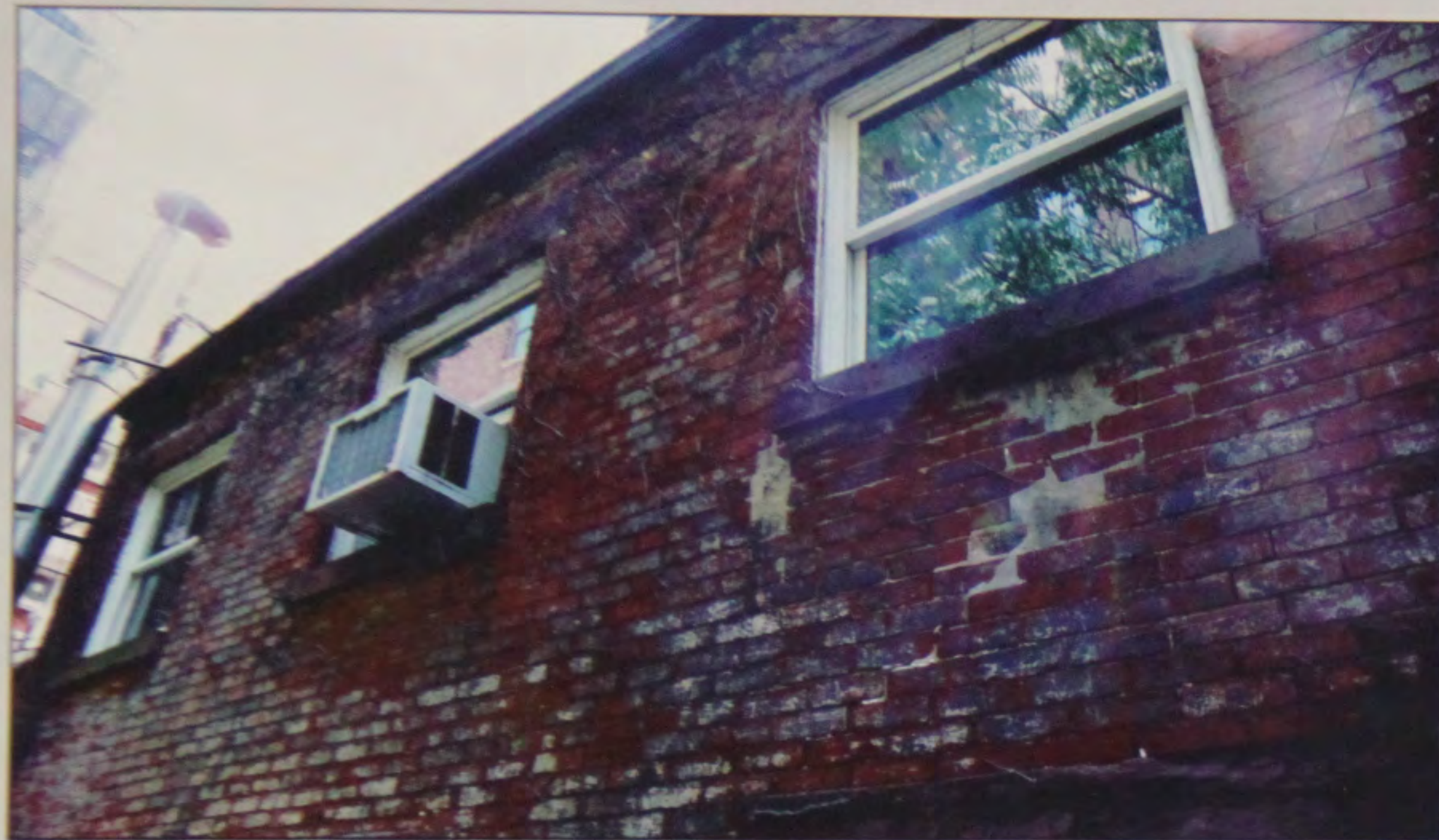
27 EAST 11 STREET (NY) - 3RD & 4TH FLOOR REAR
