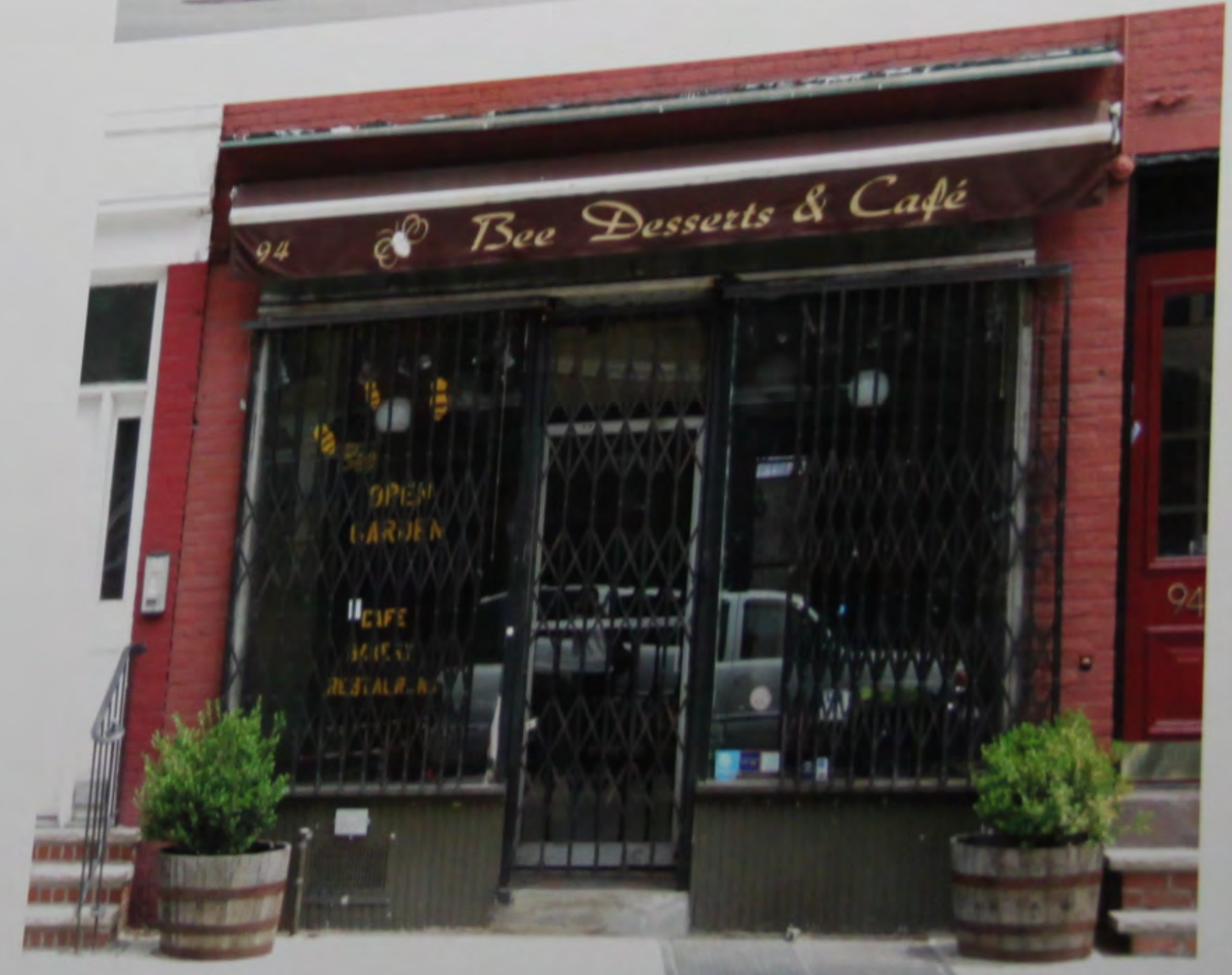
CURRENT CONDITION, FRONT VIEW
