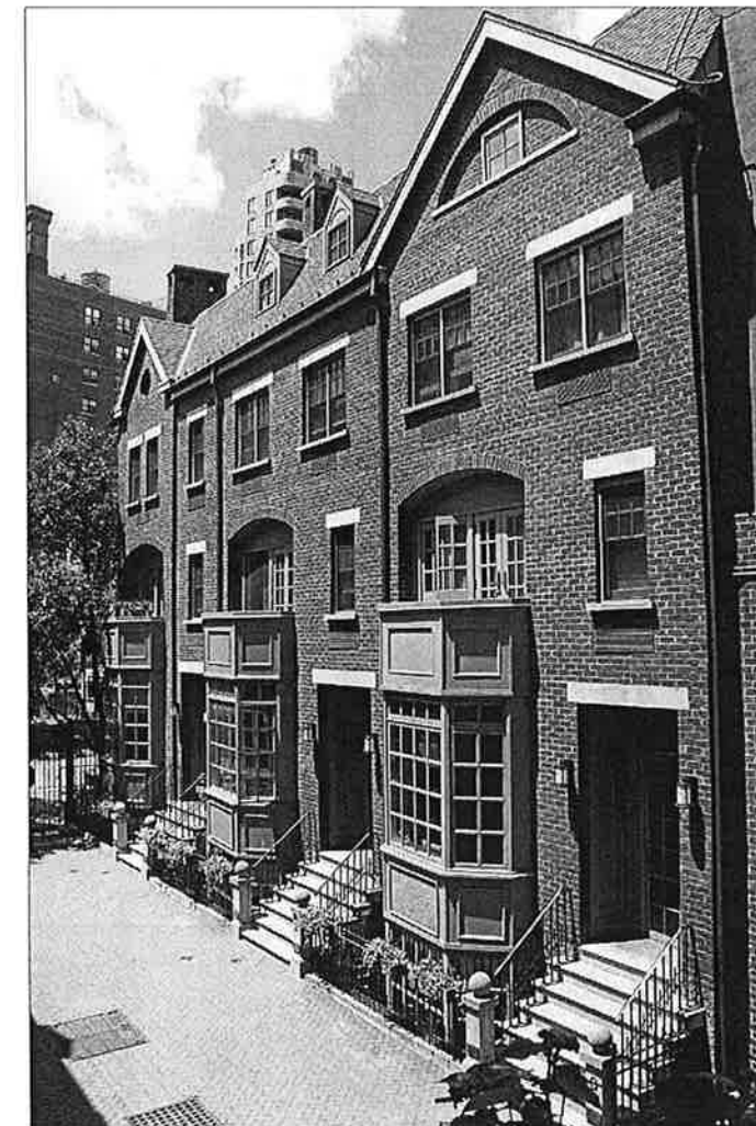
5 VIEW OF FRONT FACADE
