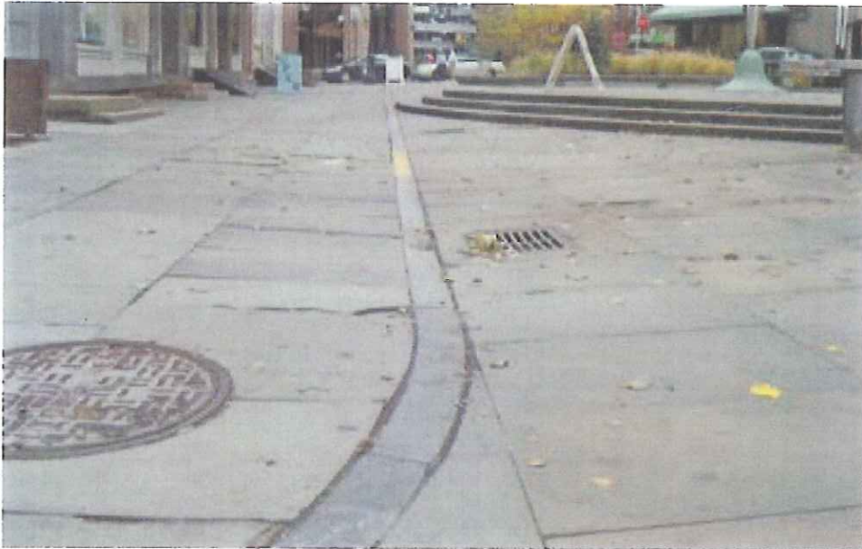
Granite Band in pavement to match new curb
