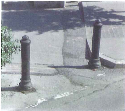
Existing bollards to be reused
