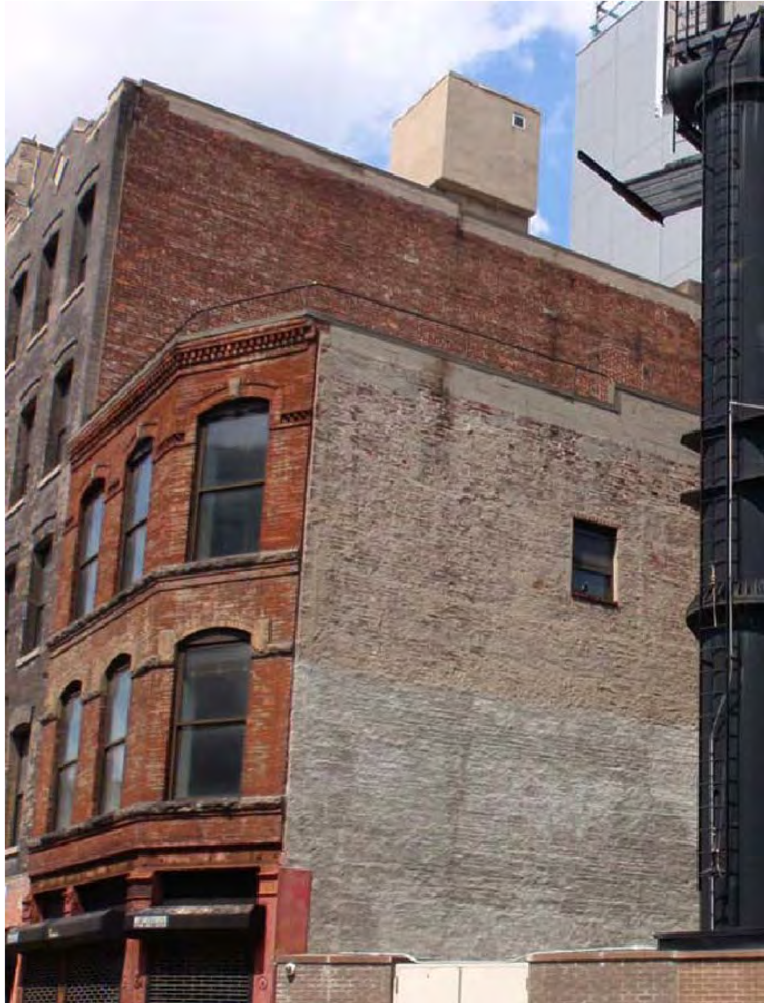
A VIEW OF EXISTING PARAPETS AT EAST ELEVATION
