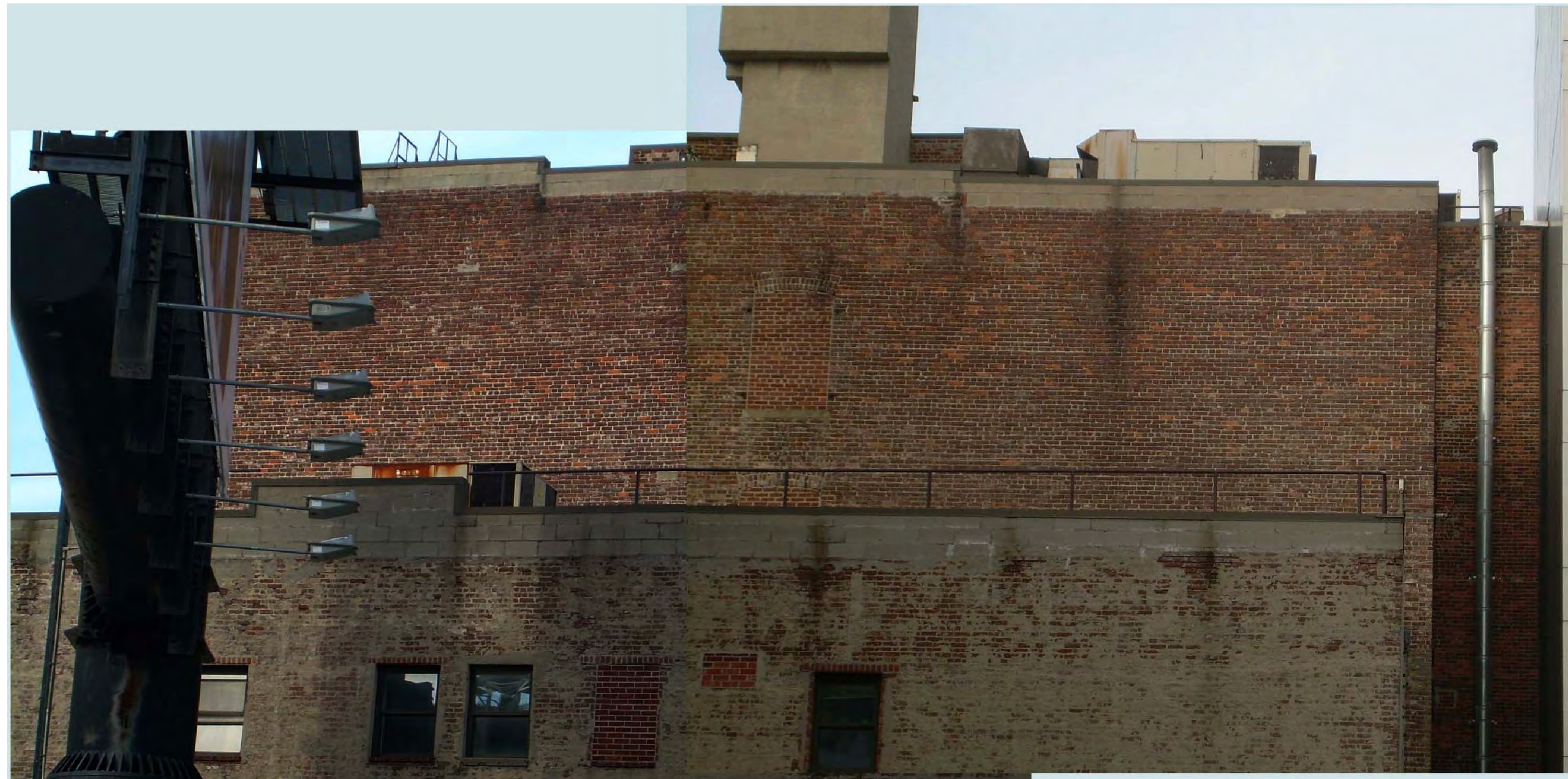
B VIEW OF EXISTING PARAPETS AT EAST ELEVATION
