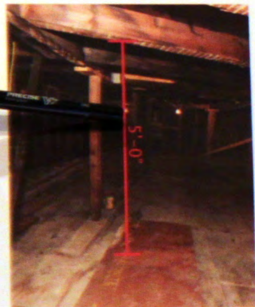
EXISTING CEILING JOISTS AT 5'-0"
