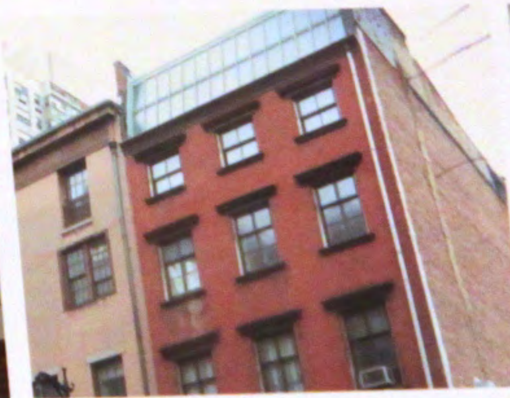
EXAMPLE AT 8 WEST 8TH STREET - NEW YORK STUDIO SCHOOL
