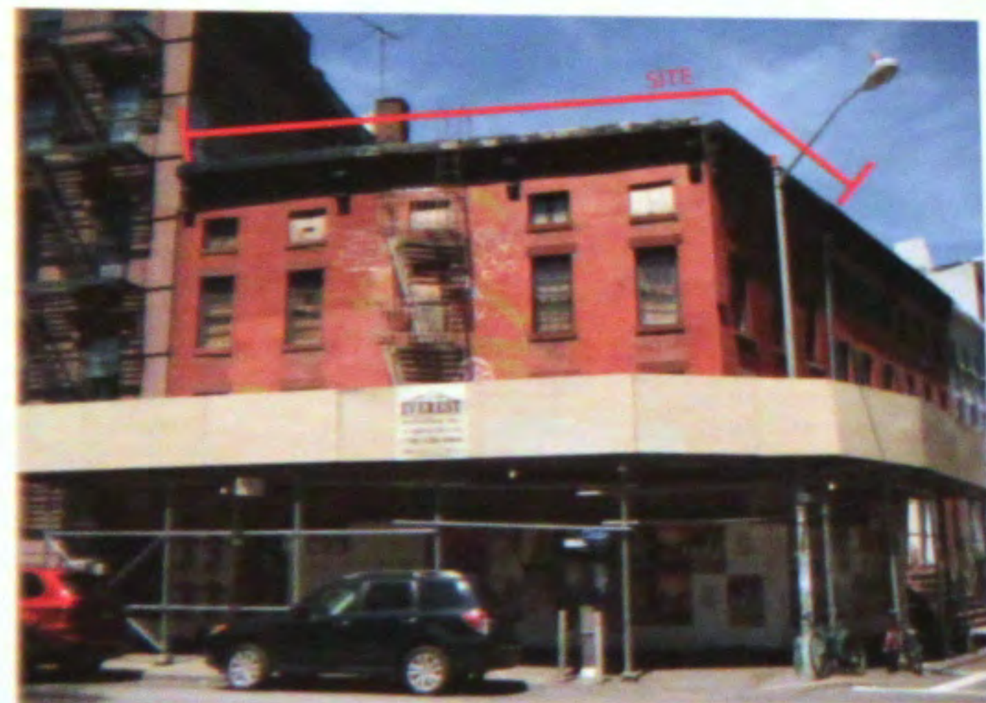
EXISTING CONDITION AT KING STREET
