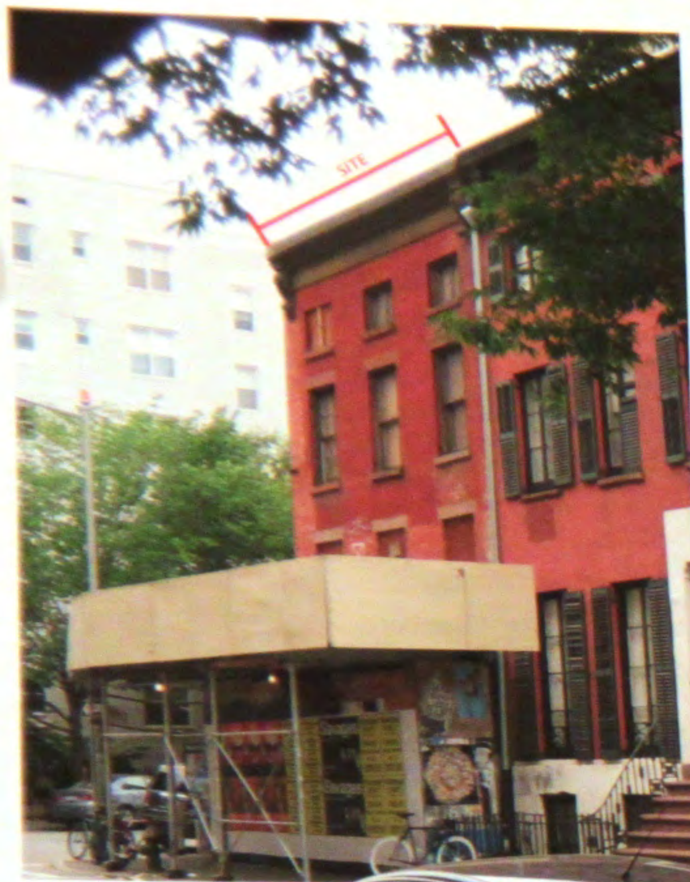
EXISTING CONDITION AT MACDOUGAL STREET
