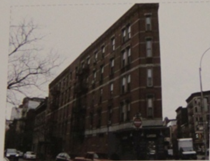
5 EXISTING CONDITIONS - NORTH ELEVATION
