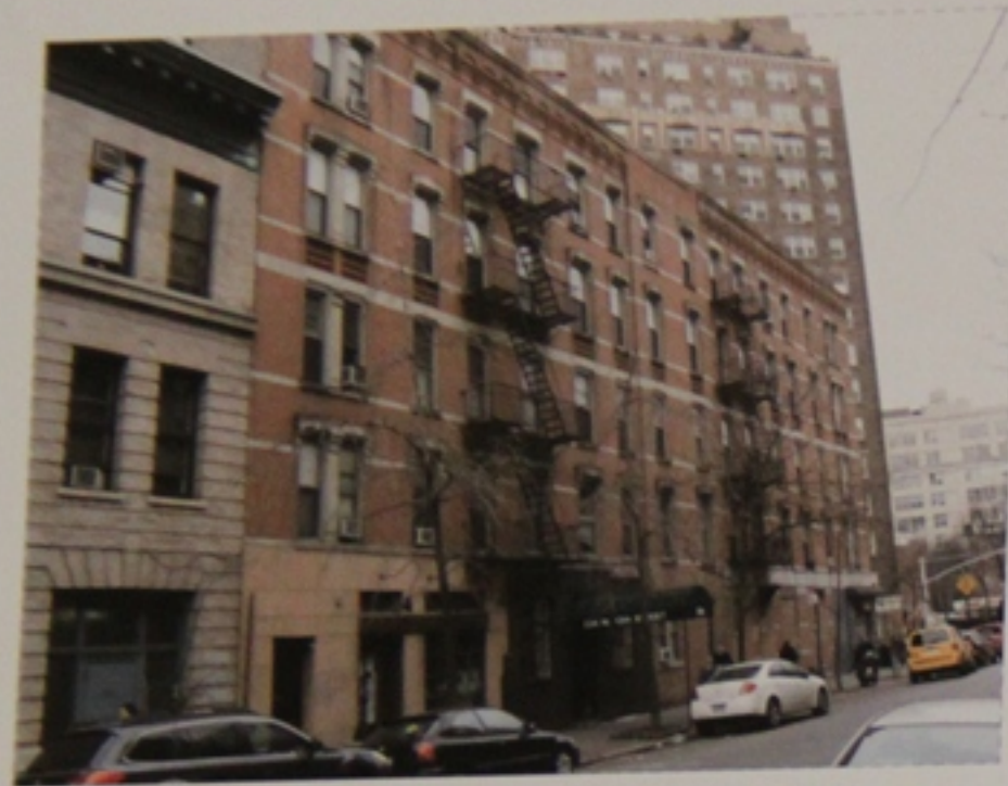
1 EXISTING CONDITIONS - NORTH ELEVATION
