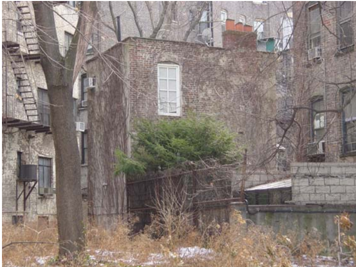
Figure 7. Rear building at 10 Bedford Street.
