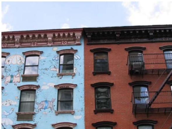
Figure 23. 498-500 LaGuardia Place, cornices.
