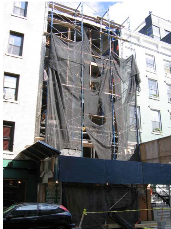
Figure 79. Former Sullivan Street Playhouse, 181 Sullivan Street, summer 2006.
