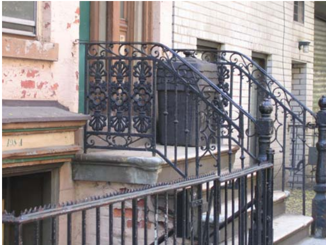
Figure 14. 198 Prince Street, ironwork.
