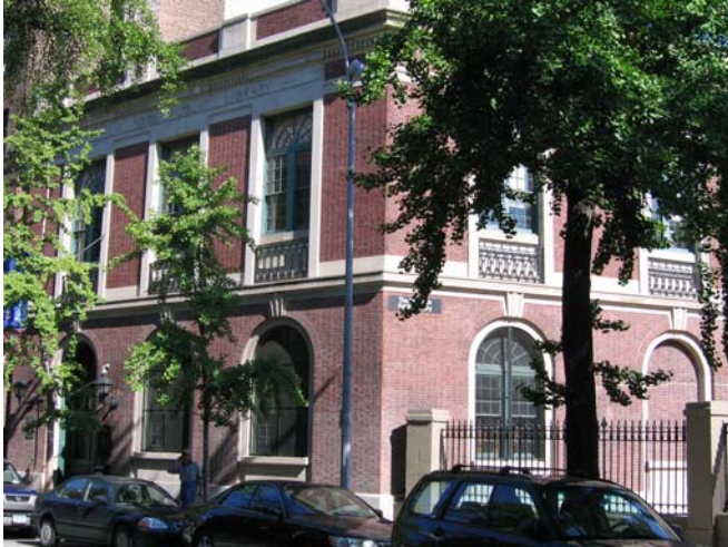
Figure 53. New York Public Library, Hudson Park Branch, 66 Leroy Street.
