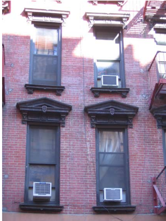
Figure 31. 39-43 Carmine Street, lintels.
