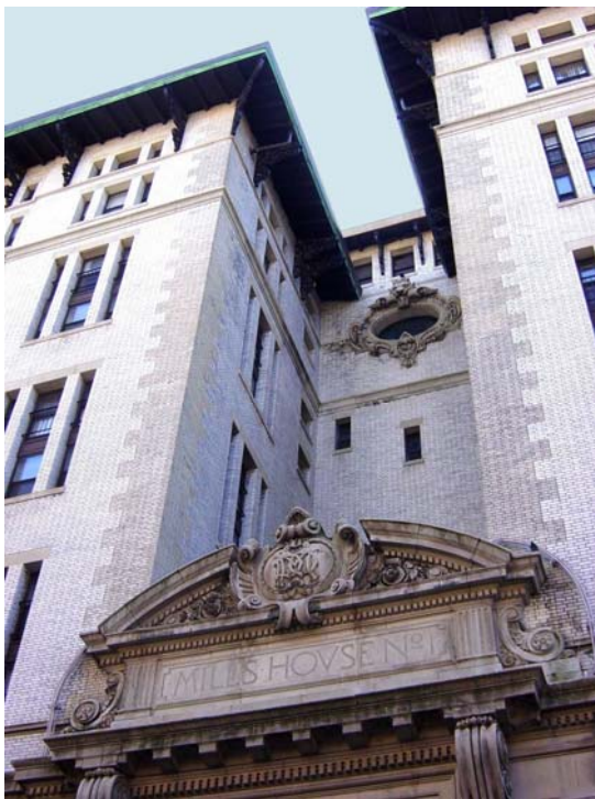
Figure 42. Mills House, 160 Bleeker Street.
