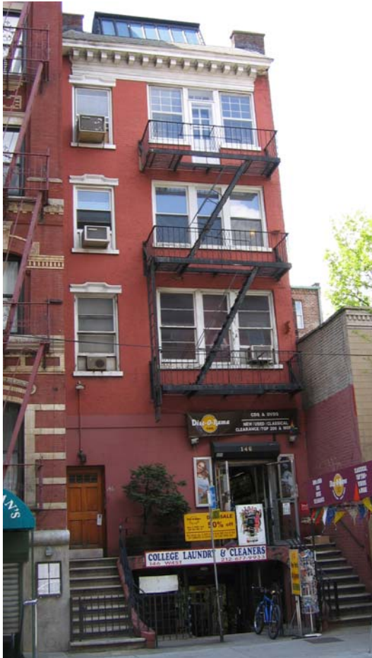
Figure 66. 146 West 4th Street.
