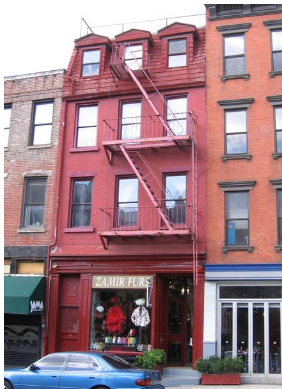
Figure 18. 90 West Houston Street.
