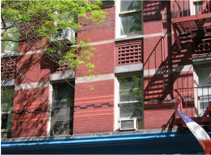
Figure 3. 36-38 MacDougal Street, brickwork.
