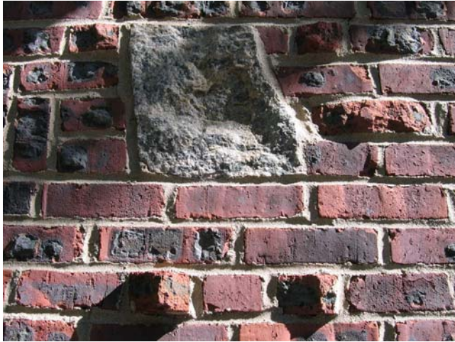
Figure 76. 62 Leroy Street, detail of brick and stone.
