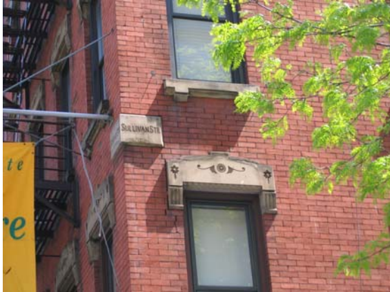
Figure 27. 200 Spring Street, lintels and street sign.
