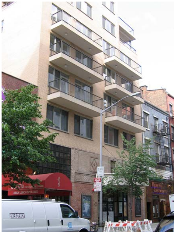
Figure 78. Former Circle in the Square Theater with Apartment Tower, 159 Bleecker Street.
