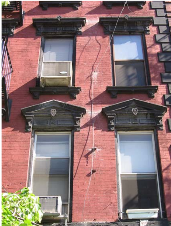
Figure 30. 143-145 Sullivan Street, lintels.
