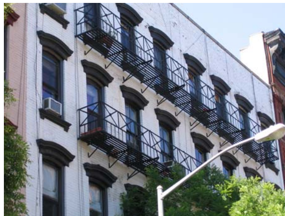
Figure 24. 25-29 Jones Street, fire balconies.
