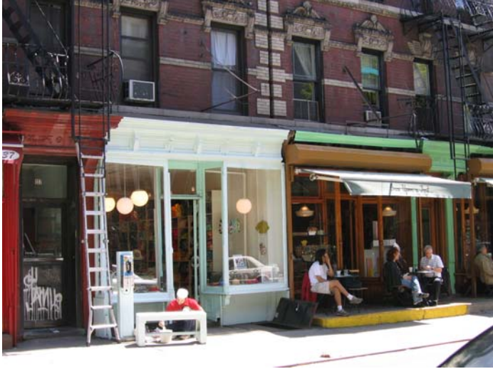
Figure 4. 135-137 Sullivan Street, storefronts.
