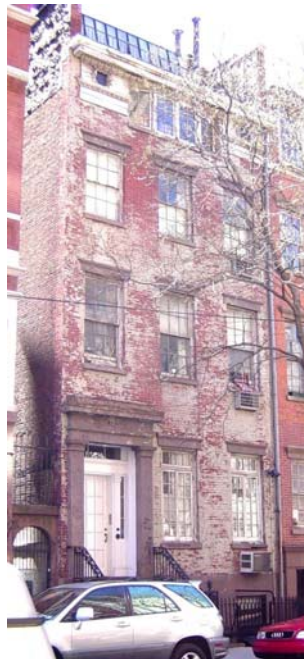
Figure 15. 132 West 4th Street.
