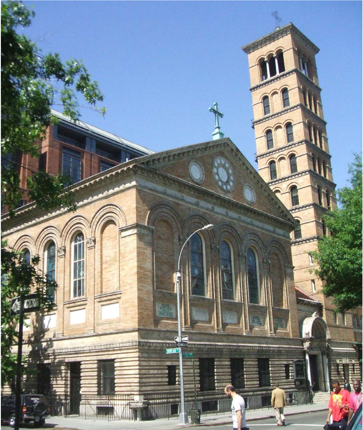
Figure 26. Judson Memorial Church, designed by McKim Mead and White and commissioned by Edward Judson and John D. Rockefeller, Sr., was a Baptist church that provided social services to the neighborhood's Italian immigrants in addition to its ministry.
