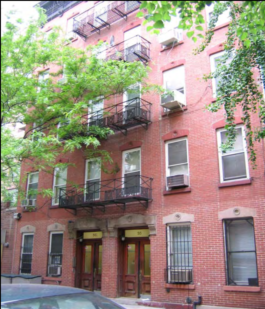
55 & 55-1/2 Downing St., architects Thom & Wilson, 1876
