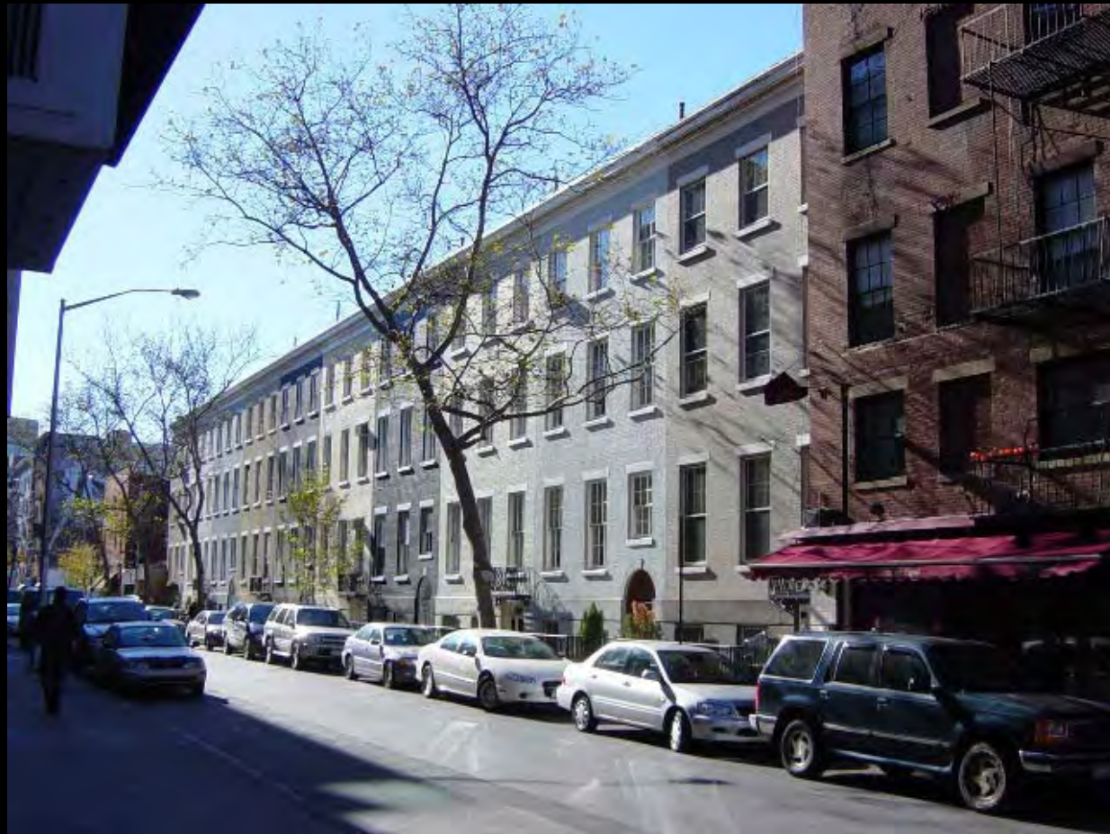
MacDougal Sullivan Gardens Historic District, altered 1917
