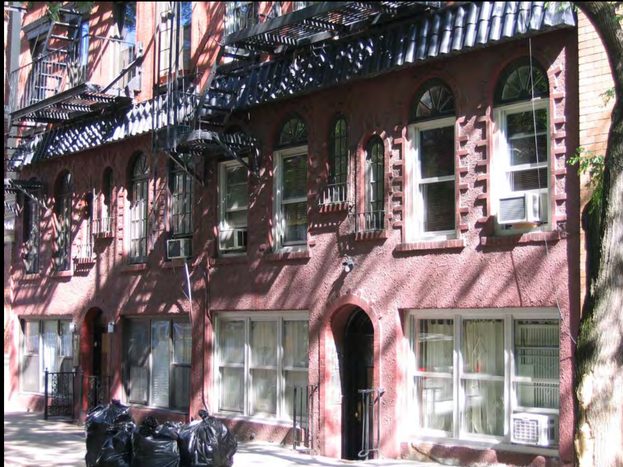
6-8 Jones Street, built 1871, altered 1929
