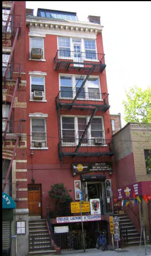
Greek Revival House at 146 West 4 th Street, altered 1916
