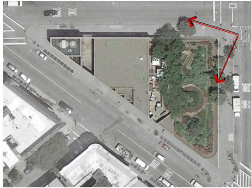
VIEW LOOKING SOUTH ON 7TH. AVENUE AND WEST 12TH. STREET'S CORNER
