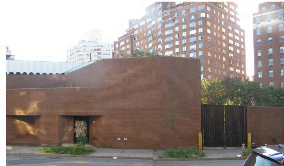
BEFORE VIEW FROM BANK STREET
