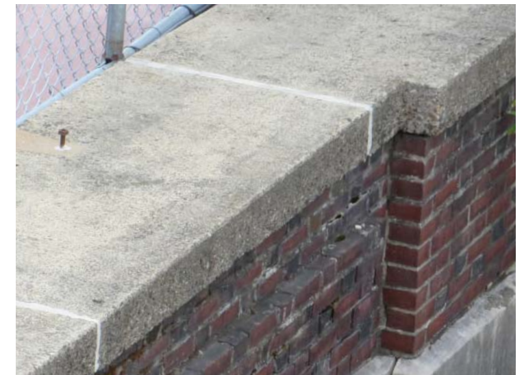
Existing Cast Stone Coping Stones:
