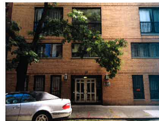
B3 EXISTING EXTERIOR FACADE PHOTO NTS
