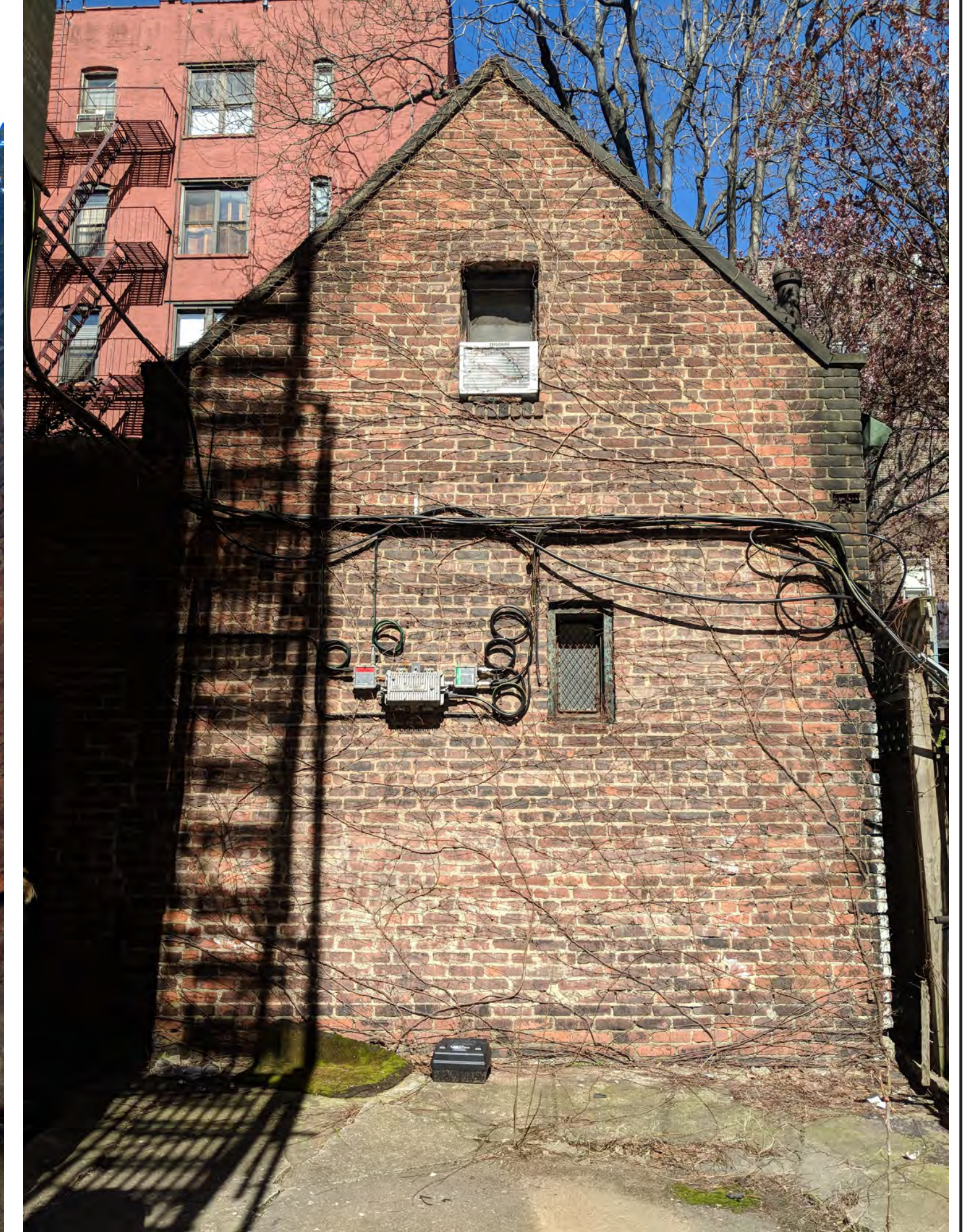
04 VIEW OF EAST FACADE OF STUDIO LOOKING NORTH
