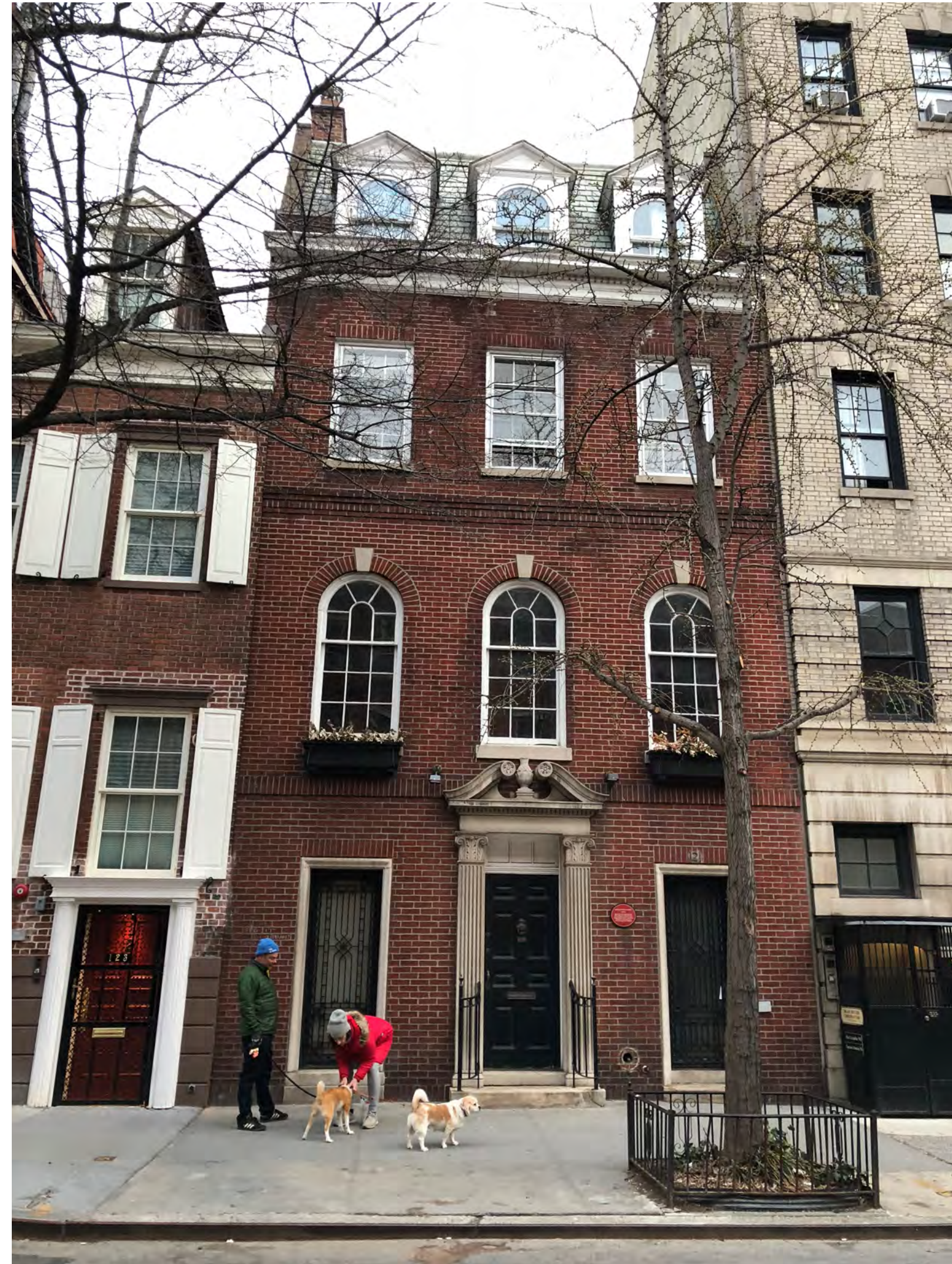
01 VIEW OF EXISTING FRONT FACADE
