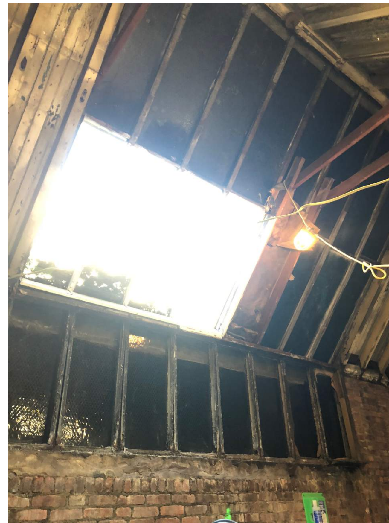
VIEW OF EXISTING SKYLIGHT OPENING AFTER INTERIOR DEMOLITION, REVEALING ORIGINAL SIZE
