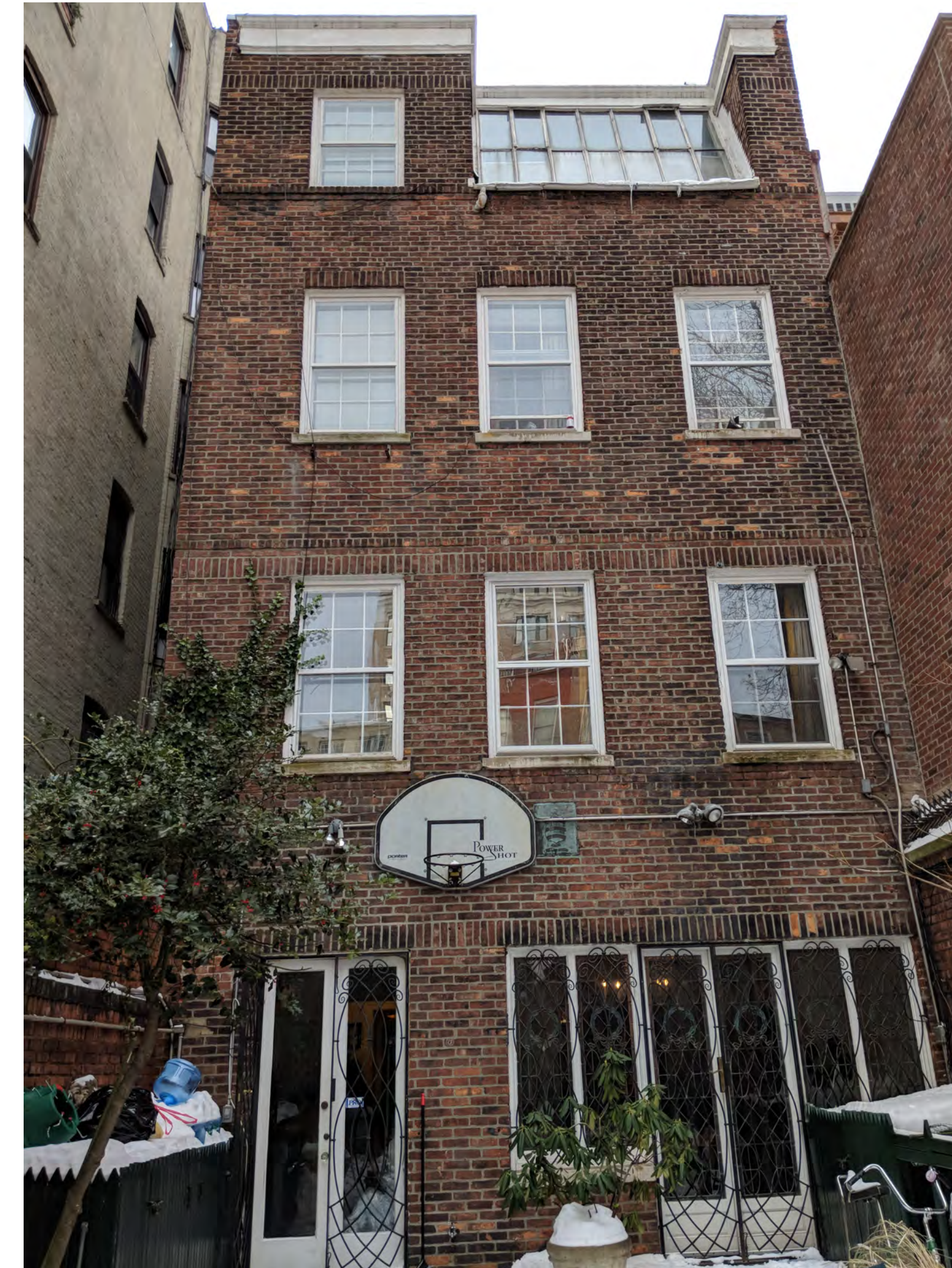
03 VIEW OF REAR FACADE
