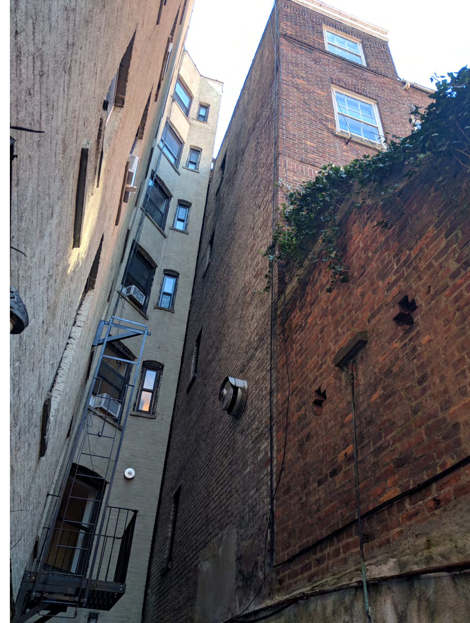
03 VIEW OF EAST FACADE OF 121 LOOKING NORTH
