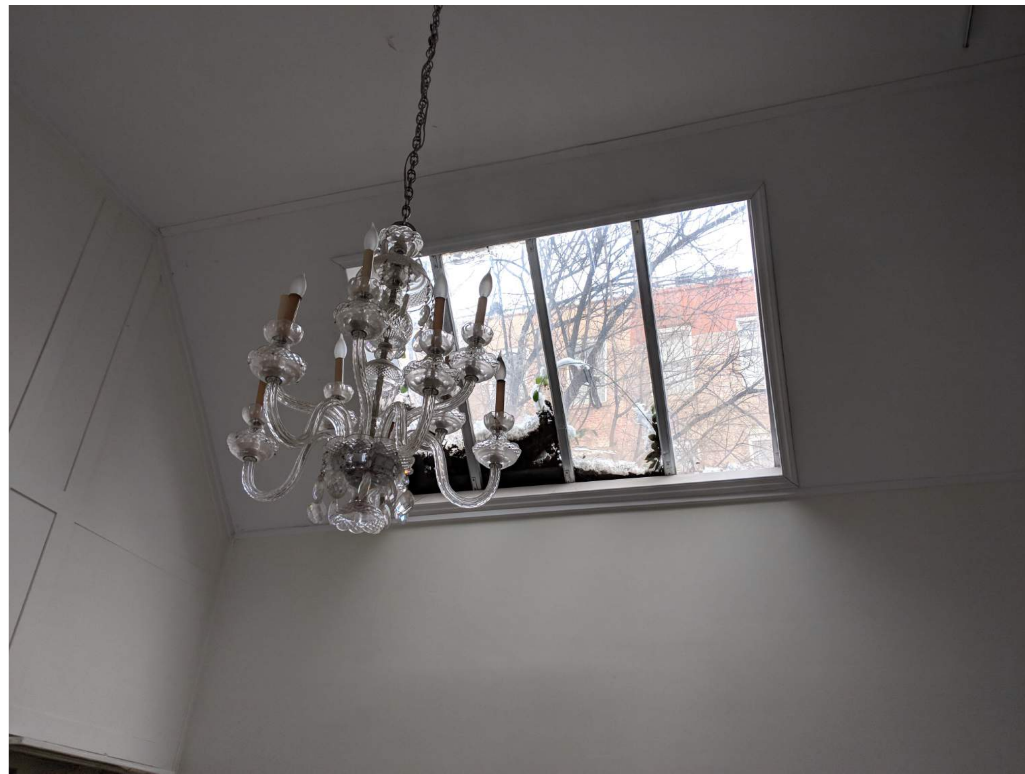
VIEW OF EXISTING SKYLIGHT OPENING BEFORE INTERIOR DEMOLITION
