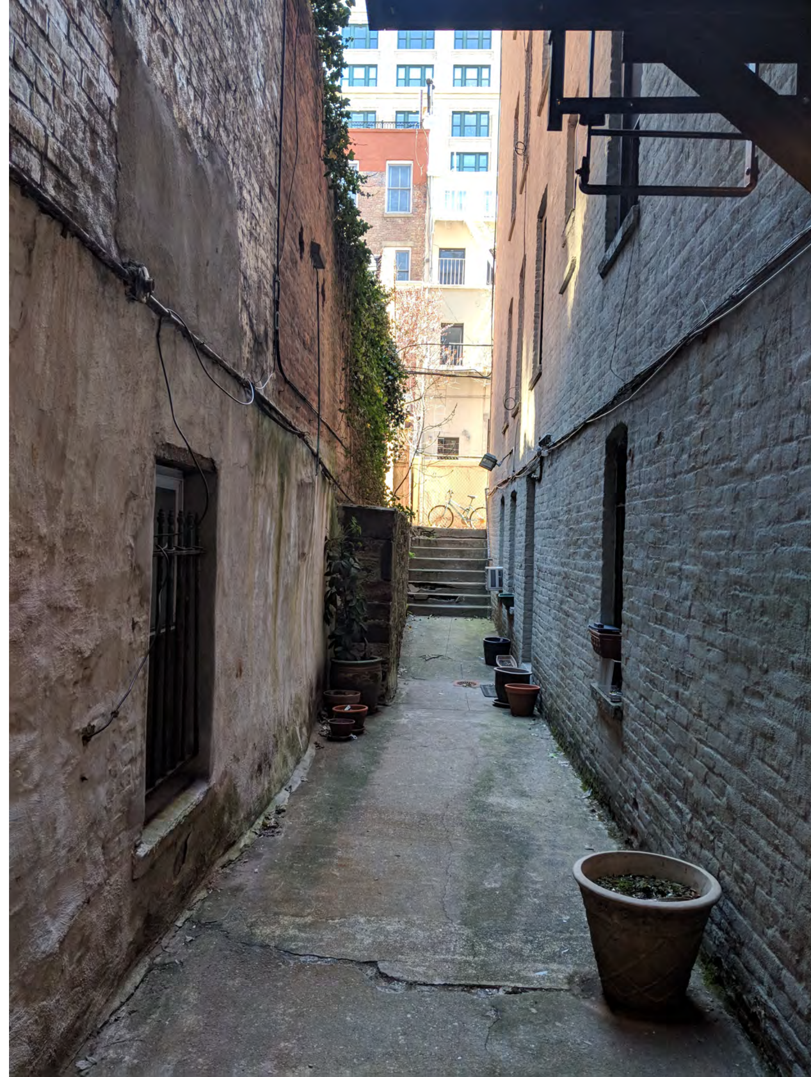
02 VIEW OF ALLEY LOOKING NORTH
