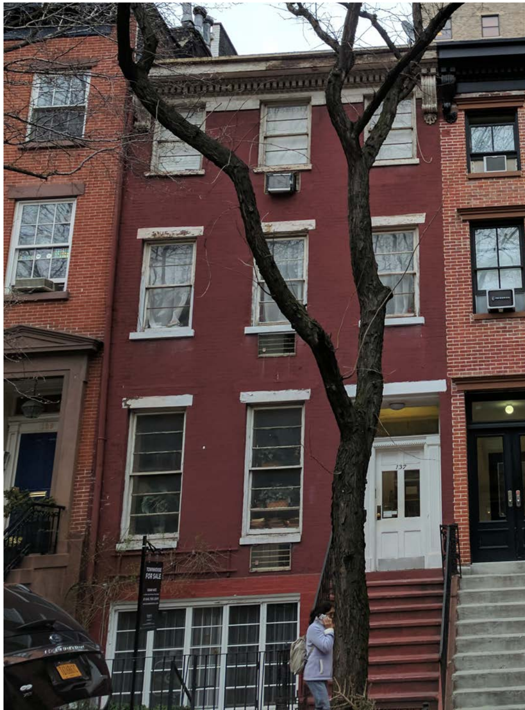
EXISTING FRONT FACADE
