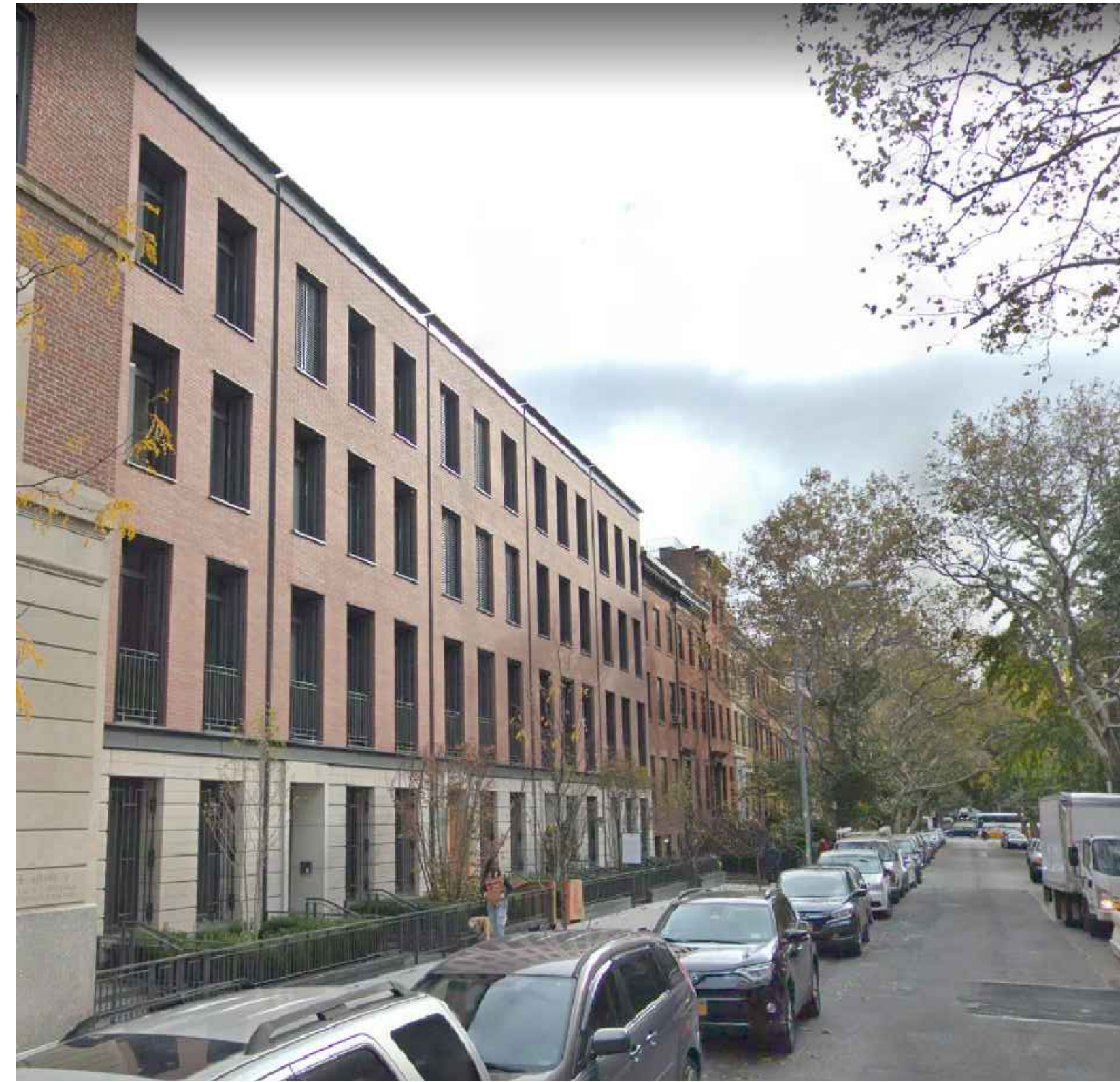
1 VIEW FROM SOUTHWEST: EXISTING
