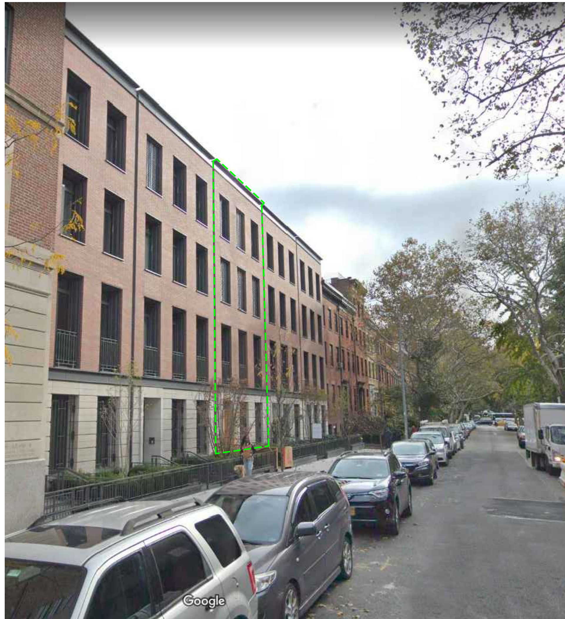
A VIEW FROM SOUTHWEST
