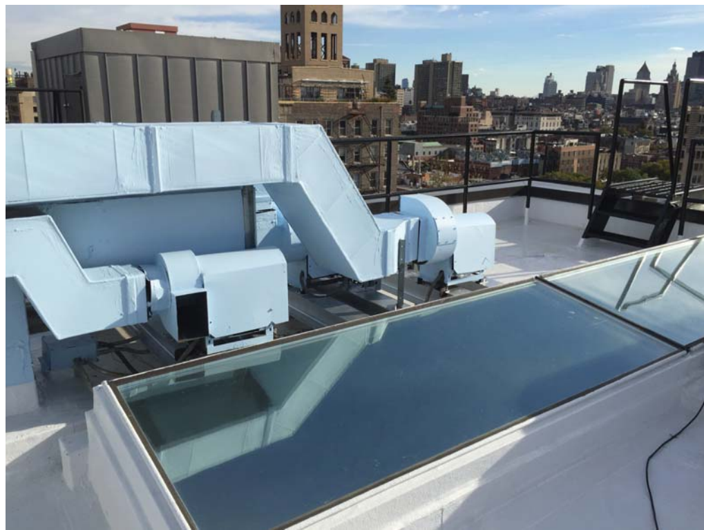
SKYLIGHT ON PENTHOUSE ROOF LOOKING SOUTH
