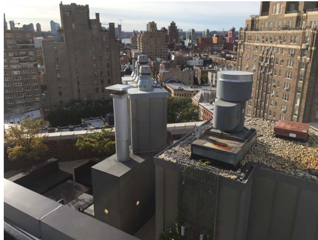
PENTHOUSE ROOF LOOKING WEST
