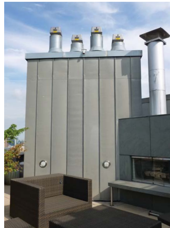
EXISTING SOUTH TERRACE VIEW PENTHOUSE FLOOR LOOKING WEST
