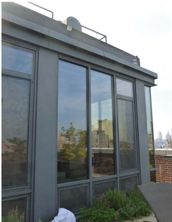
EXISTING SOUTH TERRACE VIEW PENTHOUSE FLOOR LOOKING SOUTH
