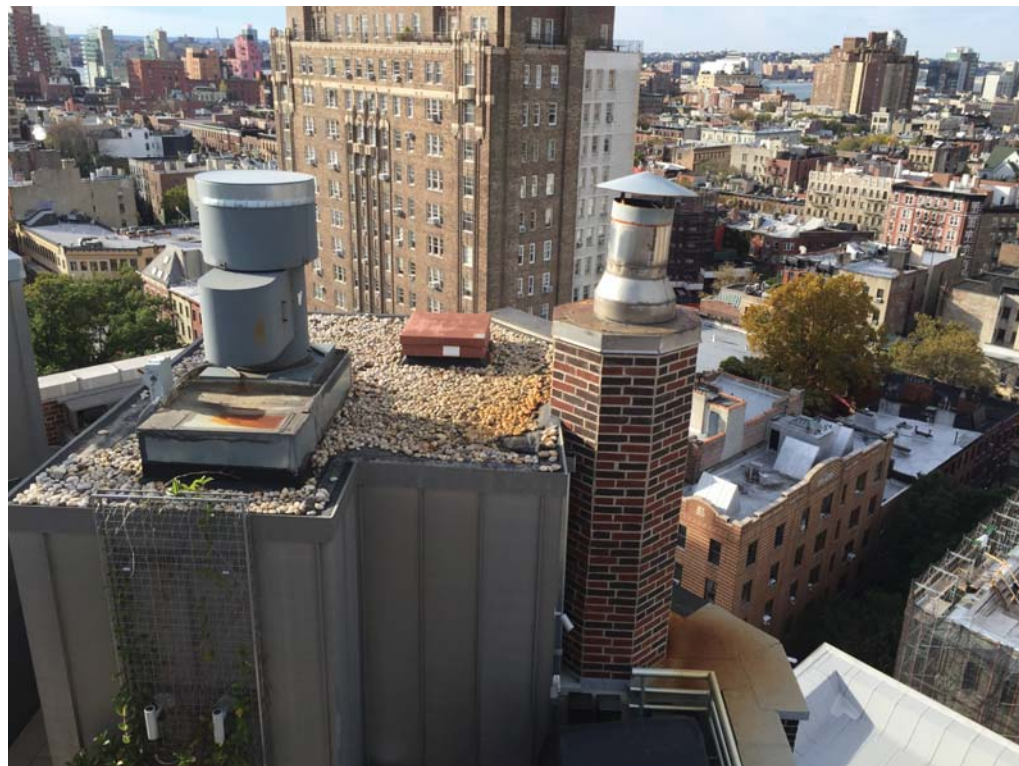
PENTHOUSE ROOF LOOKING NORTHWEST
