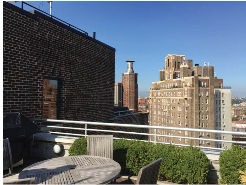
EXISTING NORTH TERRACE VIEW PENTHOUSE FLOOR LOOKING WEST
