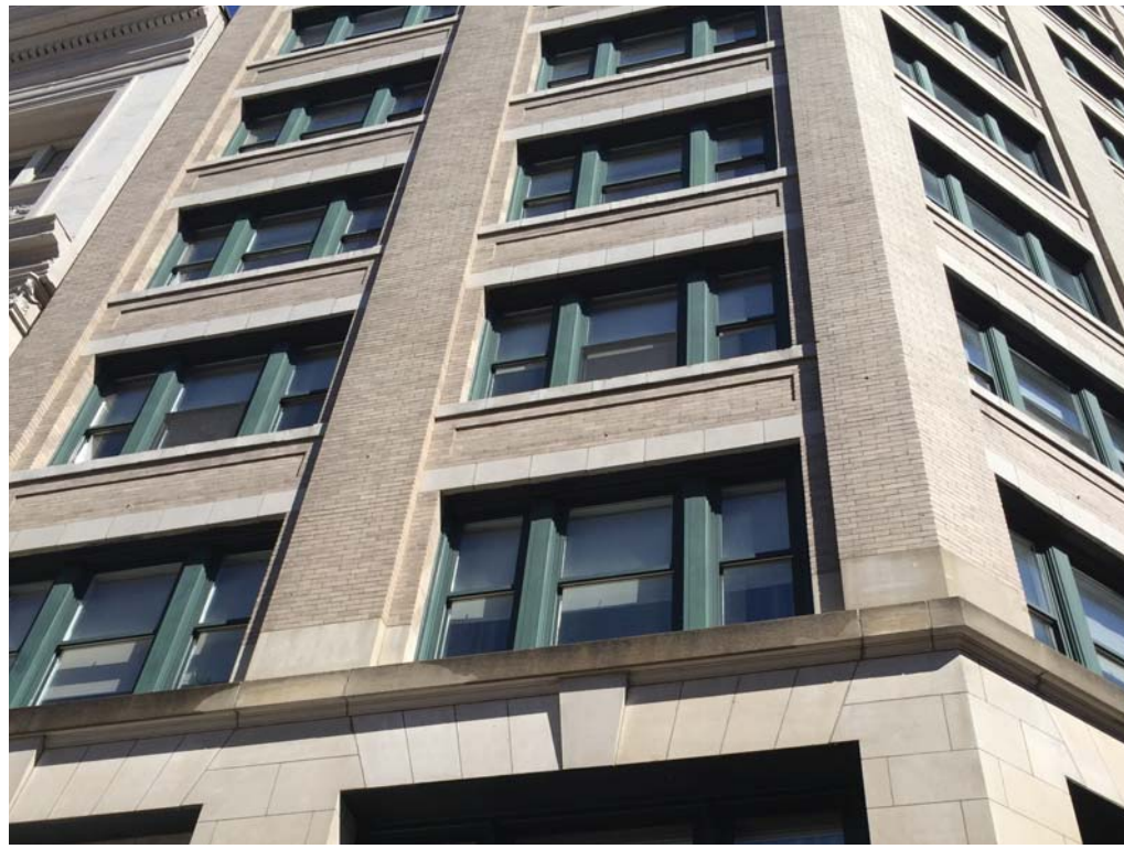
EXISTING WINDOWS ON SOUTH FACADE
