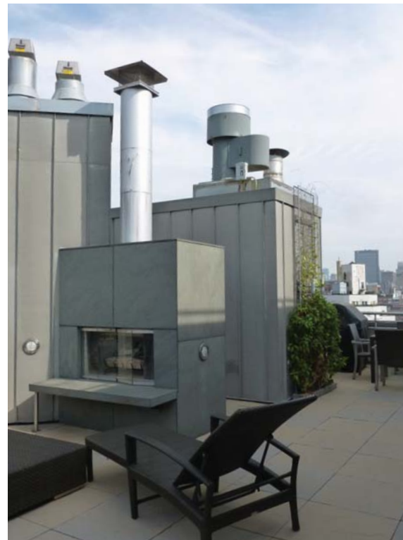
EXISTING SOUTH TERRACE VIEW PENTHOUSE FLOOR LOOKING NORTHWEST
