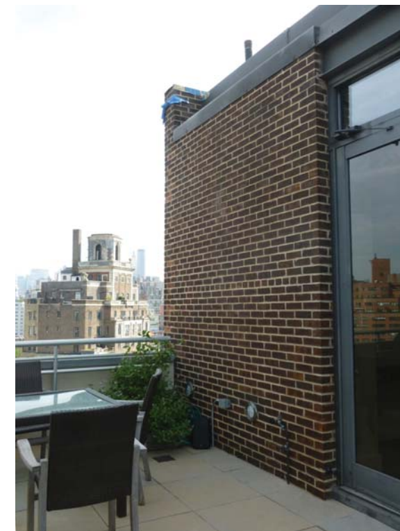
EXISTING SOUTH TERRACE VIEW PENTHOUSE FLOOR LOOKING NORTHEAST
