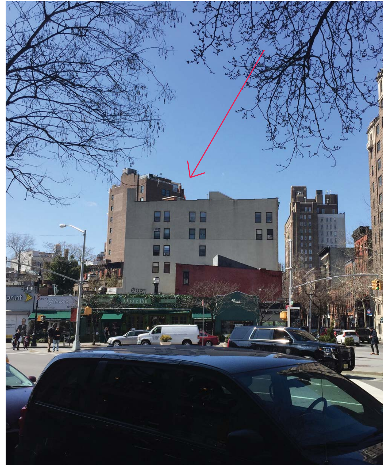
RENDERING OF PROPOSED VIEW FROM THE CORNER OF 6TH AVENUE AND WEST 9TH STREET
