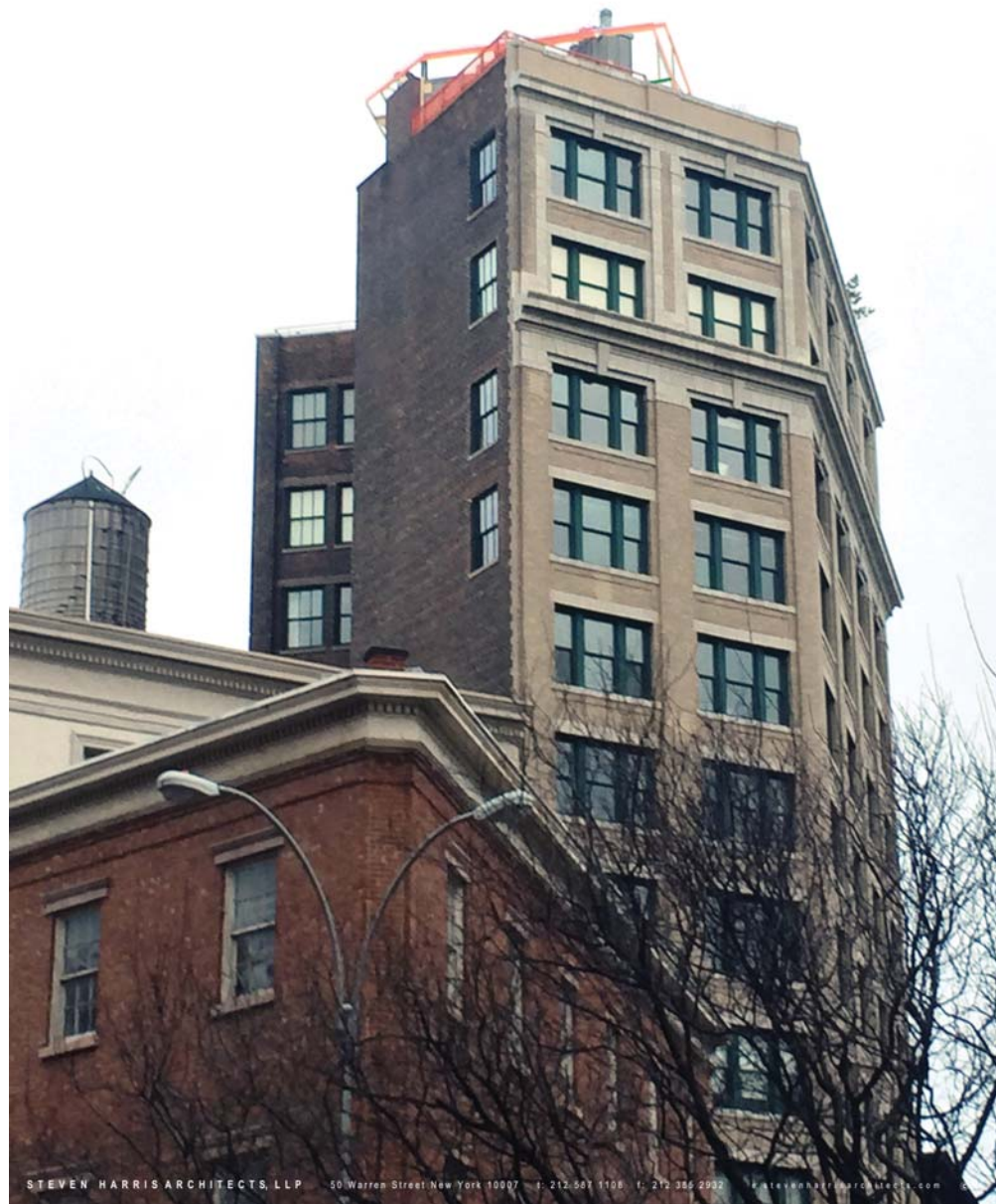
EXISTING CONDITION - VIEW FROM CHRISTOPHER STREET AND GROVE STREET
