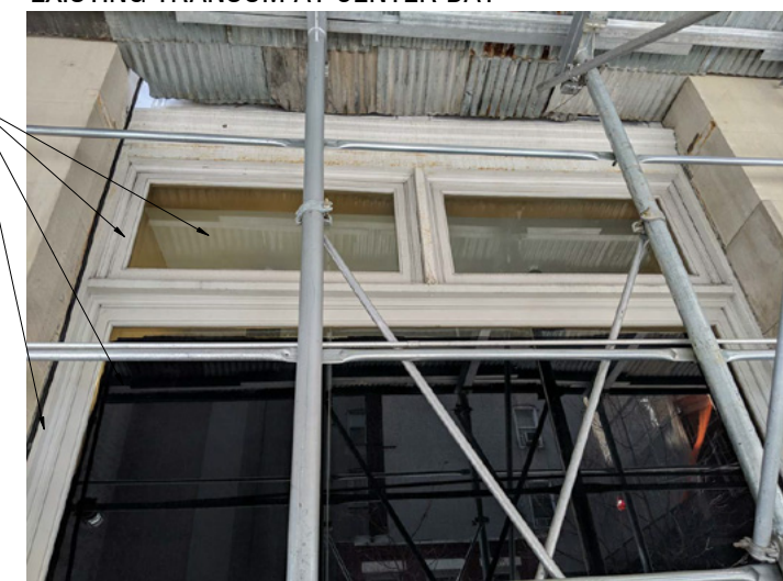
EXISTING TRANSOM AT CENTER BAY
