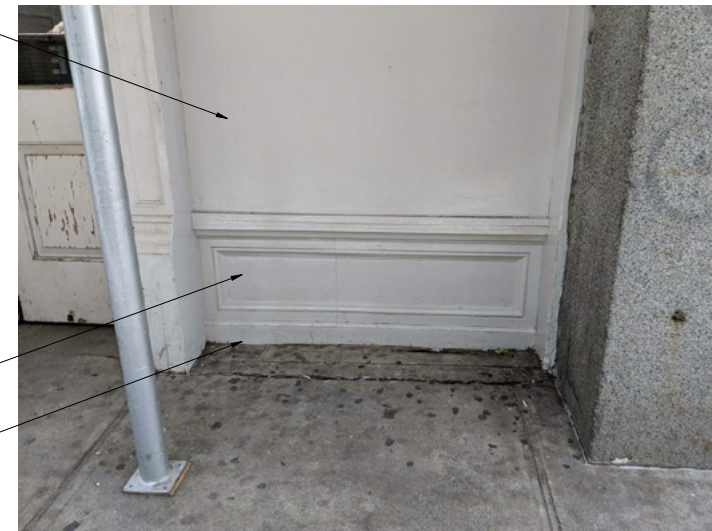
EXISTING STOREFRONT SILLS
