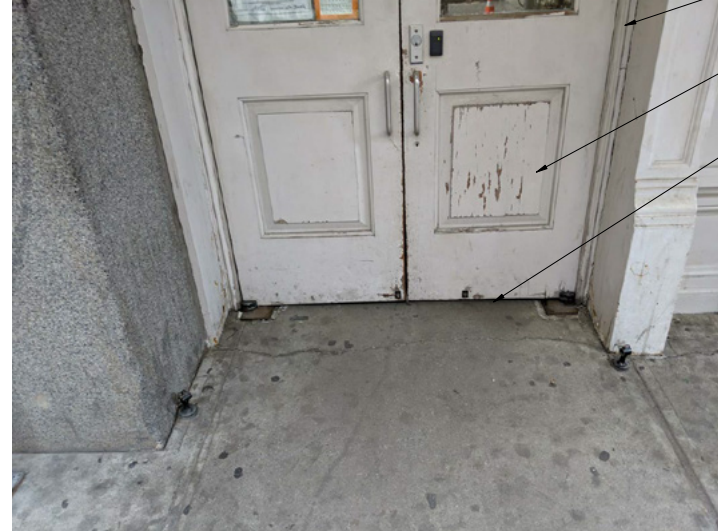
EXISTING DOOR SILL CONDITION
