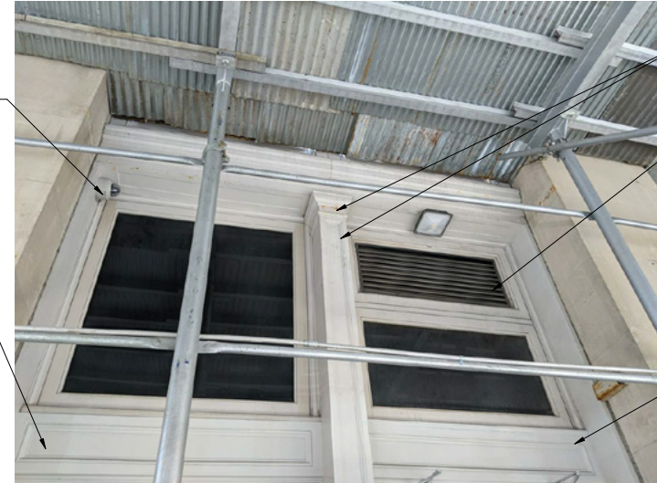
EXISTING TRANSOM PANELS AT LEFT BAY
