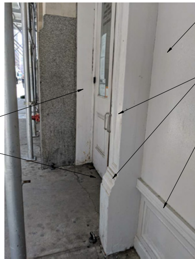
EXISTING STOREFRONT COLUMN
