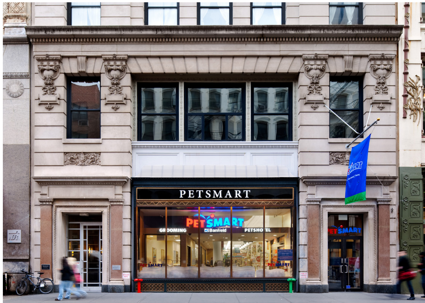
FRONT FACADE 632 BROADWAY
