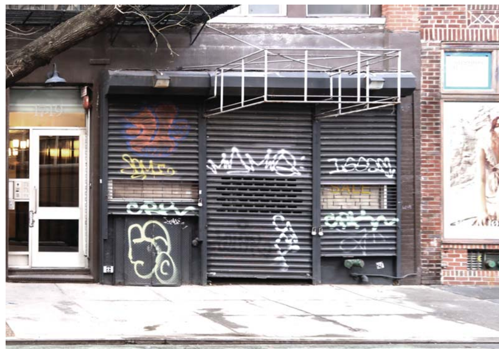
3 - 17 BLEECKER STREET - BEFORE (APRIL 2017)
