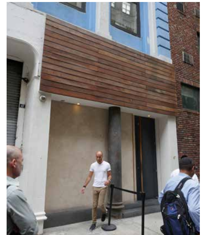
EAST 12TH STREET FACADE & STOREFRONT
