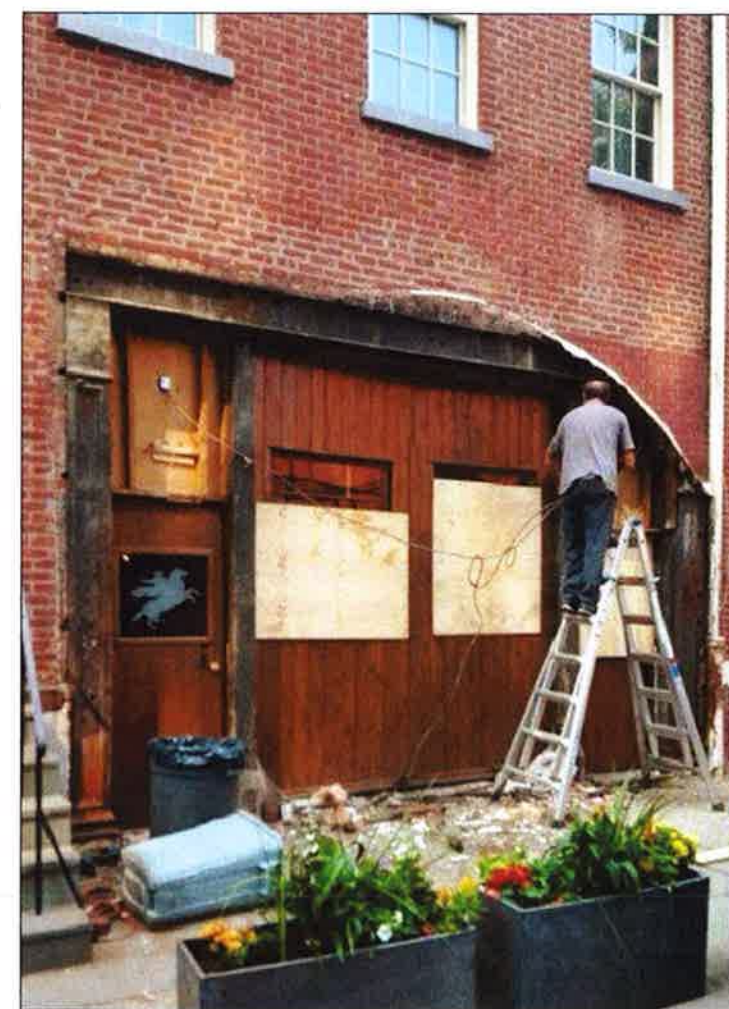
Removal of the pre-existing arch
