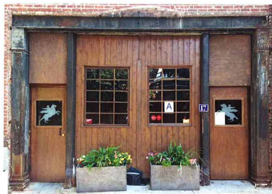
Storefront facade View
