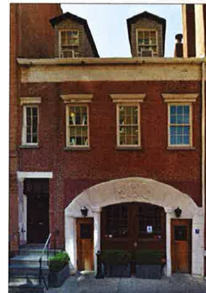
Building facade view prior the last renovation
