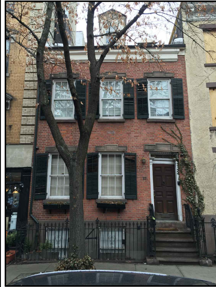
A EXISTING CONDITION
