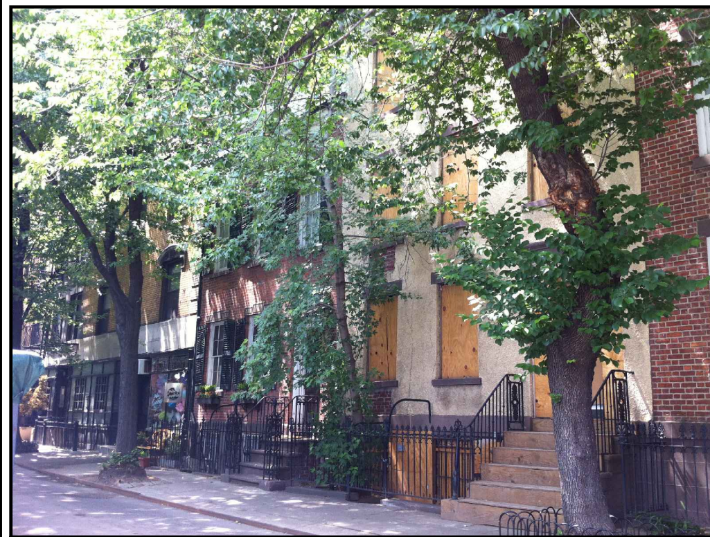
C EXISTING CONDITION
