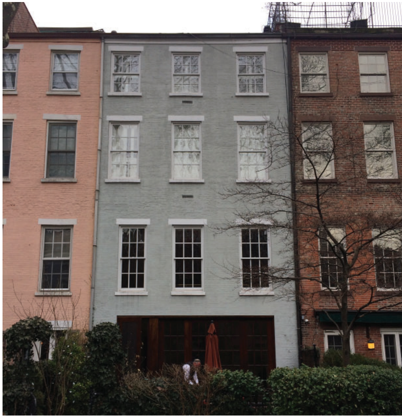
186 Sullivan Street - Existing Rear Facade
