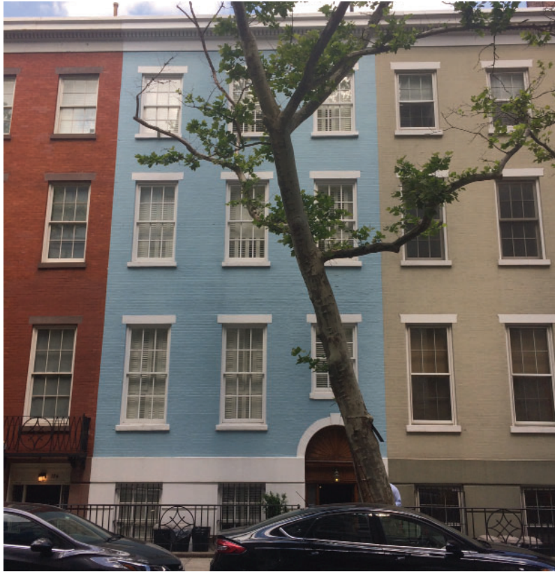
186 Sullivan Street - Existing Street Facade
