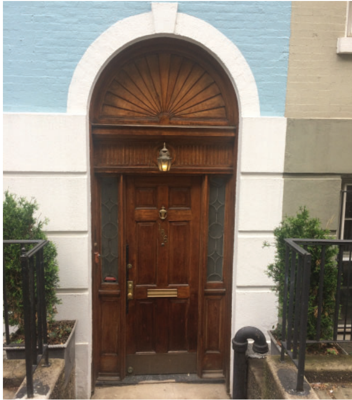
186 Sullivan Street - Existing Front Door Assembly
