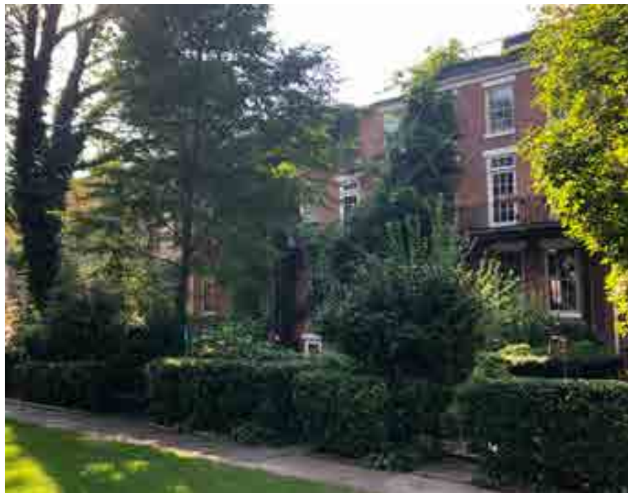
Garden Facing Southwest
