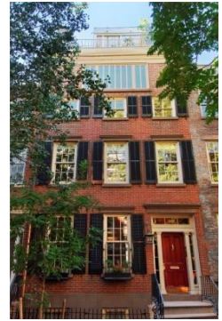
280 WEST 4TH STREET GOOGLE STREET VIEW
