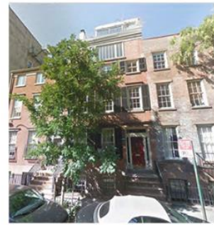
280 WEST 4TH STREET GOOGLE STREET VIEW
