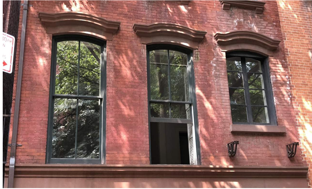
1. EXISTING PARLOR WINDOWS AT FRONT FACADE
