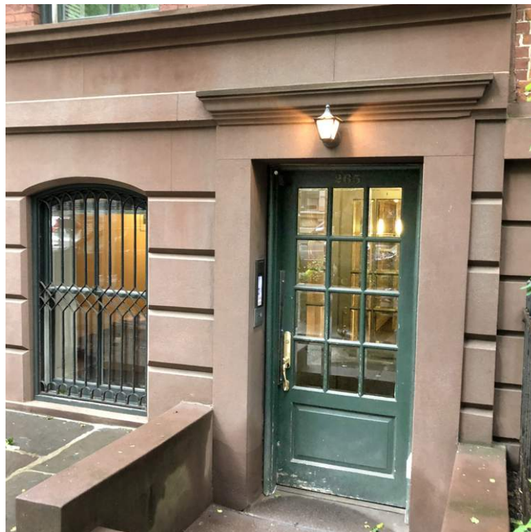
1. EXISTING FRONT DOOR AND DECORATIVE SURROUND
