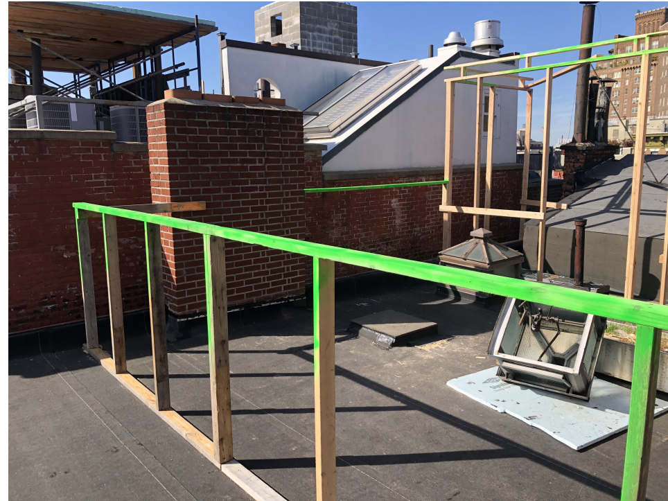
2. PHOTO OF PROPOSED BULKHEAD MOCKUP
