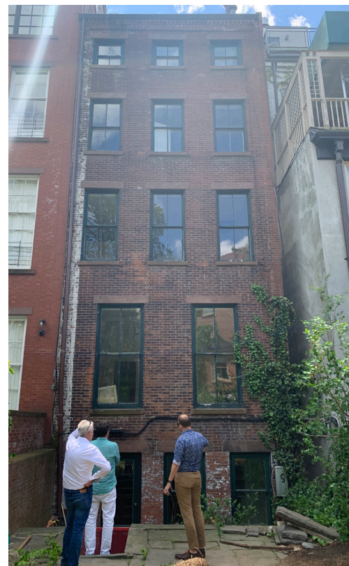
265 WEST 11TH STREET, CURRENT REAR FACADE
