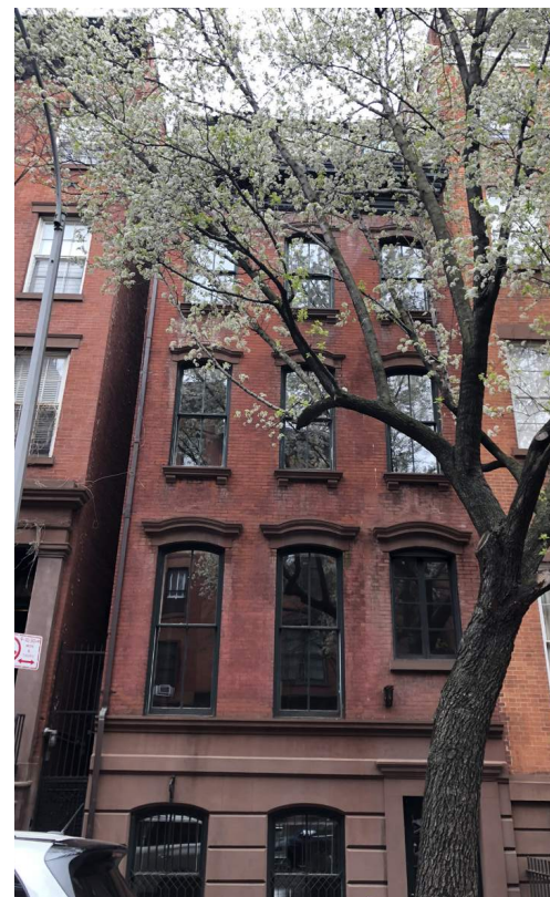
265 WEST 11TH STREET, CURRENT STREET FACADE
