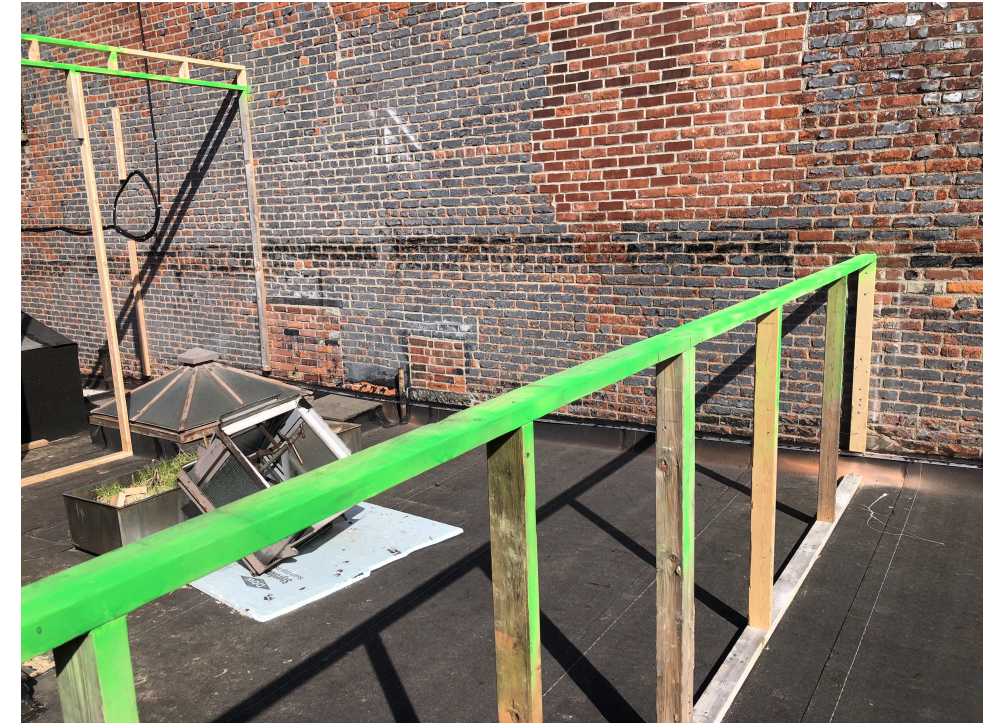
3. PHOTO OF PROPOSED BULKHEAD MOCKUP
