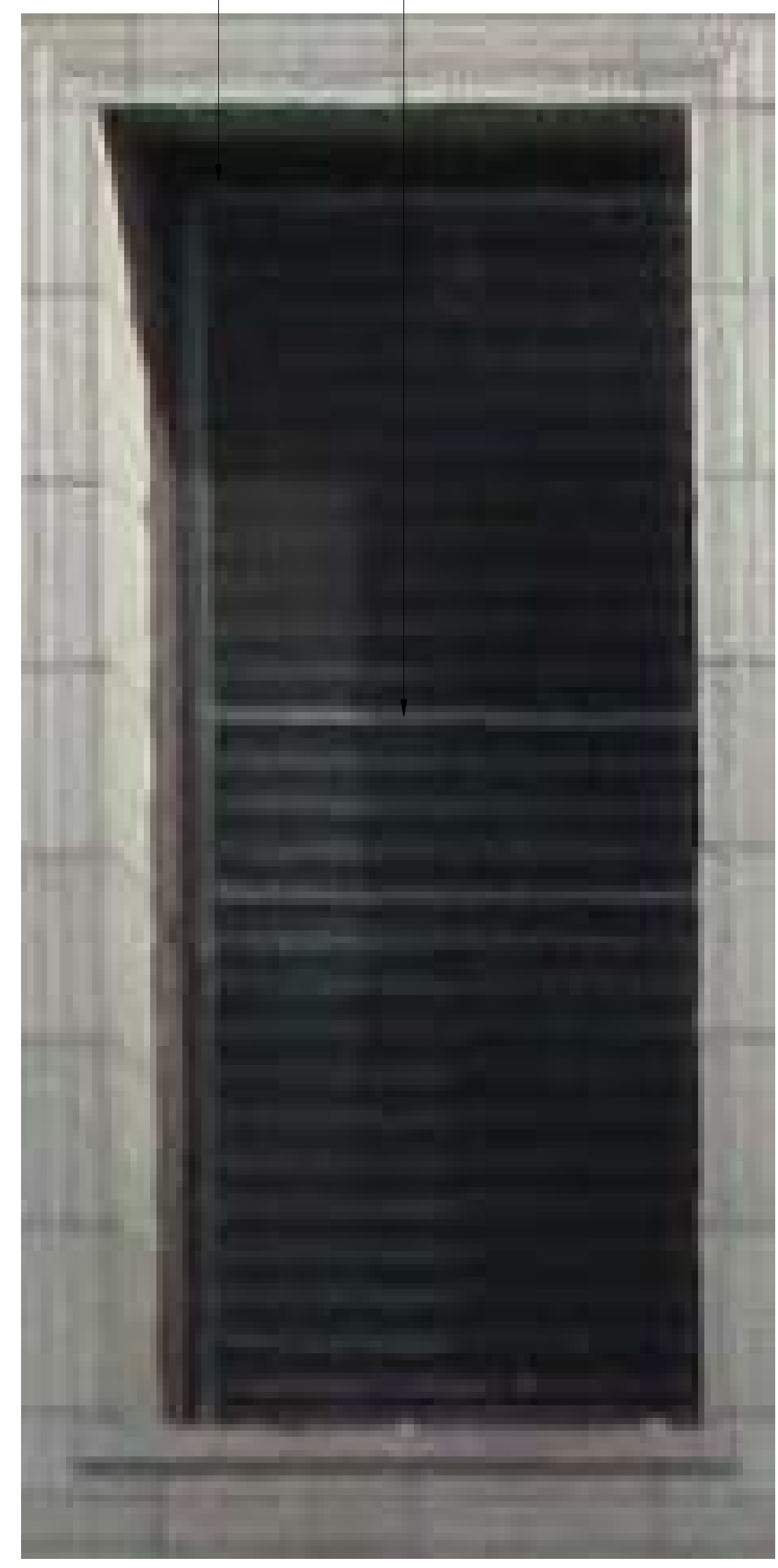
1 11TH FLOOR - TYP. EXISTING GLASS WINDOW AND GLASS TRANSOM.
