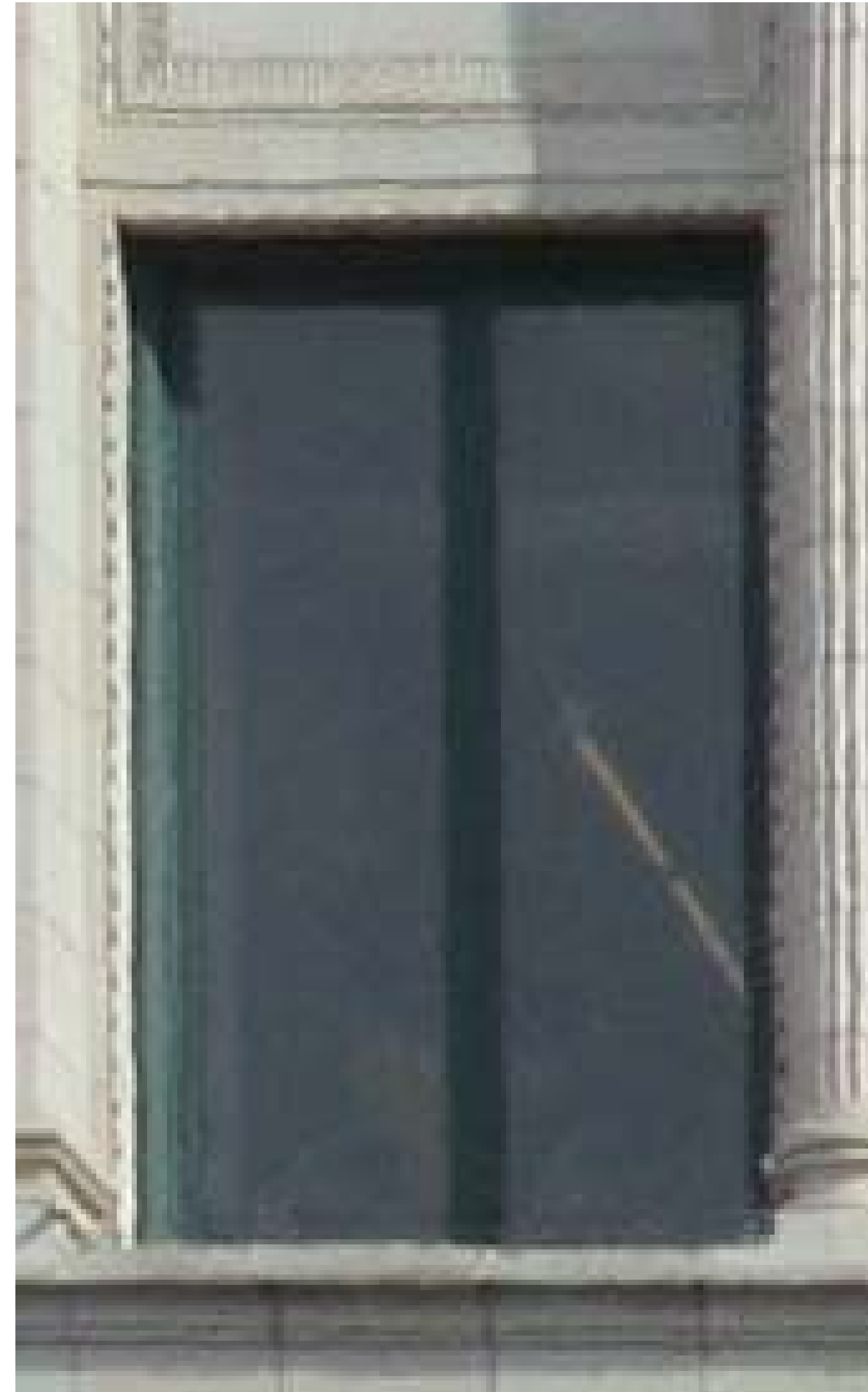
5 13TH FLOOR- EXISTING GLASS WINDOW
