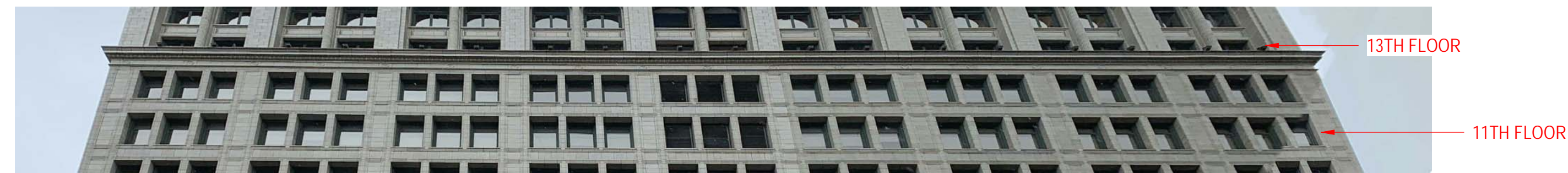
STREET VIEW- EXISTING WEST ELEVATION( PARTIAL)
