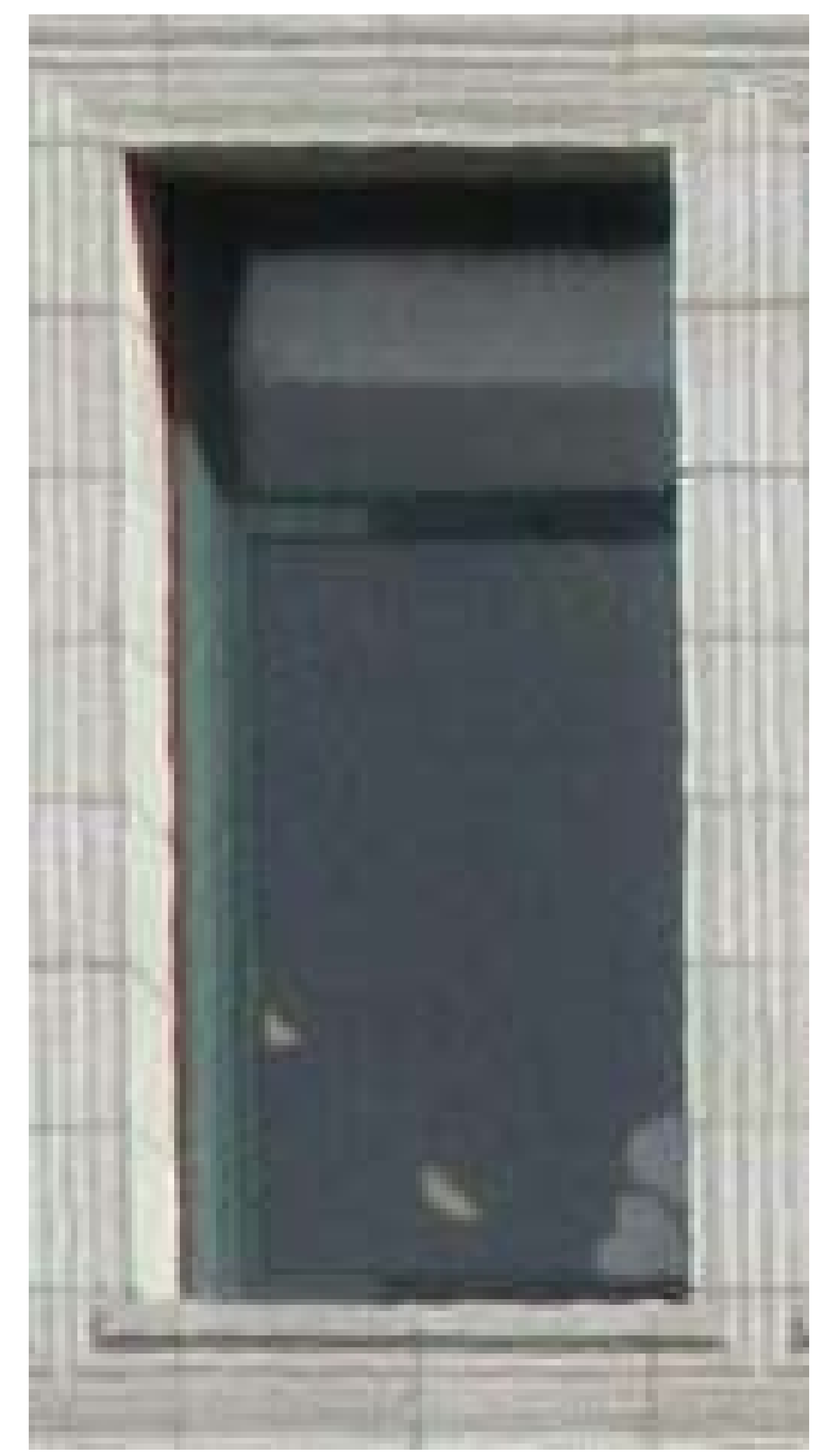
2 11TH FLOOR - TYP. EXISTING GLASS WINDOW AND GLASS TRANSOM.
