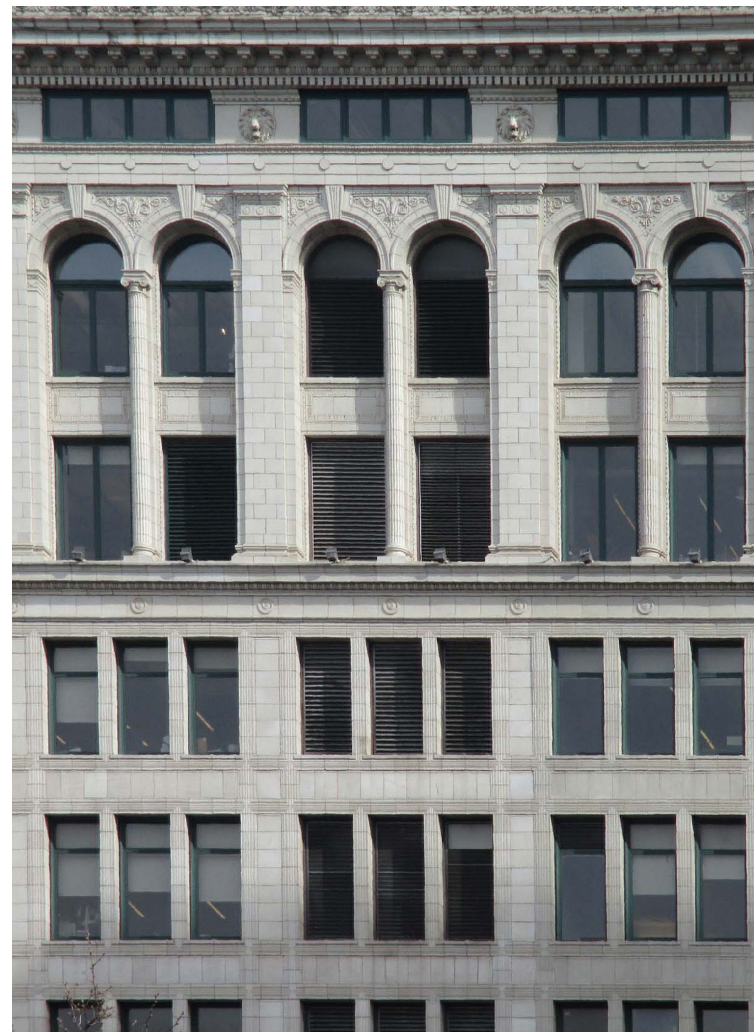
CLOSE UP - WEST FACADE
