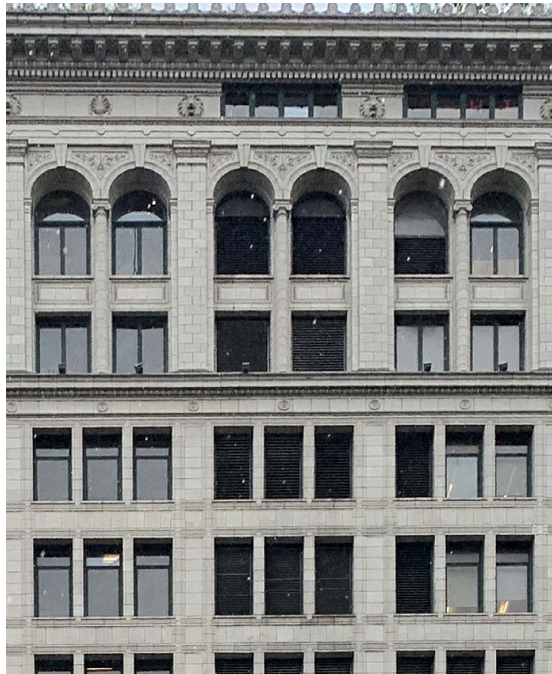
CLOSE UP - EAST FACADE
