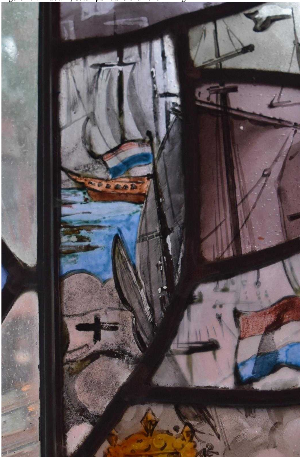
Figure 4: Window 1, detail paint and enamel crizzling
