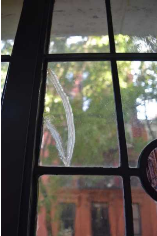
Figure 15: Window 5, detail, broken glass, plaster and frame damage
