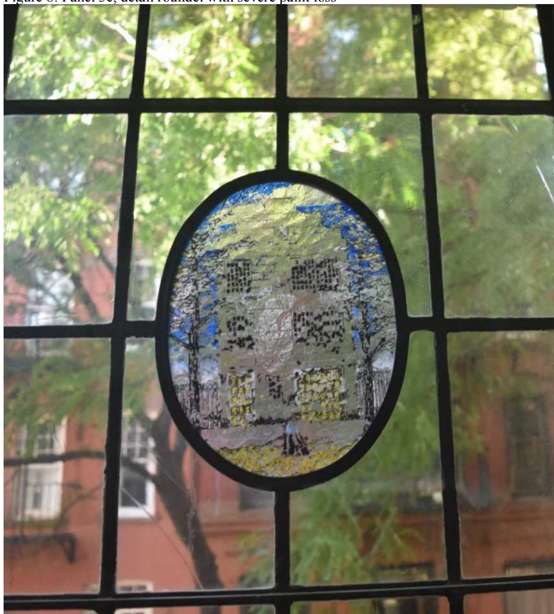
Figure 8: Panel 3c, detail roundel with severe paint loss
