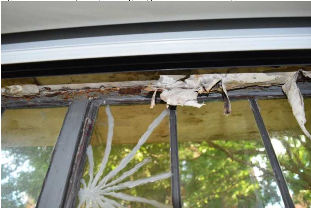
Figure 15: Window 5, detail, broken glass, plaster and frame damage
