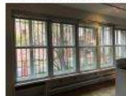
EXISTING FIRST FLOOR NORTH WINDOWS ①
