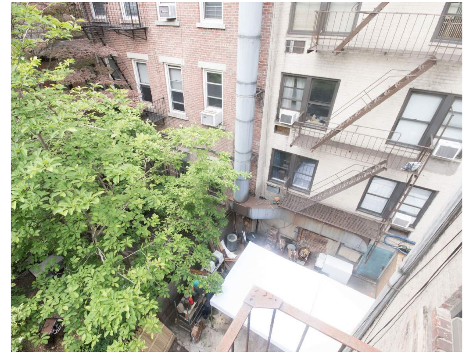
3- VIEW OF SIDE YARD, FROM ROOF OF 200 PRINCE ST.
