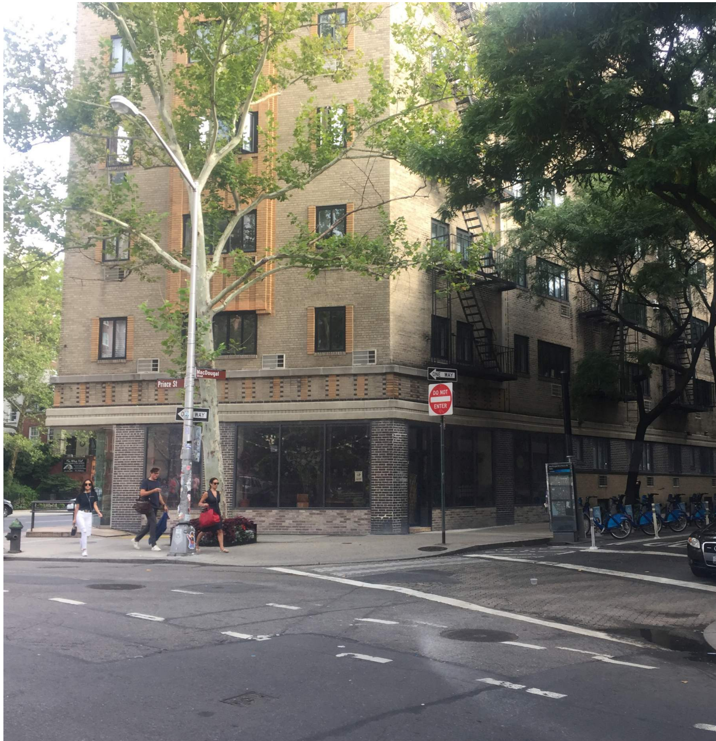
210 AVE. OF THE AMERICAS- VIEW FROM PRINCE STREET, ACROSS THE PROJECT'S SITE
