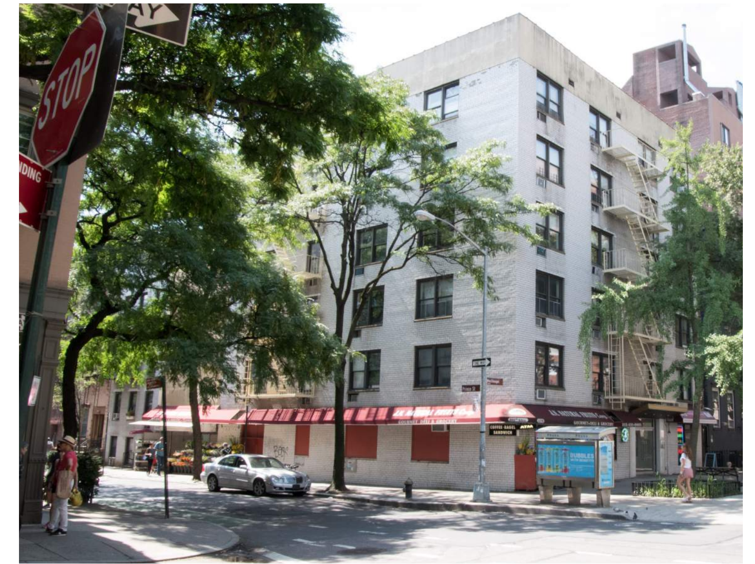
3- VIEW FROM CORNER OF MACDOUGAL ST AND PRINCE ST
