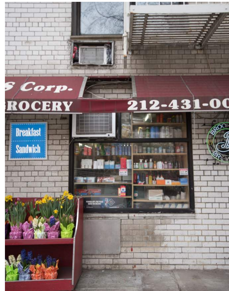
3- ALUMINUM FRAME WINDOW AT GROUND FLOOR FACING THE PARK
