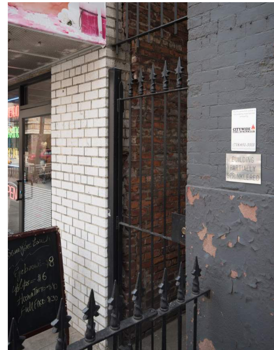
4 THROUGH 8- CORNER DETAIL ACROSS 198 6TH AVE. DETAIL OF ORIGINAL BRICK WALL WITH LATER ADDED WHITE BRICK
