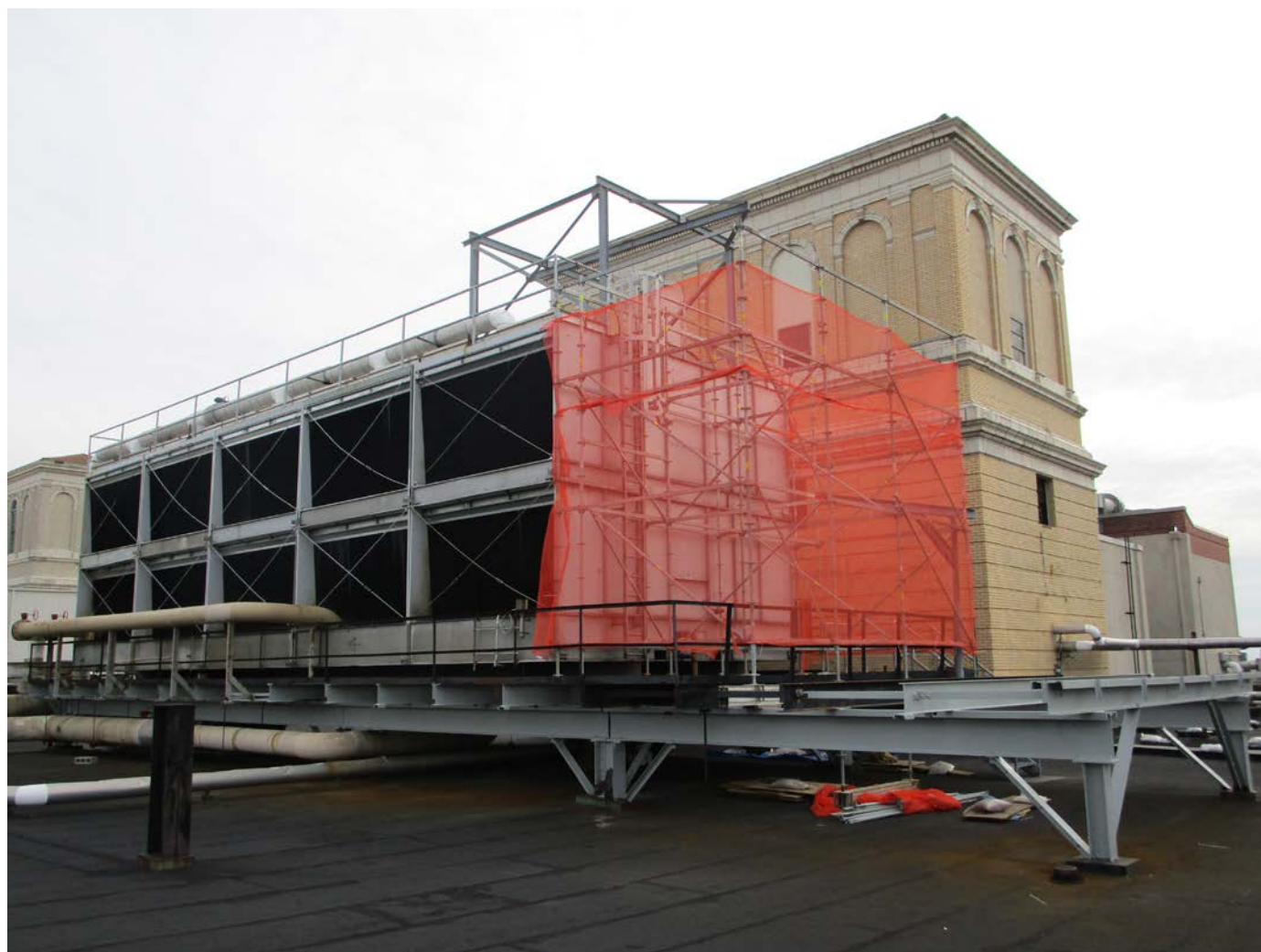
PH-12 COOLING TOWER MOCK UP
