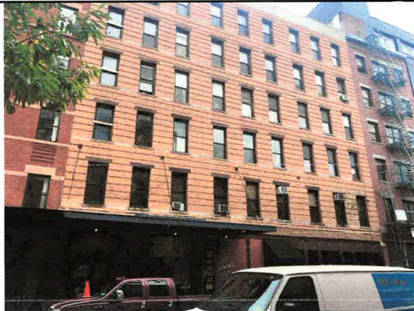
OVERALL BUILDING PHOTO
