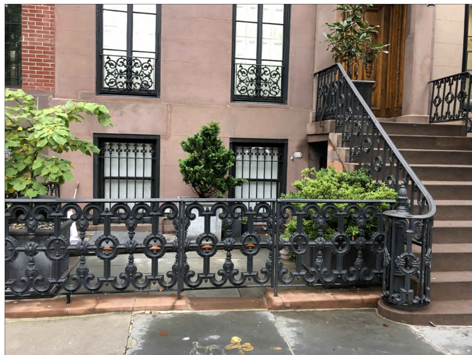
AREAWAY RAILING @ 15 LEROY STREET
