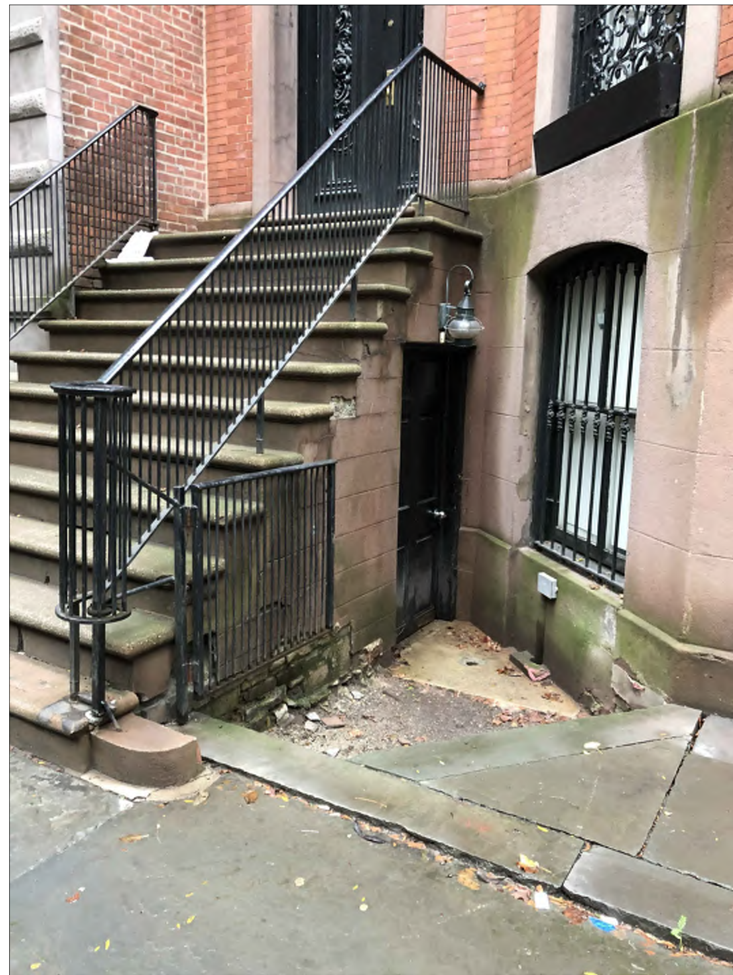
EXISTING STOOP & BASEMENT ENTRANCE DOOR @ EAST SIDE OF AREAWAY
