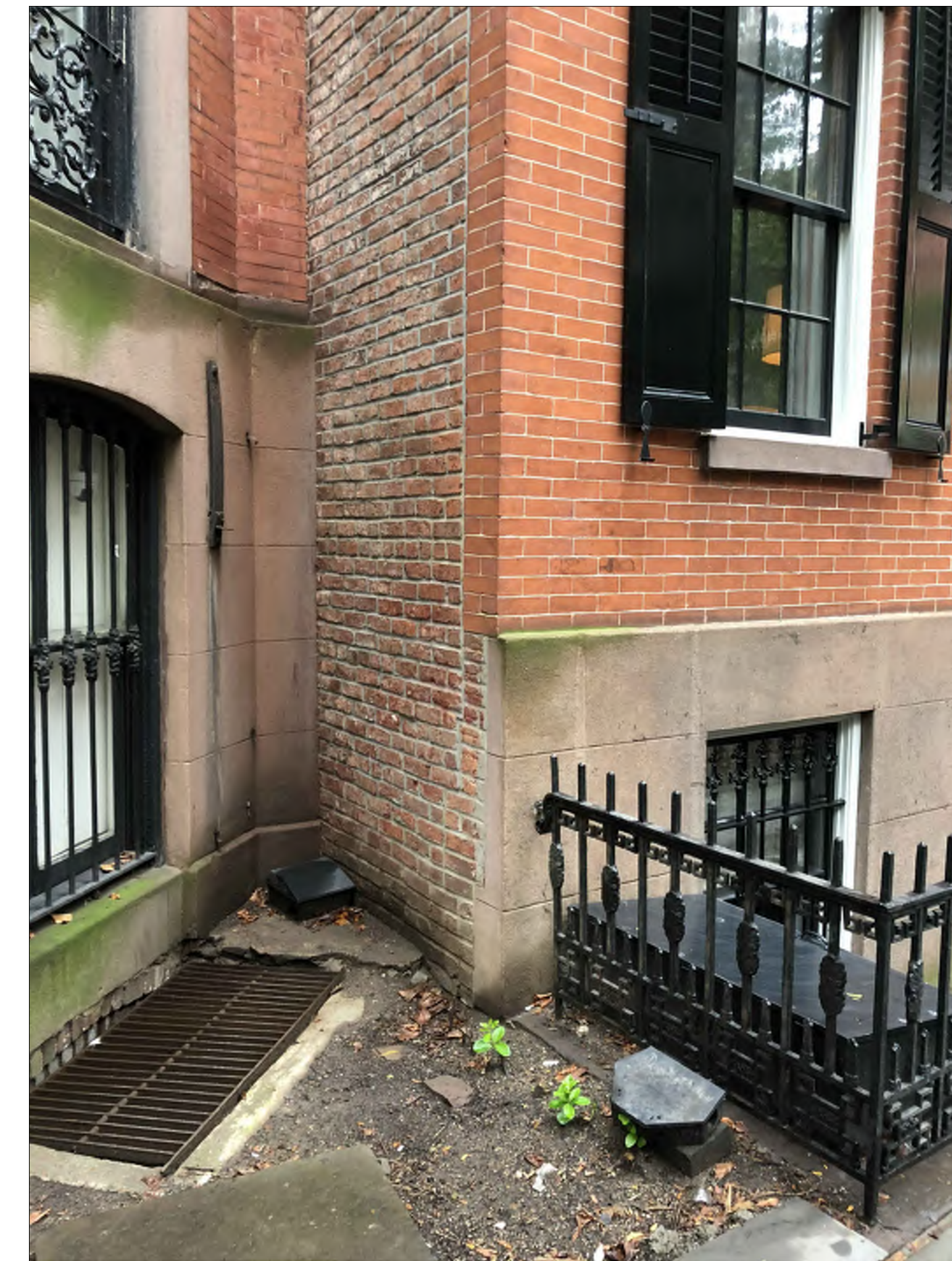
WEST SIDE OF AREAWAY ABUTTING 68 MORTON STREET
