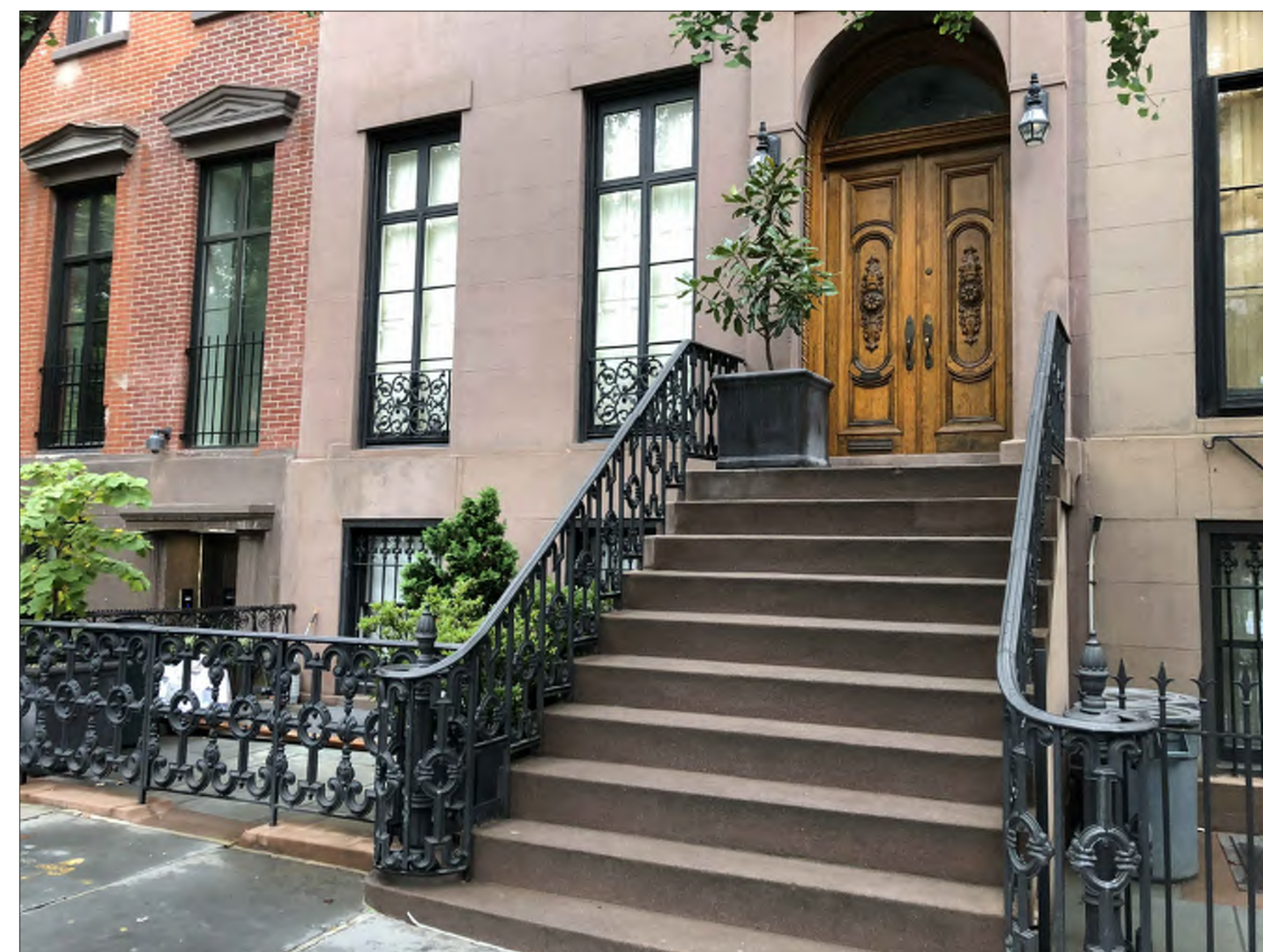
STOOP AND AREAWAY IRON WORK @ 15 LEROY STREET
