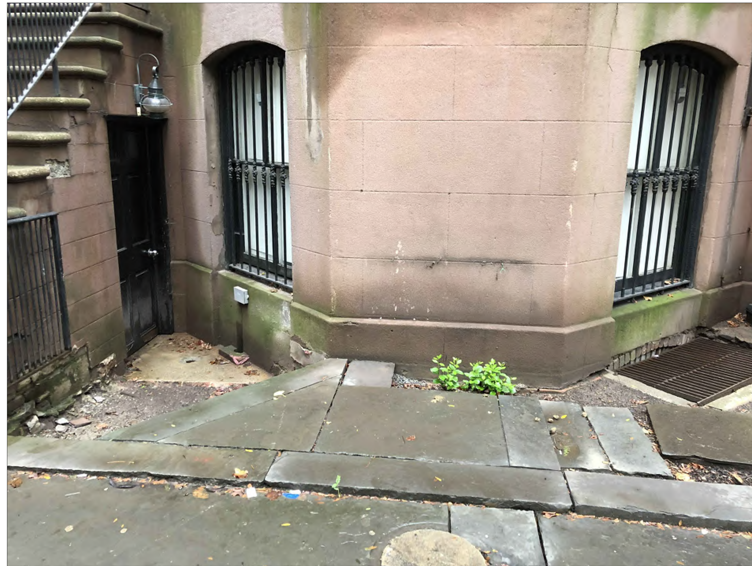
EXISTING AREAWAY @ 66 MORTON STREET
